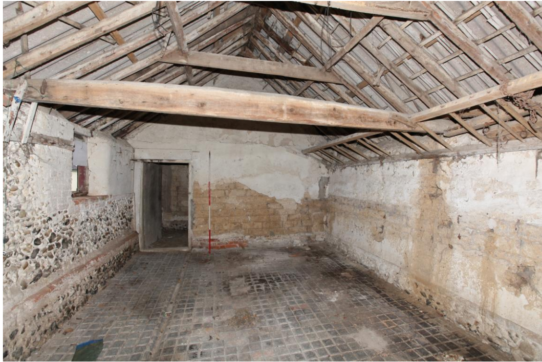
Illus. 7. The interior from the north-west of the single-storied clay-lump stable (2b) showing the largely intact 19 th century hay rack to the right and the entrance to the southernmost of the two tack rooms (2a) to the left. The scar of the missing manger is visible beneath the rack.
