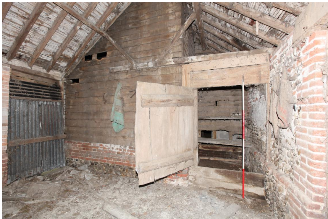
Illus. 4. The weatherboarded north-western corner of the barn (1b) within the 19 th century enclosed shed (3a). An unusual lean-to storage cupboard lies in the angle of the flint-rubble shed and the earlier porch (1c) to the right. The door to the left opens onto the horse yard.
