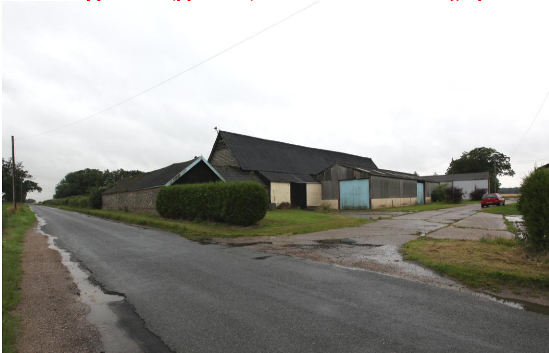
Illus. 1. A general view of the site from the public road to the north showing the farm entrance to the right. The flint-rubble shelter-shed (3) adjoins the road to the left with the partly original lean-to porch (1c) and the 20 th century store (4) adjoining the main barn (1) to the right.
