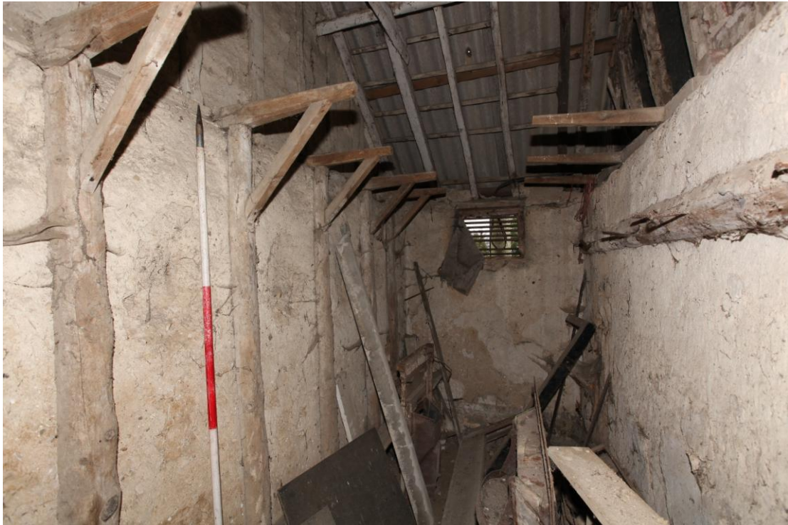
Illus. 9. The northern tack room (2c) from the north-east showing its original wooden harness hooks to both left and right.
