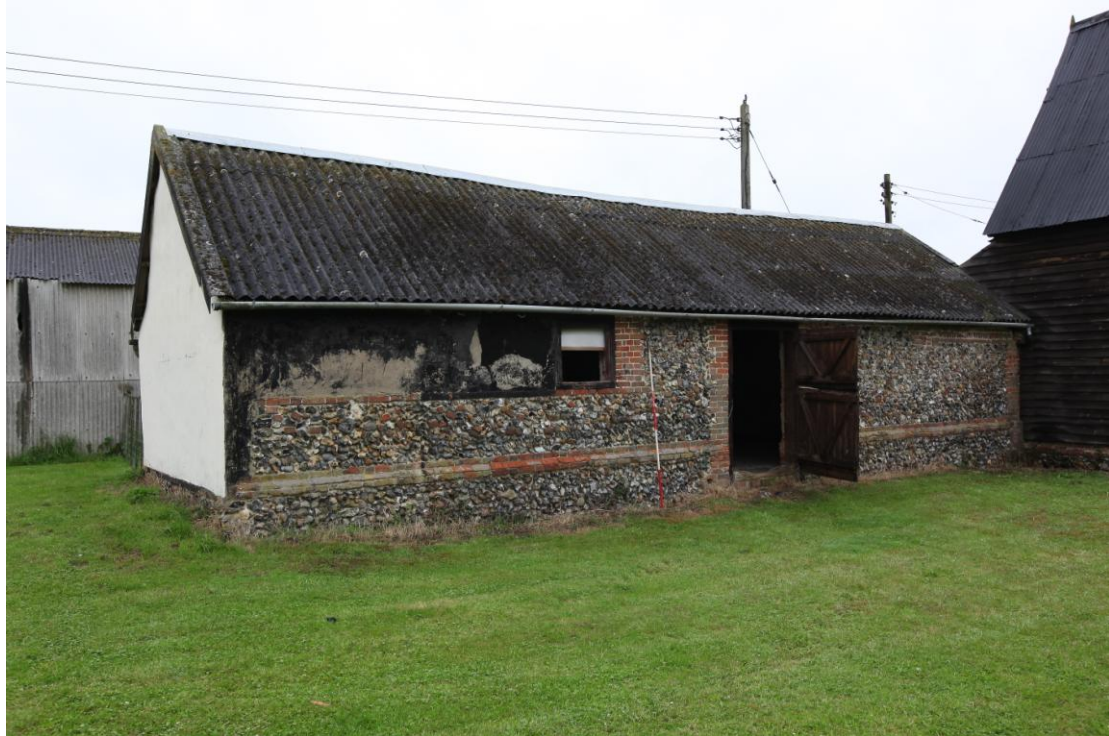
Illus. 3. The flint-rubble north-eastern facade of the clay-lump stable (2a-2c) from the east showing its original entrance with the scar of a demolished adjoining shed to the left. The upper part of the wall to the left of the window appears always to have consisted of clay-lump. The junction with the barn (1a) is visible to the right.
