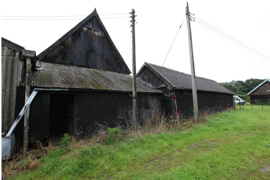
Illus. 2. The south-western gable of the barn showing the adjoining 19 th century clay-lump lean-to shed (2d) with the clay-lump stable (2a-2c) to the right and the 20 th century store (4) to the left. The building in the rear to the right is an open-sided cart lodge behind the house known as 'Greystones'.
