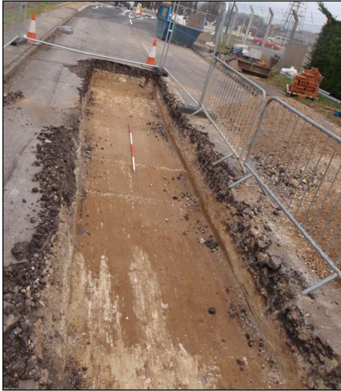
Plate 1. Trench 1 facing east, individual scale bars at 0.5m
