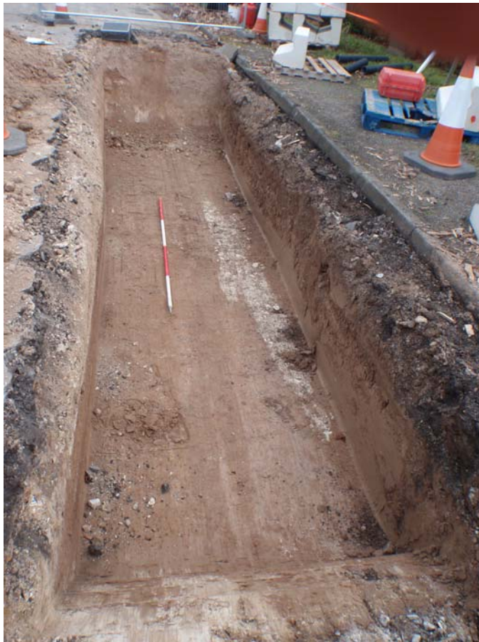
Plate 4. Trench 4 facing east, individual scale bars at 0.5m
