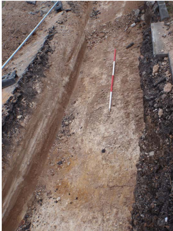
Plate 2. Trench 2 facing east, individual scale bars at 0.5m
