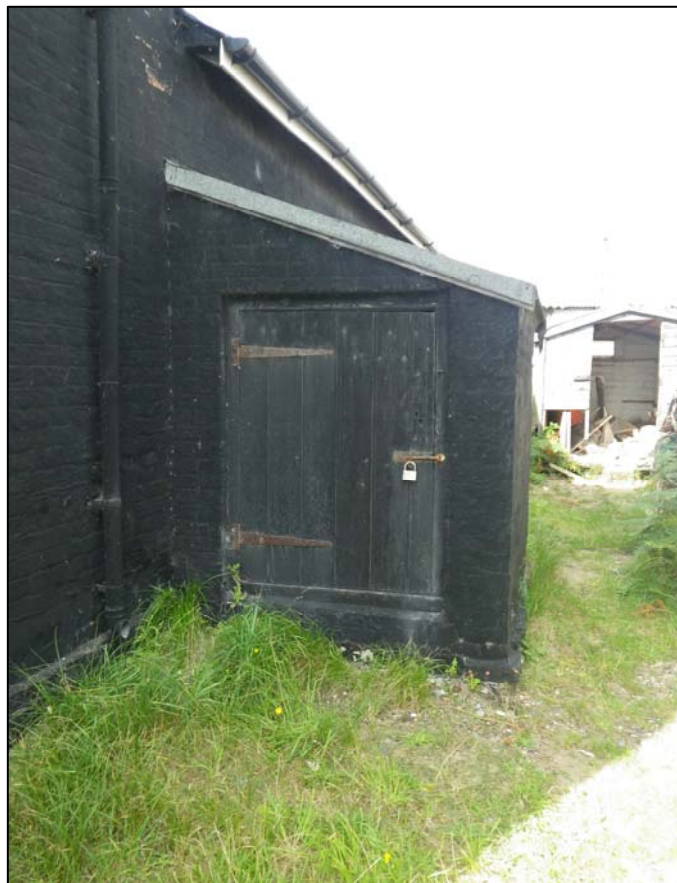
Plate 12. fuel store on northern side of the main structure (ref. HQC 59)
