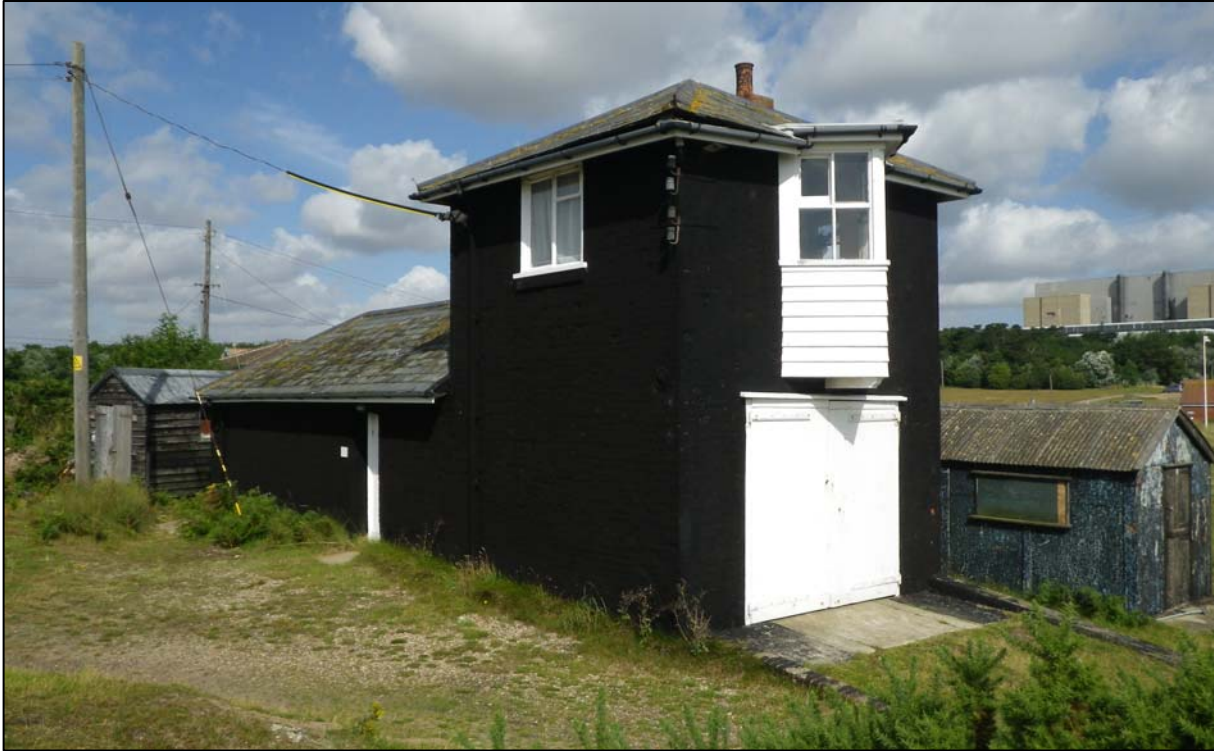
Plate 1. general view, camera facing north-west (ref. HQC 50)
