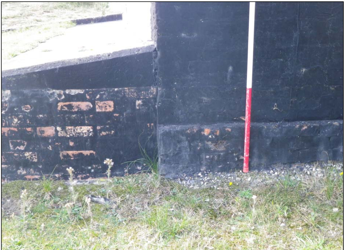
Plate 6. stepped brickwork at the base of the northern wall (ref. HQC 63)
