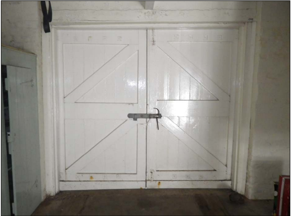
Plate 11. double doors in eastern façade, interior view (ref. HQC 91)
