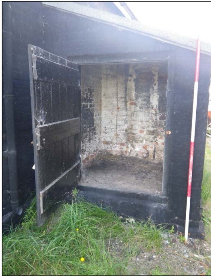
Plate 13. fuel store on northern side of the main structure (ref. HQD 79)
