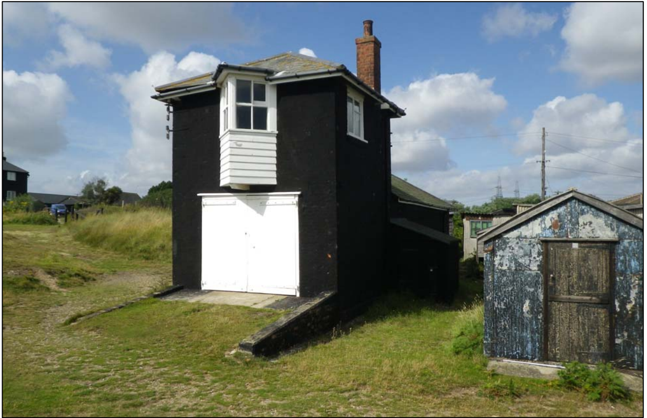
Plate 3. general view, camera facing south-west (ref. HQC 46)
