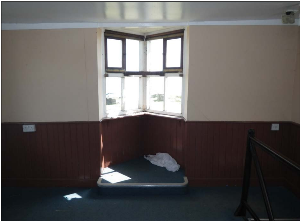
Plate 26. first floor bay window, camera facing east (ref. HQD 20)
