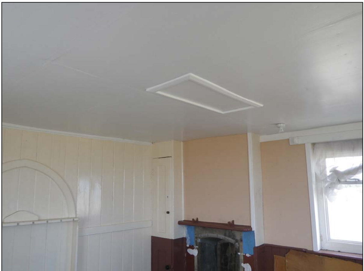
Plate 28. ceiling, first floor, camera facing north-west (ref. HQD 55)
