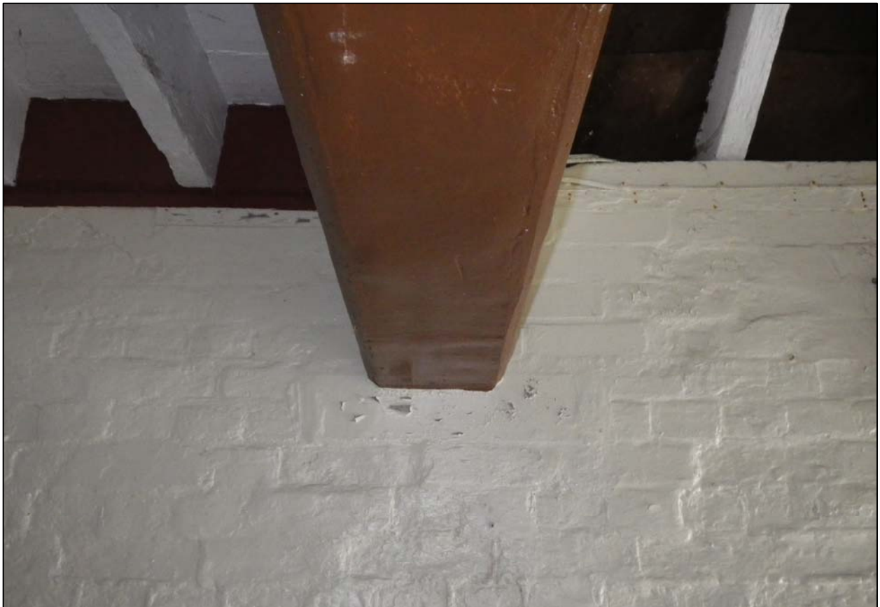
Plate 16. beam supporting the west wall of the upper storey (ref. HQD 05)
