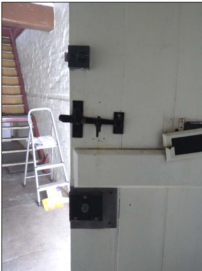
Plate 8. doorway in the southern façade, interior, locks and latches (ref. HQD 77)
