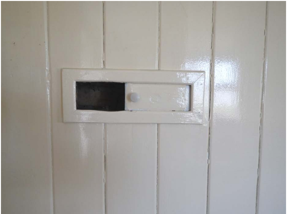
Plate 34. sliding timber panel, possible vent or peep-hole (ref. HQD 30)
