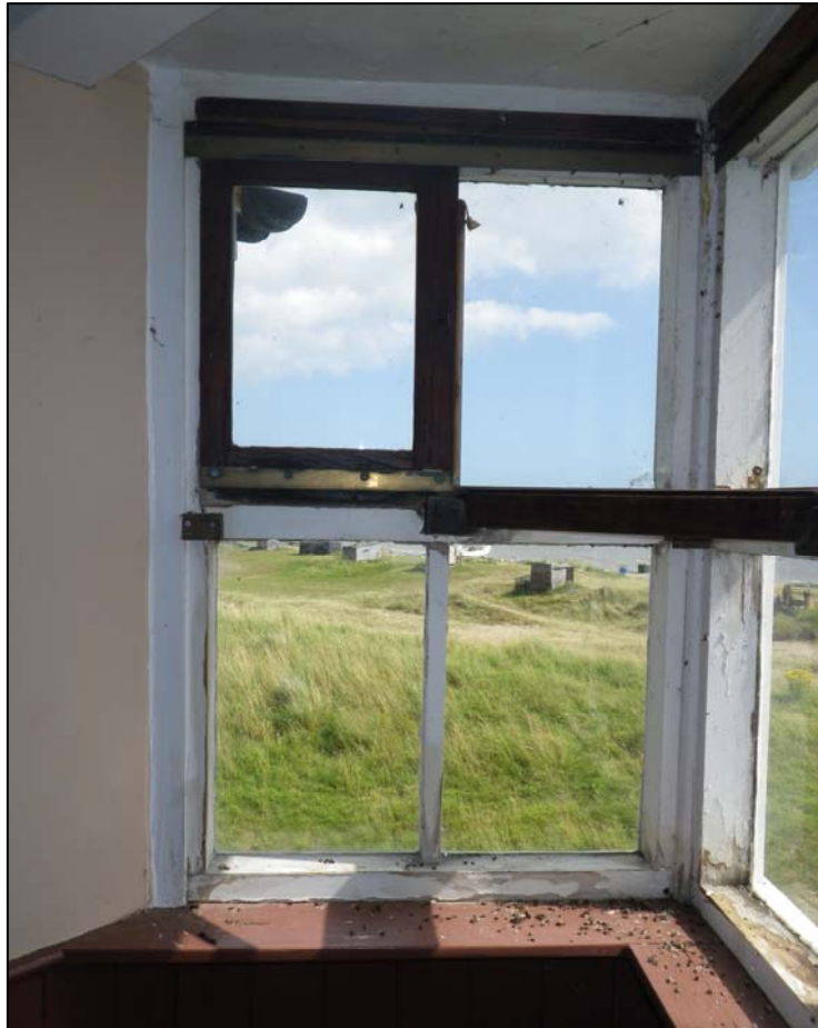
Plate 29. bay window, sliding frame, camera facing north-east (ref. HQD 47)
