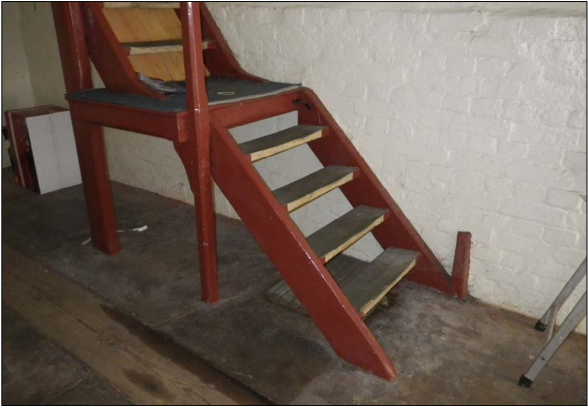
Plate 23. stairs to first floor, removable section (ref. HQC 89)
