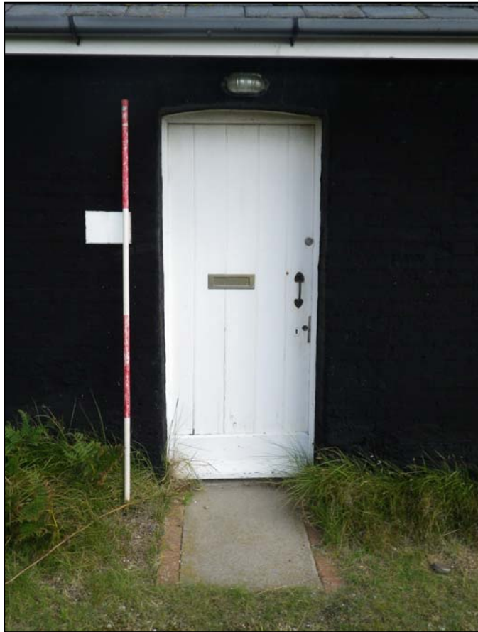
Plate 7. doorway in the southern façade (ref. HQC 56)
