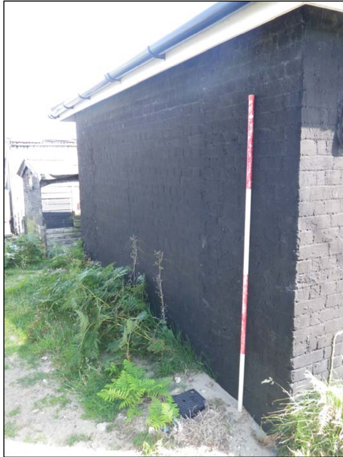
Plate 5. infilled doorway in the western façade (ref. HQC 58)
