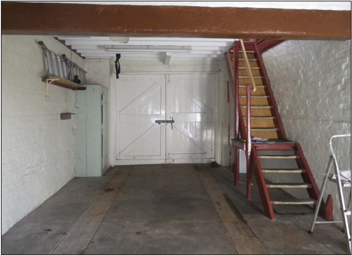
Plate 17. general view of the interior of the building, camera facing east (ref. HQC 85)
