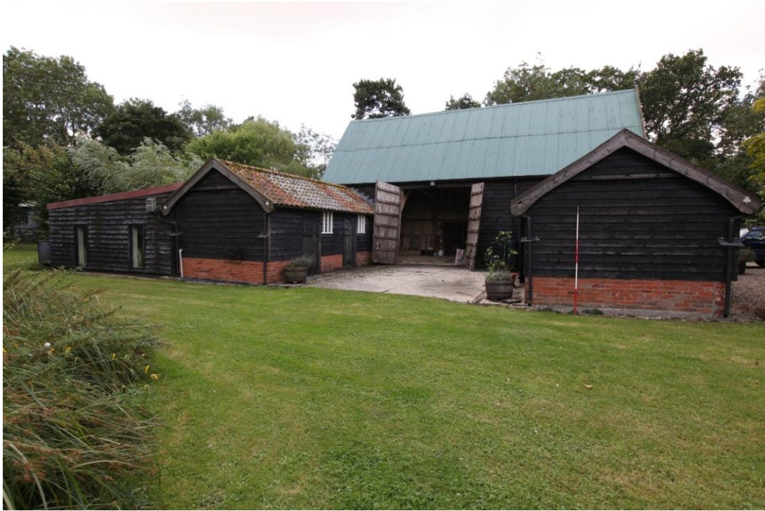
Illus. 3. The barn complex from the east showing the timber-framed threshing barn (1) with its corrugated iron roof in the rear and the 19th century yard sheds (3 & 4) to left and right. The 20 th century lean-to to the extreme left (4) houses a swimming pool and the adjoining yard shed has been converted into boiler and wet rooms.
