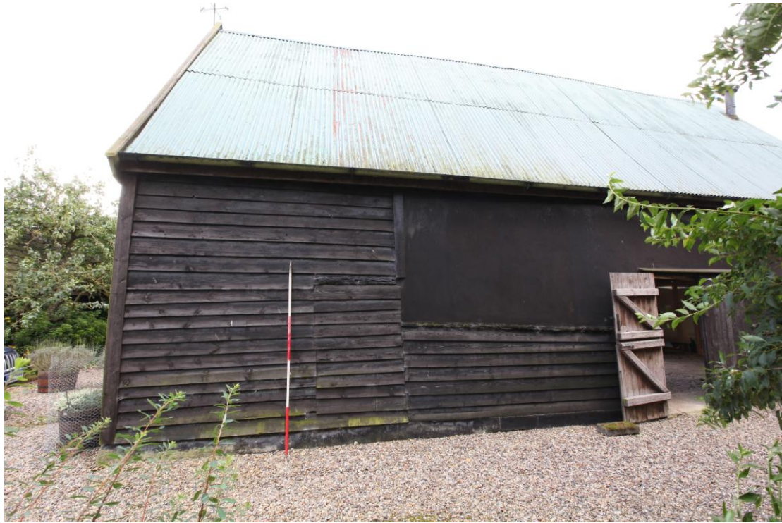
Illus. 5. The western exterior of the barn's northern showing the outline of a blocked secondary door in the position of the original ground-floor window in bay C (the window lintel forming the door lintel to the right of the scale rod). The two-tier cladding of cement-rendered clay daub above weatherboarding reflects the barn's appearance in the 18 th and 19 th centuries, although the daub probably extended to the ground initially.
