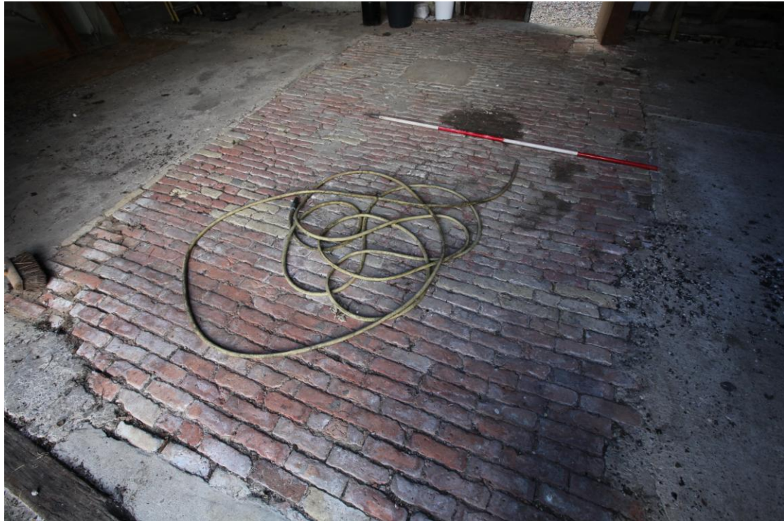
Illus. 7. The well preserved 19th century threshing floor of mixed red and gault brick in bay B of the barn (1), seen from its eastern entrance. The floor is of modern concrete elsewhere.
