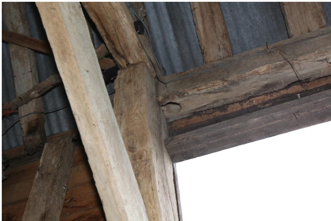
Illus. 14. A detail of the eastern roof-plate of bay B showing the circular pin-hinge housing of the original entrance door. The present doors are modern replacements.
