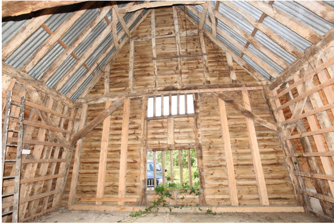
Illus. 13. The interior of the northern gable. The vertical studs were replaced as part of a late-20 th century restoration, and the left-hand brace is also secondary, but the right-hand brace and window jambs are original with pegged trenches for a missing mid-rail. A pegged mortise in the left-hand corner post and a corresponding gap in the studwork reveal the position of an original external door. The diamond mullion windows are modern and it is unclear whether they recreate original features or are entirely secondary.
