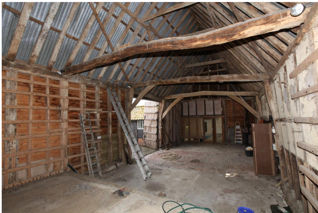
Illus. 6. The interior of the barn (1) from the north, showing the original tie-beam without braces between bays C and D in the foreground and three of the original four arch-braces flanking the threshing floor in bay B to the rear. The braces were omitted to maximise headroom on the (removed) loft in the two northern bays.
