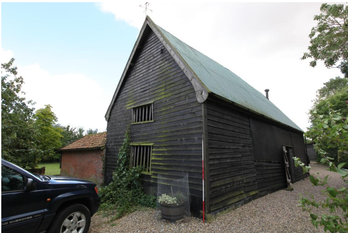
Illus. 4. The exterior of the barn (1) from the north-west showing the late-20th century diamond-mullion windows in its gable. There is internal evidence of an original gable door to the left of the scale rod.
