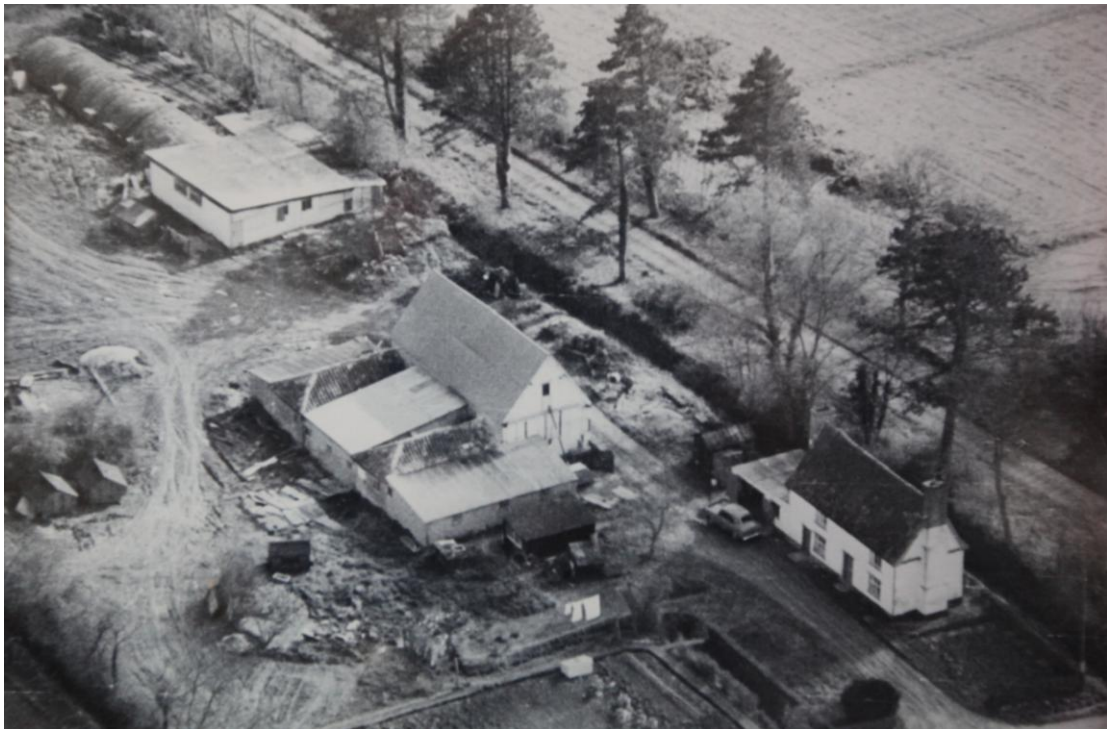
Illus. 1. An Aerial photograph of 1964 taken from the north-east and showing the close proximity of the grade II-listed farmhouse (5, right) and the grade II-listed barn (1, centre). The yard adjoining the barn's eastern elevation is walled and roofed as a lean-to, with a separate lean-to against the northern yard shed (4) – both since demolished. The house has two doors and appears to form a pair of cottages.
