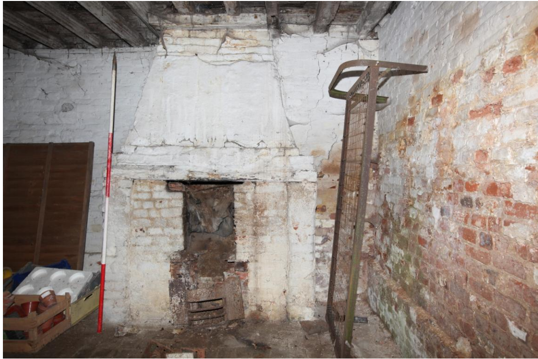
Illus. 7. The original fireplace in the south-western internal gable of the early-19th century shed (2). This was reduced in width to install a cast-iron coal grate with floral decoration in the late-19 th century but is otherwise identical to the fireplace on the other side of the chimney (illus. 4) – although its lintel is 0.5 m higher due to the sunken floor.
