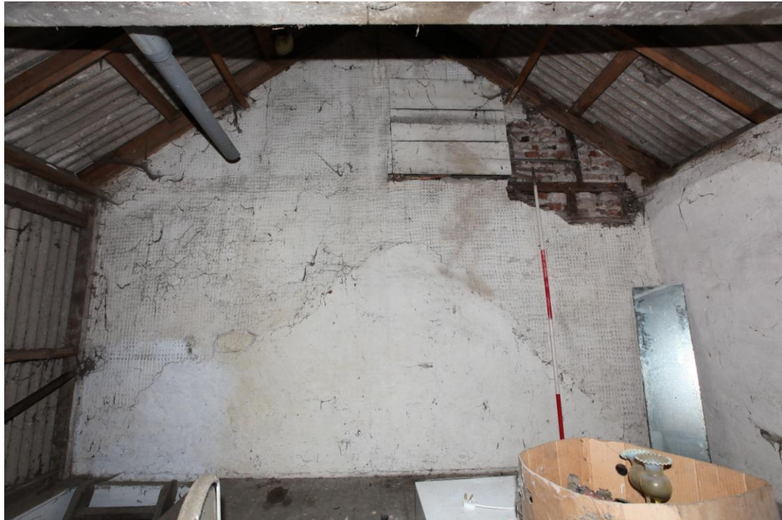
Illus. 15. The interior of the late-19 th century shed (3) from the north-east, showing the original whitewashed external pargeting of the early-19 th century shed (2) with the roof outline of an earlier, lower building on the same site. The roof and most of the south-eastern facade (left) of the late-19 th century shed was rebuilt in softwood and corrugated asbestos in the mid-20 th century
