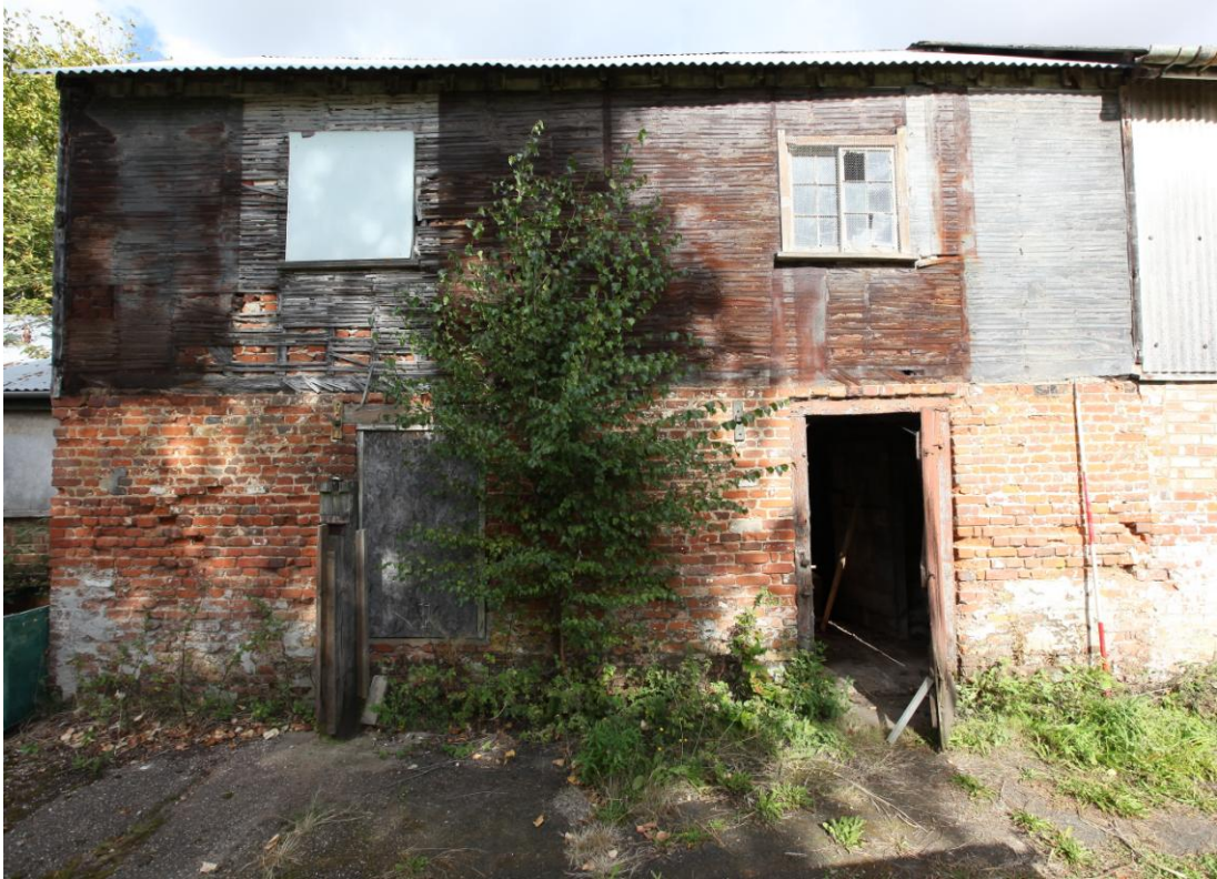
Illus. 5. The south-eastern facade of the early-19th century shed (2) showing its original door and horizontal sash window to the right with boarded sash windows to the left. The plaster of the timber-framed upper storey has been removed and the exposed battens are now covered only by expanded metal lath. The original peg tiles were replaced by corrugated metal after Mr Eaves' death in the 1990s.
