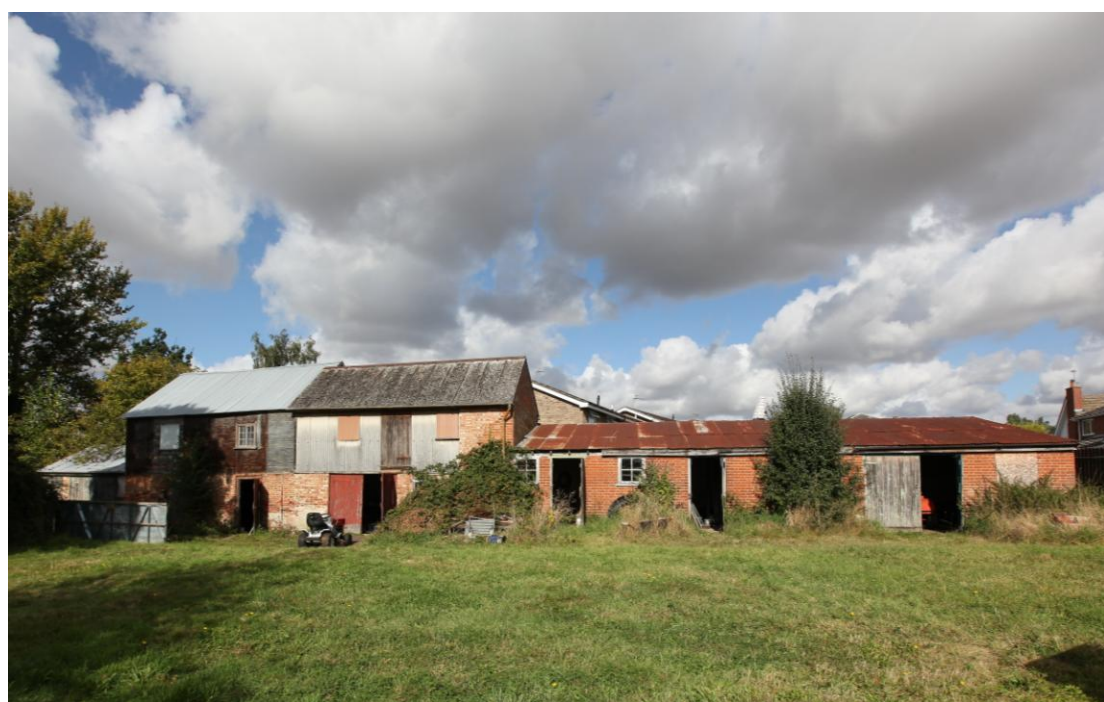
Illus. 2. The buildings from the former orchard to the south-east showing from left to right the single-storied 20 th century vehicle shed (1), the early-19 th century shed (2), the late-19 th century shed (3) and the long, single-storied brick shed with a mono-pitch roof and separate entrances to its three compartments (4a-c).
