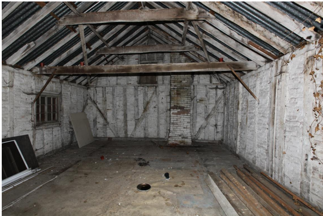
Illus. 12. The interior from the north-east of the loft in the early-19th century shed (2) showing one of the two probably original horizontal sliding-sash window in the south-eastern facade to the left with the chimney and hatch in the south-western gable. There are no windows or doors in the entire rear north-western elevation (right). The wall studs and rafters include a high proportion of re-used medieval timber.
