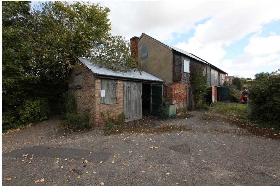
Illus. 3. The sheds from the south showing the footpath to the left of the single-story early-20 th century Fletton-brick vehicle shed (1) with the adjoining early-19 th century shed (2) on the right.
