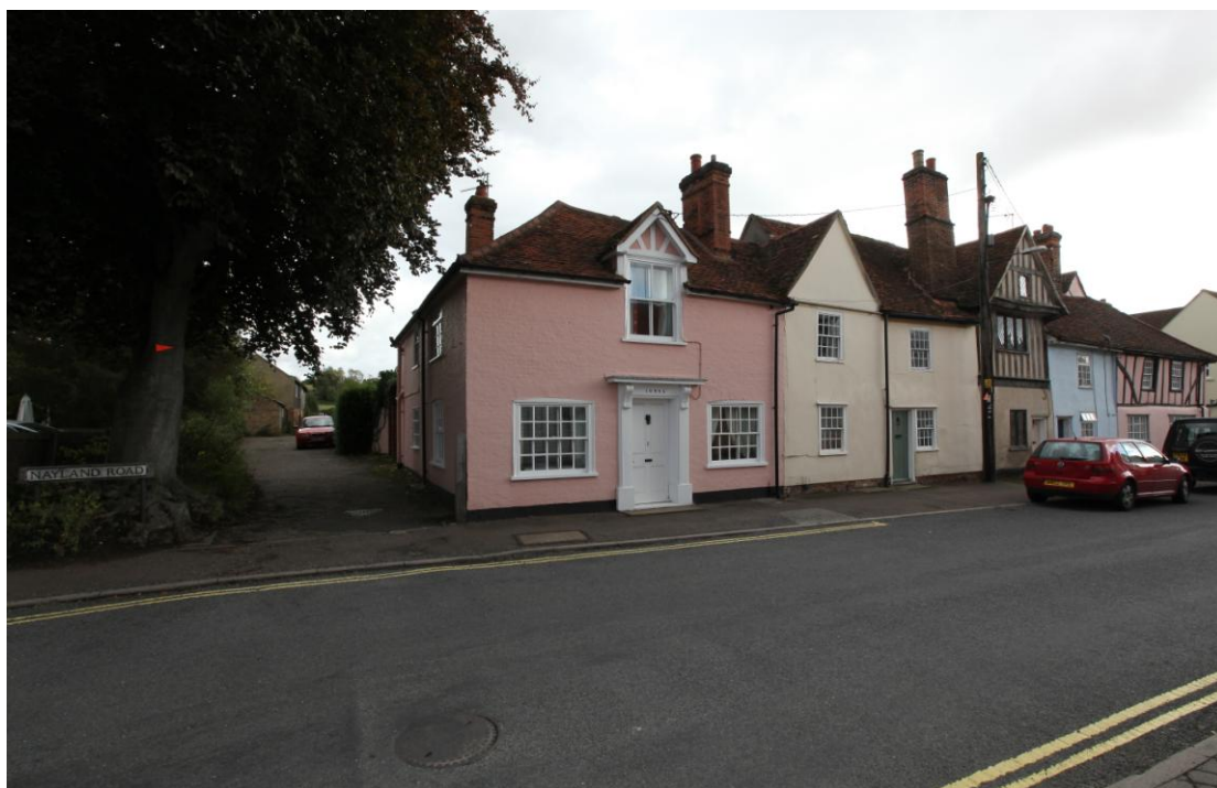
Illus. 1. The entrance to the site from Nayland Road showing the sheds in the rear to the left and the range of cottages to which they formerly belonged on the right. All are listed at grade II and appear to have formed the front range of a large Tudor inn. The tallest gable is a gatehouse that opened onto a courtyard of buildings from which the re-used timber in the early-19 th century shed (2) probably derived.
