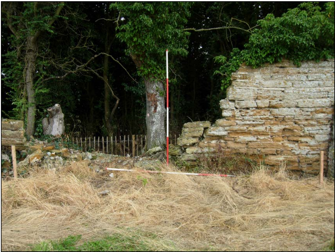
Plate 21. E. precinct wall: Stint 50 – 55m
