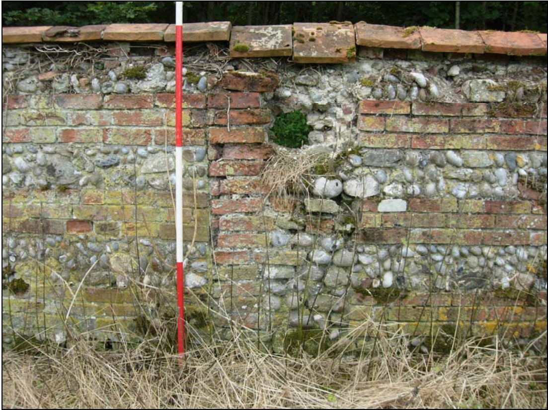
Plate 75. S. precinct wall: internal, blocked opening
