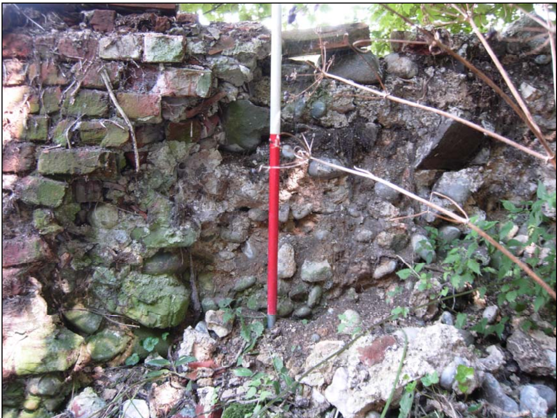
Plate 68. S. precinct wall: external, junction between fabrics
