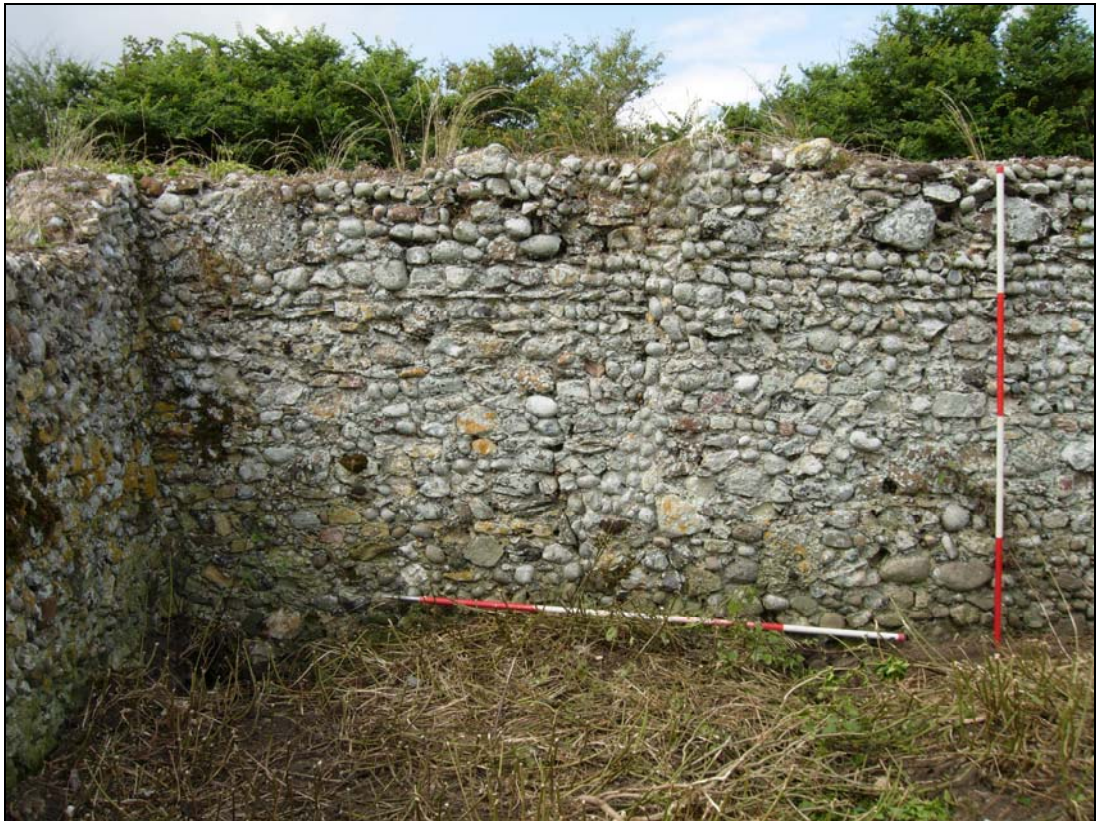
Plate 59. W. precinct wall: SW. corner wall fabric, internal
