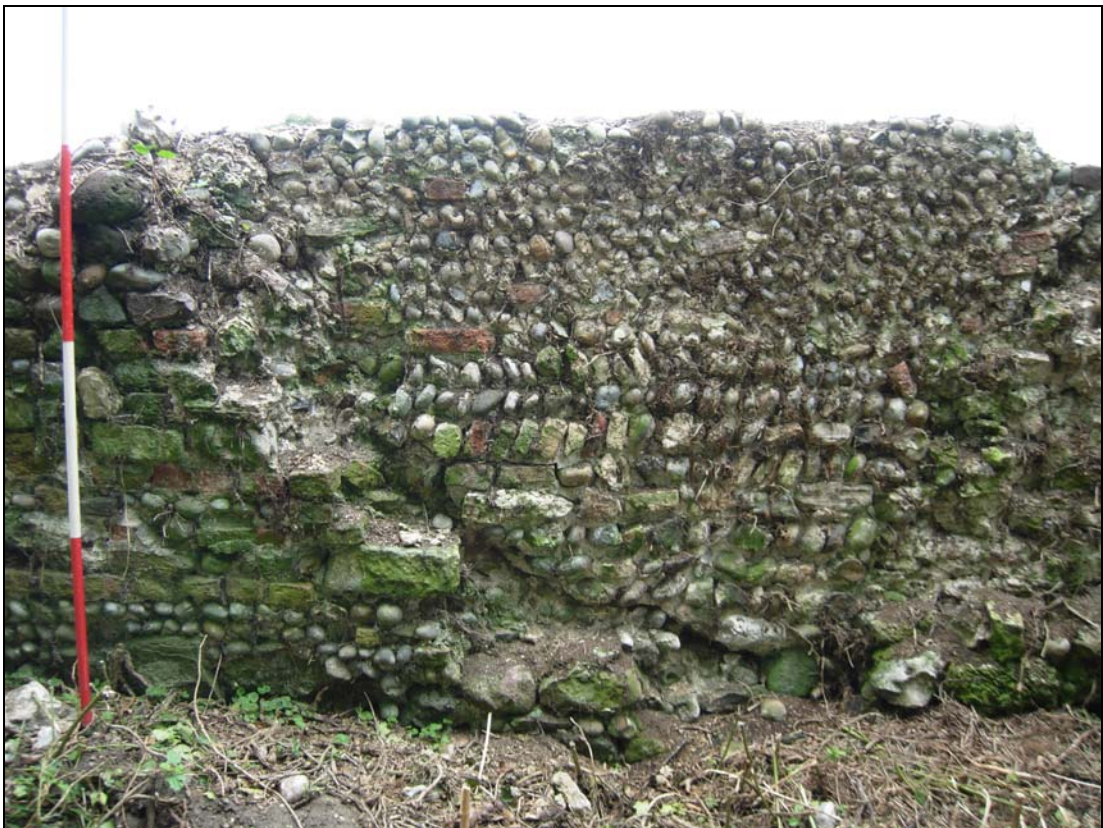
Plate 66. S. precinct wall: external, E. end repaired face
