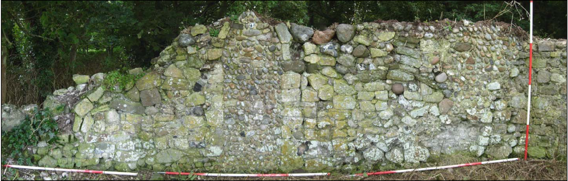
Plate 57. Precinct wall, SE corner: blocked doorway (internal)
