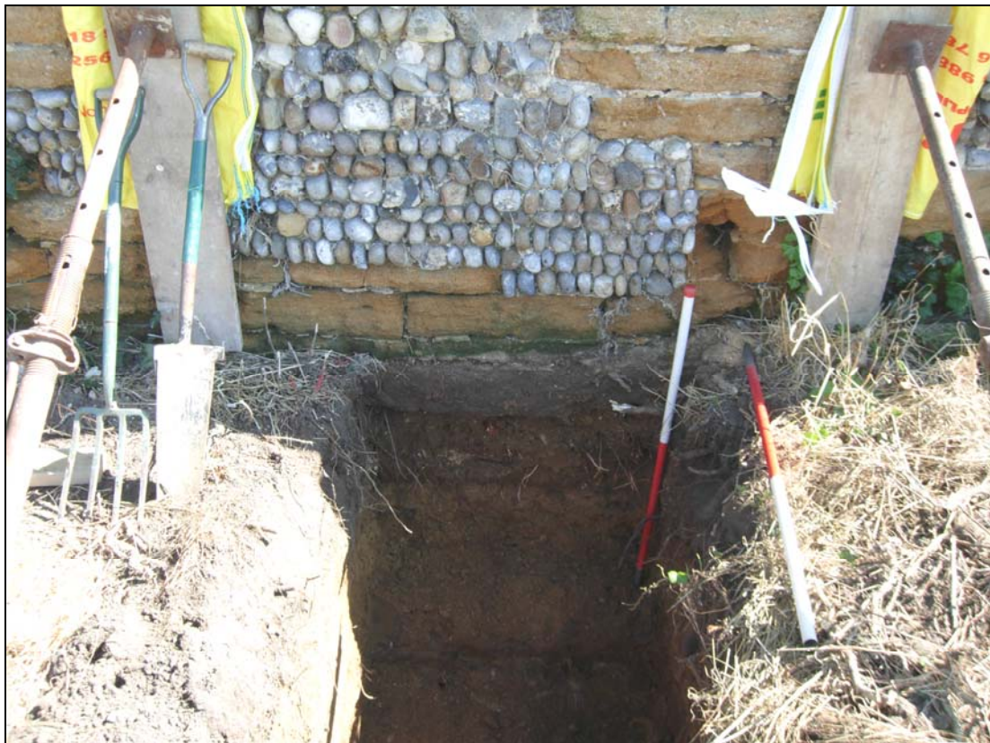
Plate 54. E. precinct wall: buttress footing 5
