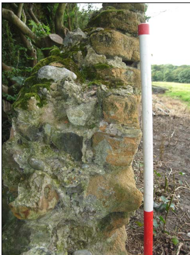
Plate 41. E. precinct wall: cross-section through wall at c.33m
