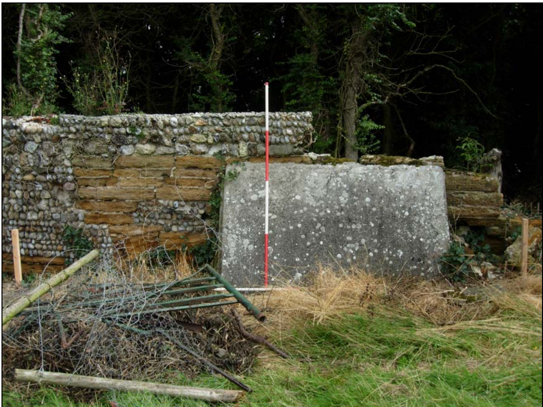
Plate 20. E. precinct wall: Stint 45 – 50m
