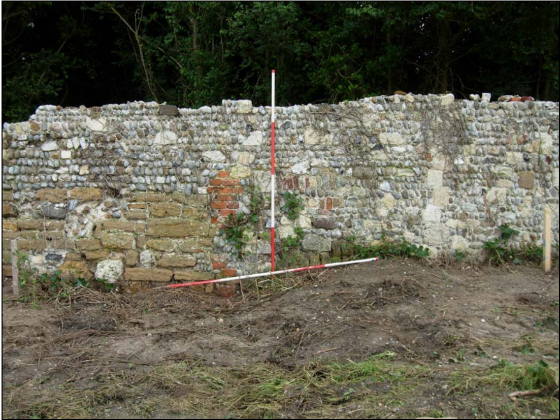
Plate 13. E. precinct wall: Stint 10 – 15m
