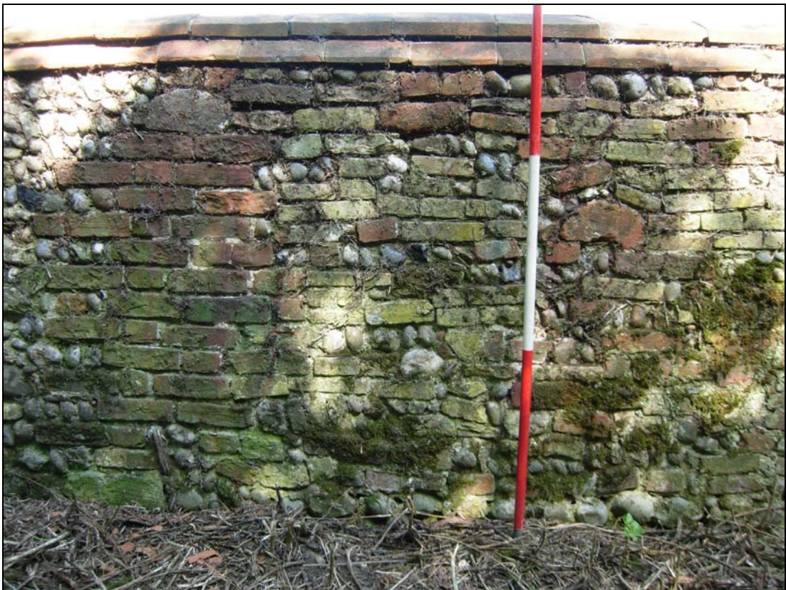
Plate 72. S. precinct wall: external, example of vertical brick element
