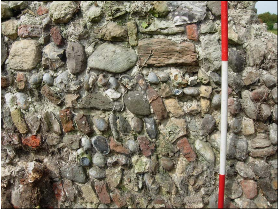
Plate 47. E. precinct wall: external, representative example of facing at c.95m
