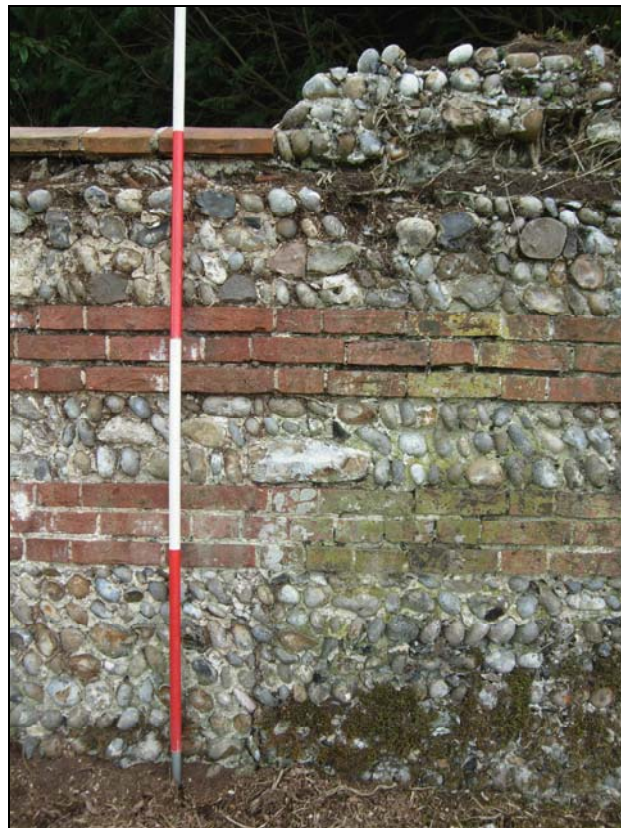
Plate 76. S. precinct wall: internal, wall fabric junction
