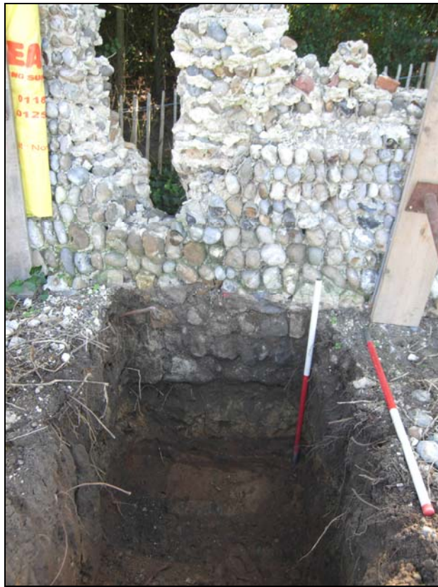
Plate 51. E. precinct wall: buttress footing 2
