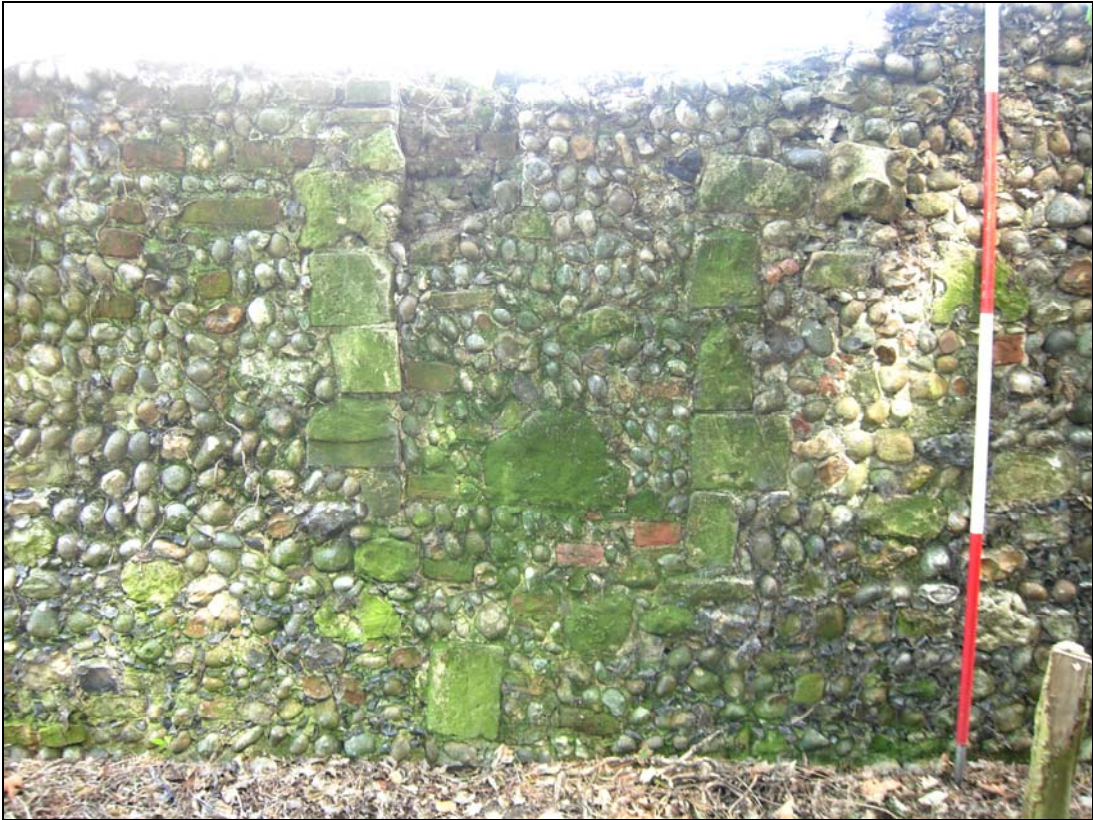
Plate 81. S. precinct wall: external, blocked opening
