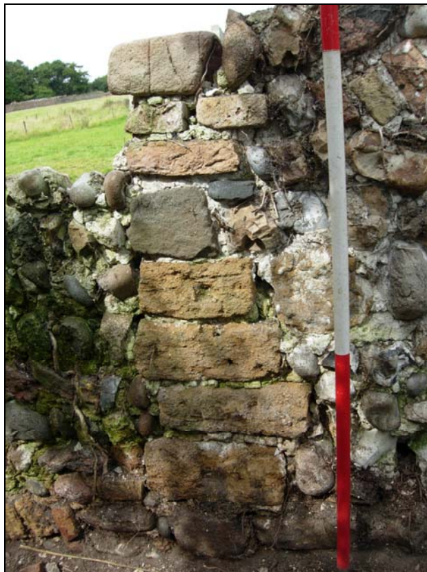
Plate 48. E. precinct wall: external, vertical element with limestone crag
