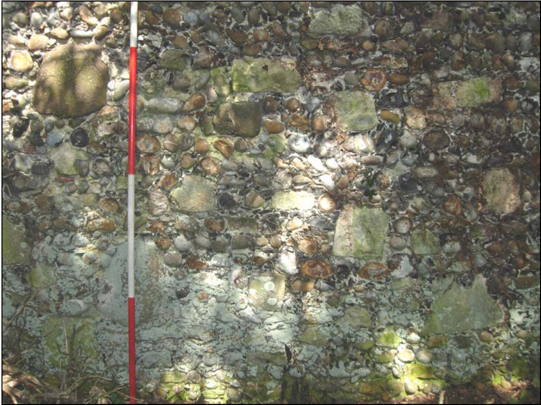
Plate 79. S. precinct wall: external, example of facing
