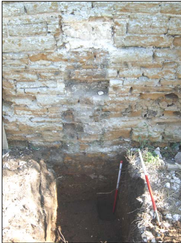
Plate 55. E. precinct wall: buttress footing 6
