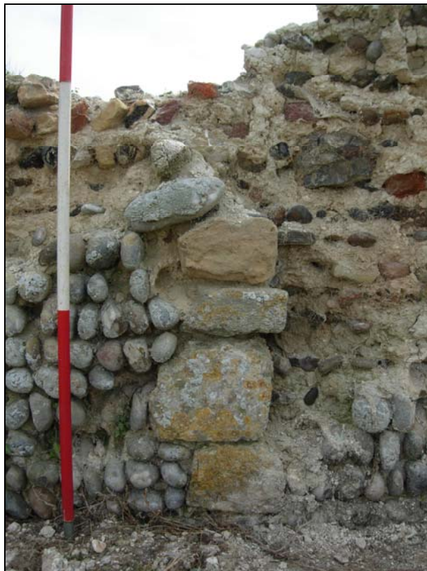
Plate 46. E. precinct wall: internal, example of vertical element
