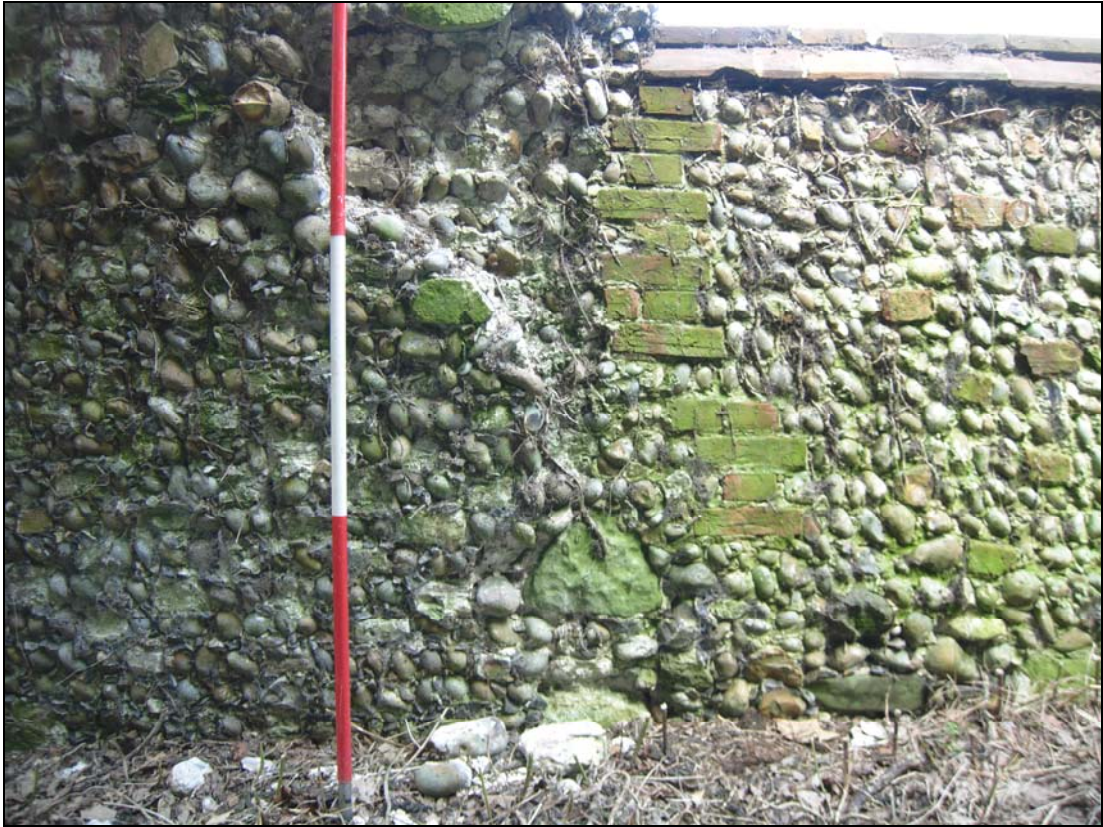
Plate 77. S. precinct wall: external, wall fabric junction
