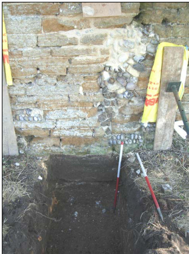
Plate 56. E. precinct wall: buttress footing 7
