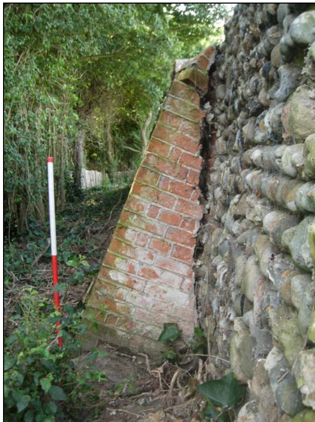
Plate 34. E. precinct wall: brick buttress from the N.
