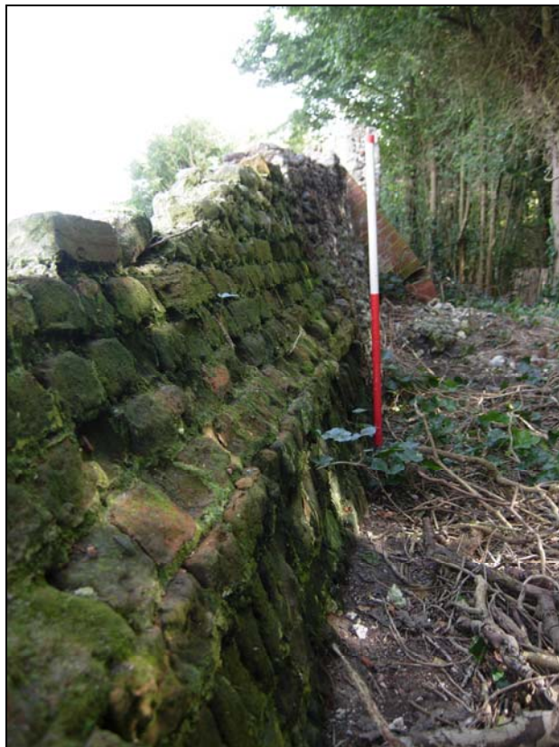
Plate 40. E. precinct wall: external brick face c.25 – 32m, taken from S.
