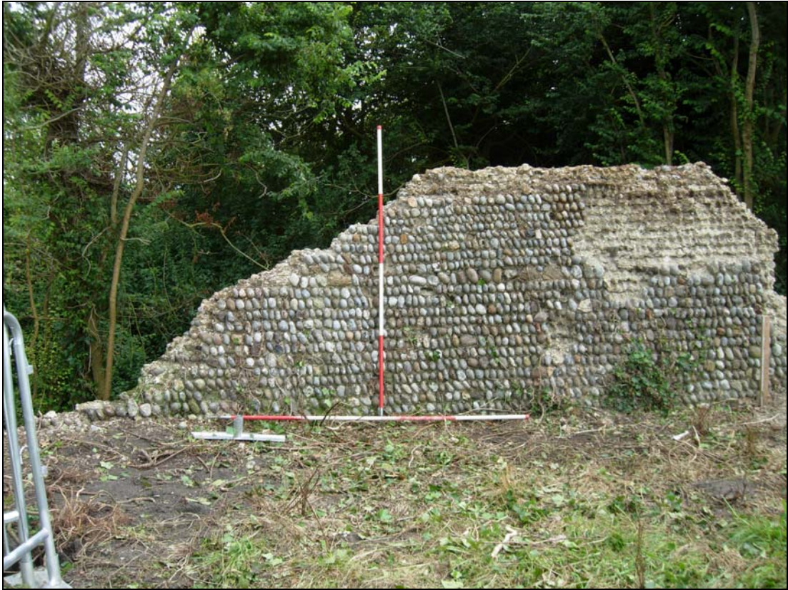
Plate 11. E. precinct wall: Stint 0 – 5m
