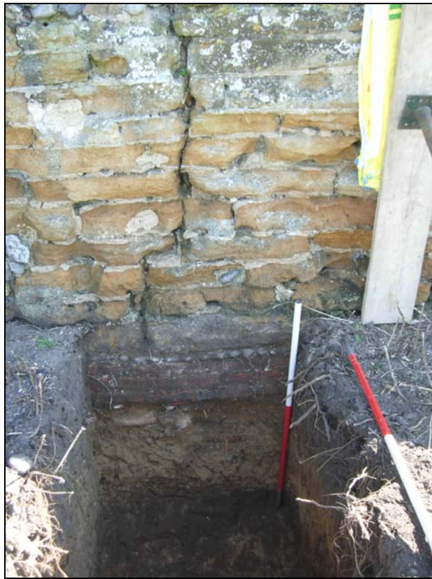
Plate 53. E. precinct wall: buttress footing 4
