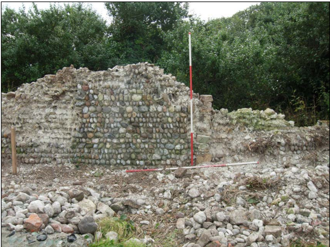
Plate 32. E. precinct wall: Stint 105 – 110m
