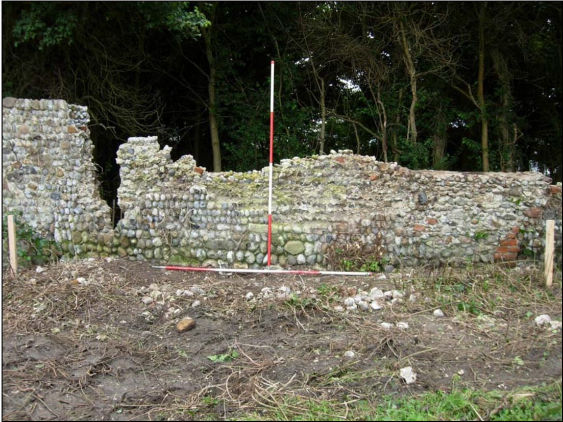
Plate 15. E. precinct wall: Stint 20 – 25m
