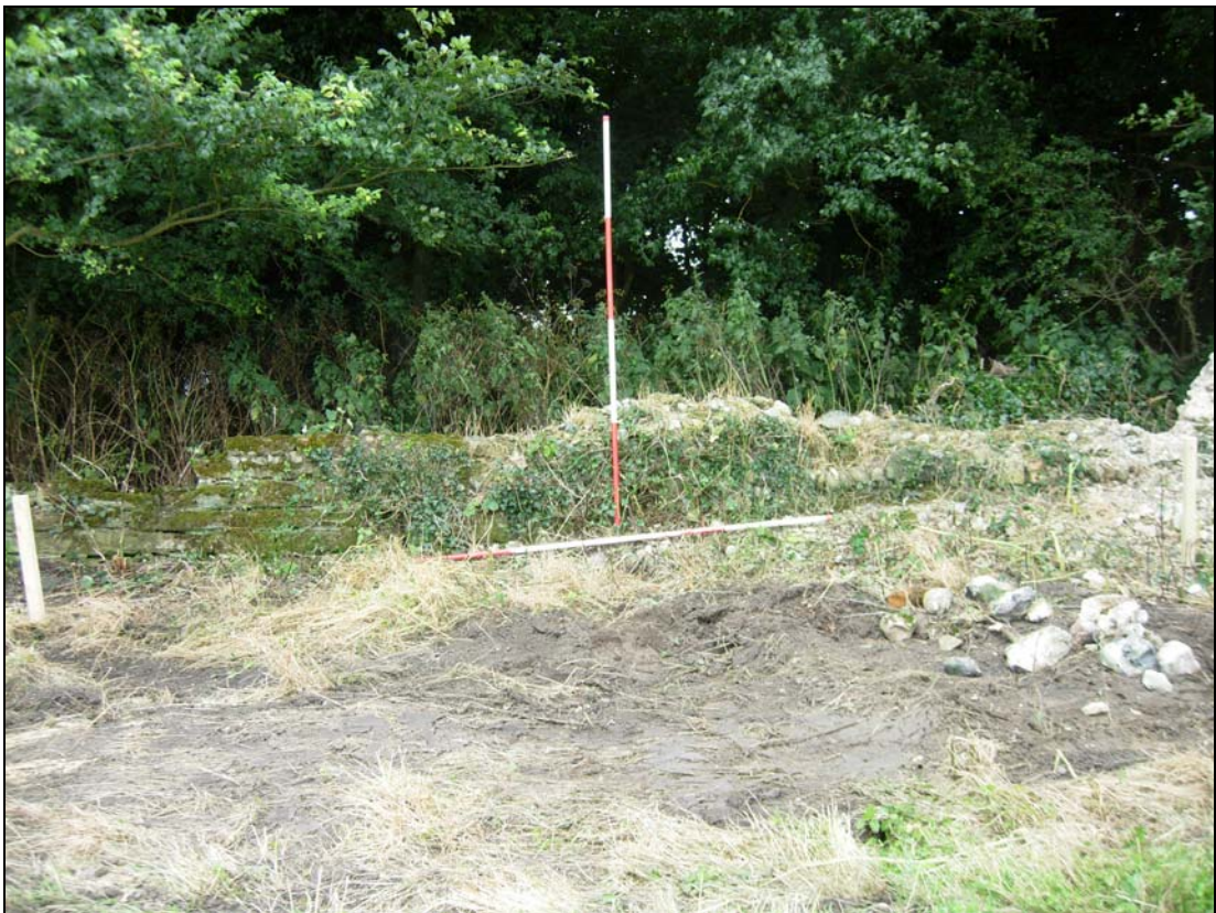
Plate 26. E. precinct wall: Stint 75 – 80m
