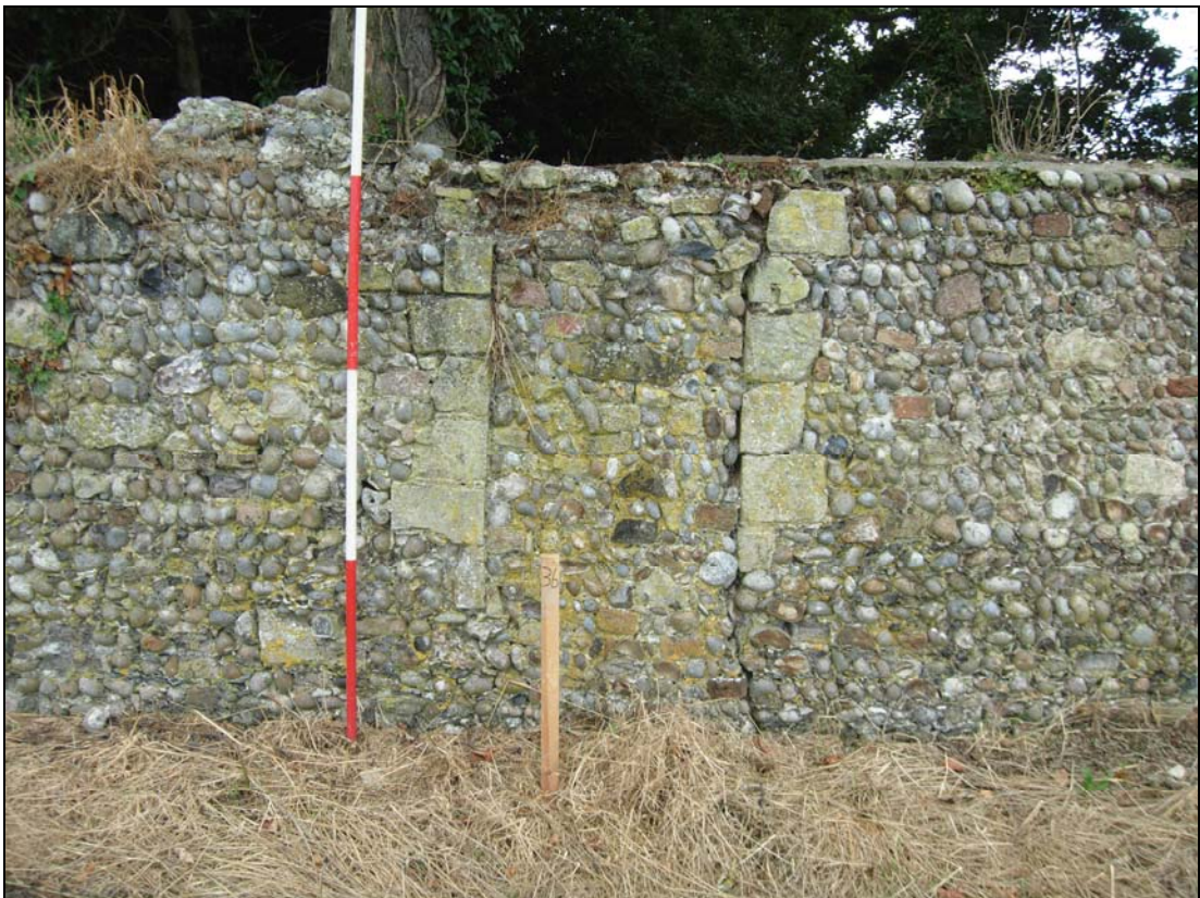
Plate 80. S. precinct wall: internal, blocked opening
