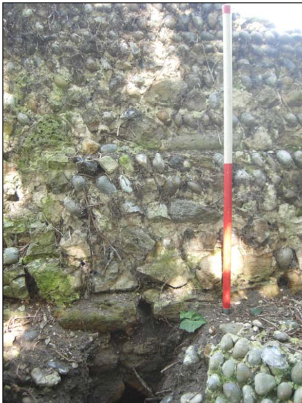
Plate 38. E. precinct wall: external face with limestone crag base
