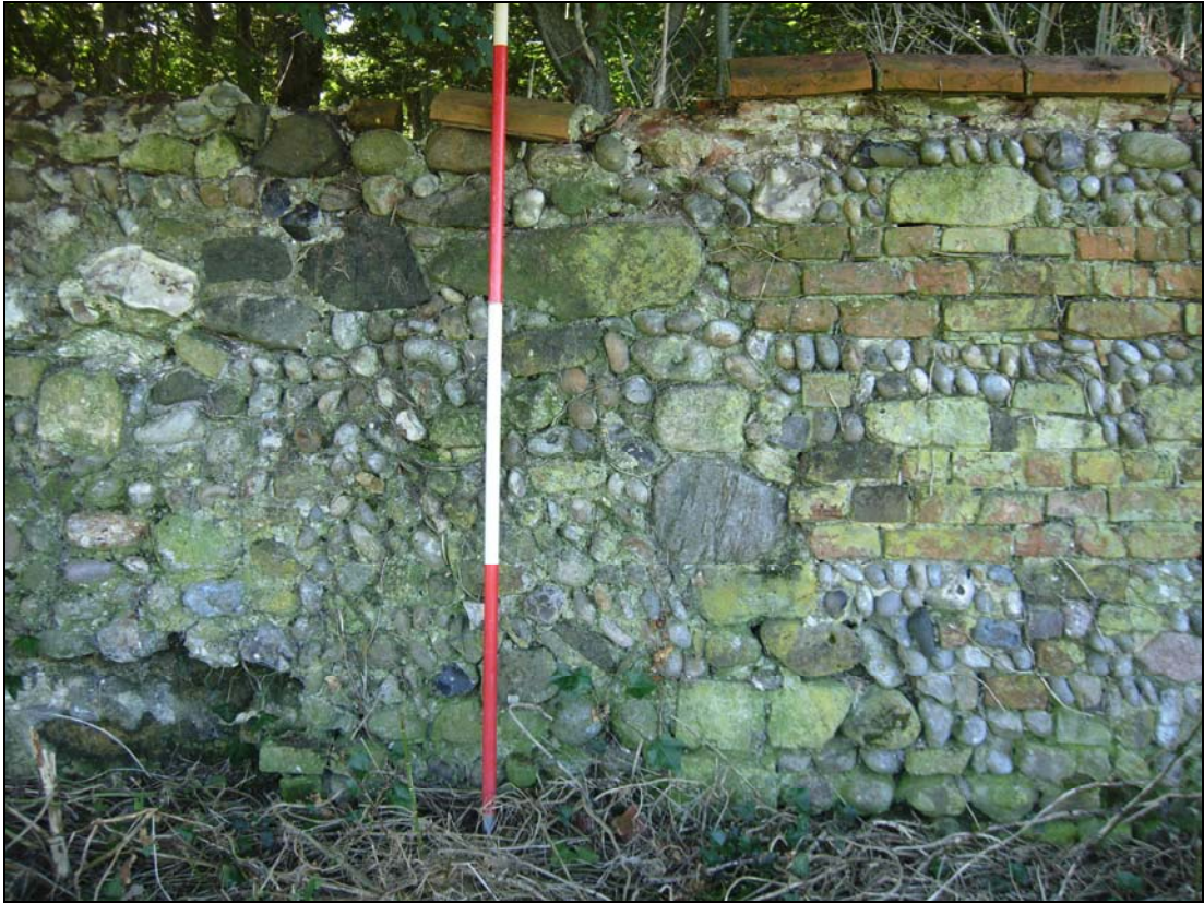
Plate 67. S. precinct wall: internal, junction between fabrics
