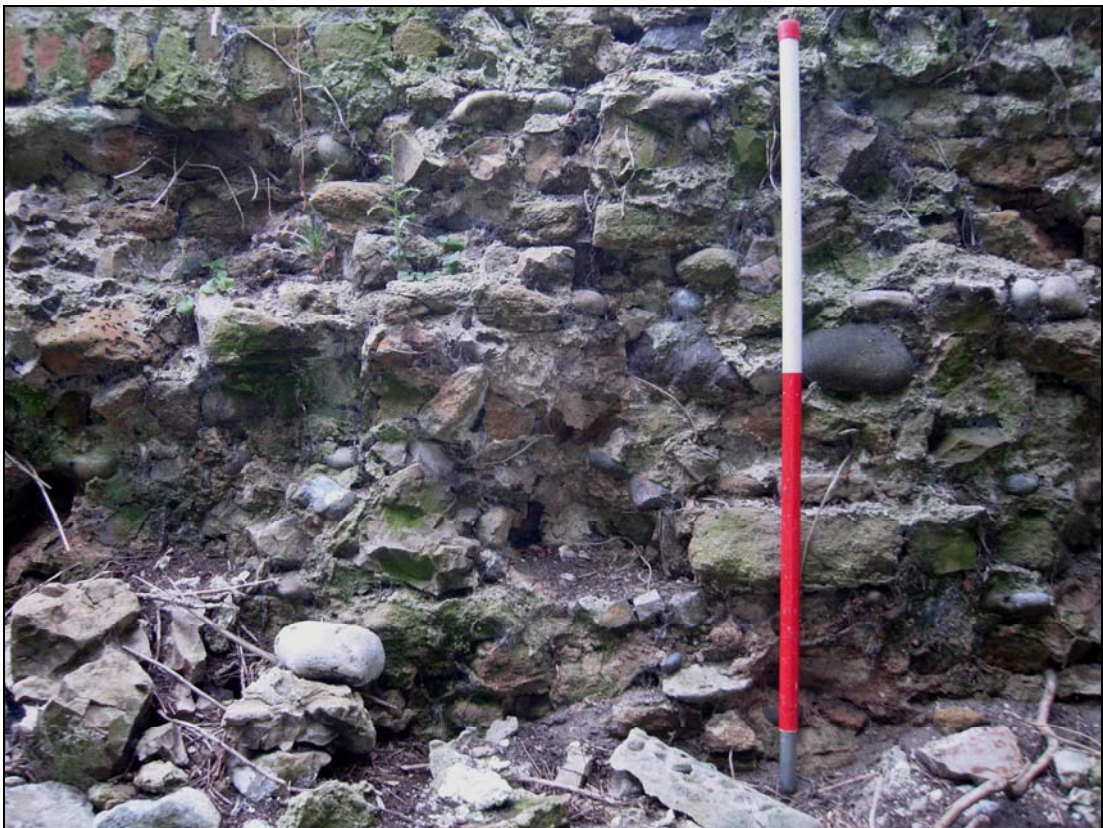
Plate 44. E. precinct wall: external, example of original medieval corework
