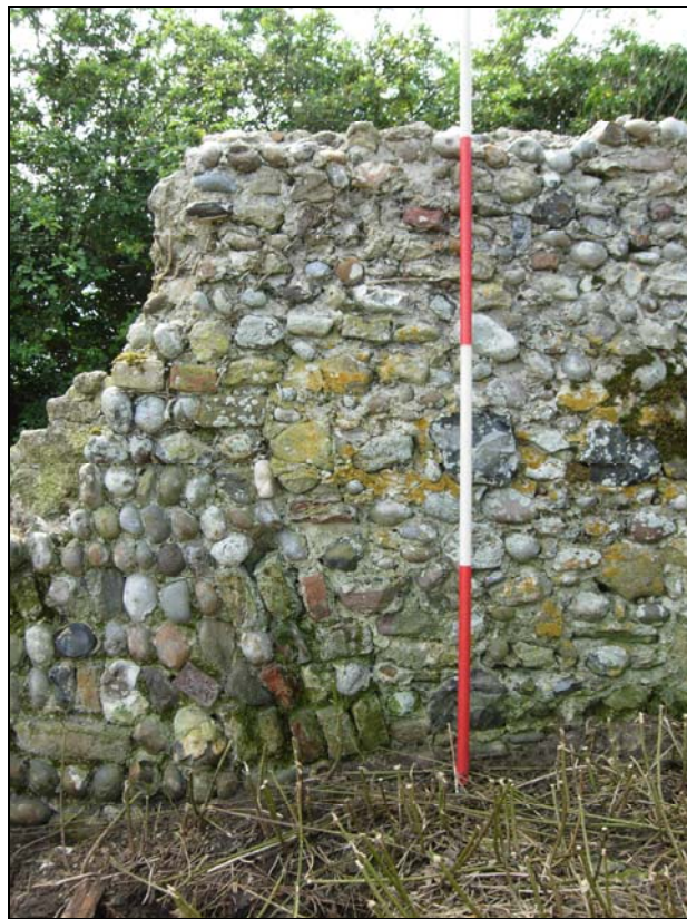
Plate 60. S. precinct wall: W. end, fabric joint, internal
