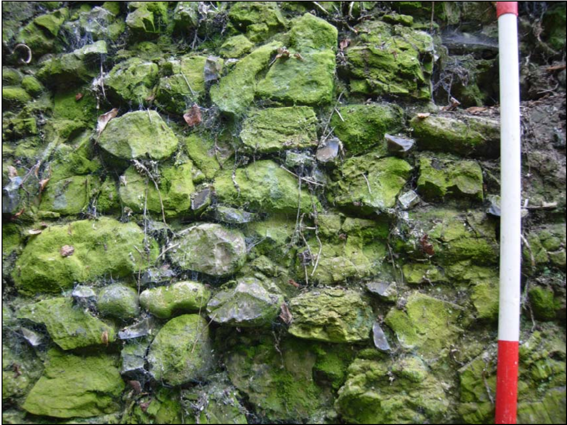
Plate 43. E. precinct wall: external, example of original medieval facing
