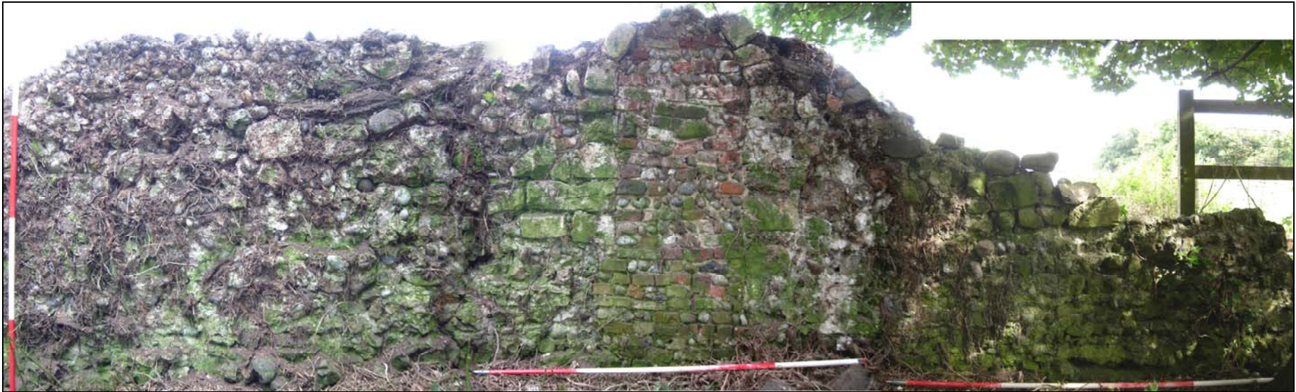
Plate 58. Precinct wall, SE corner: blocked doorway (external)
