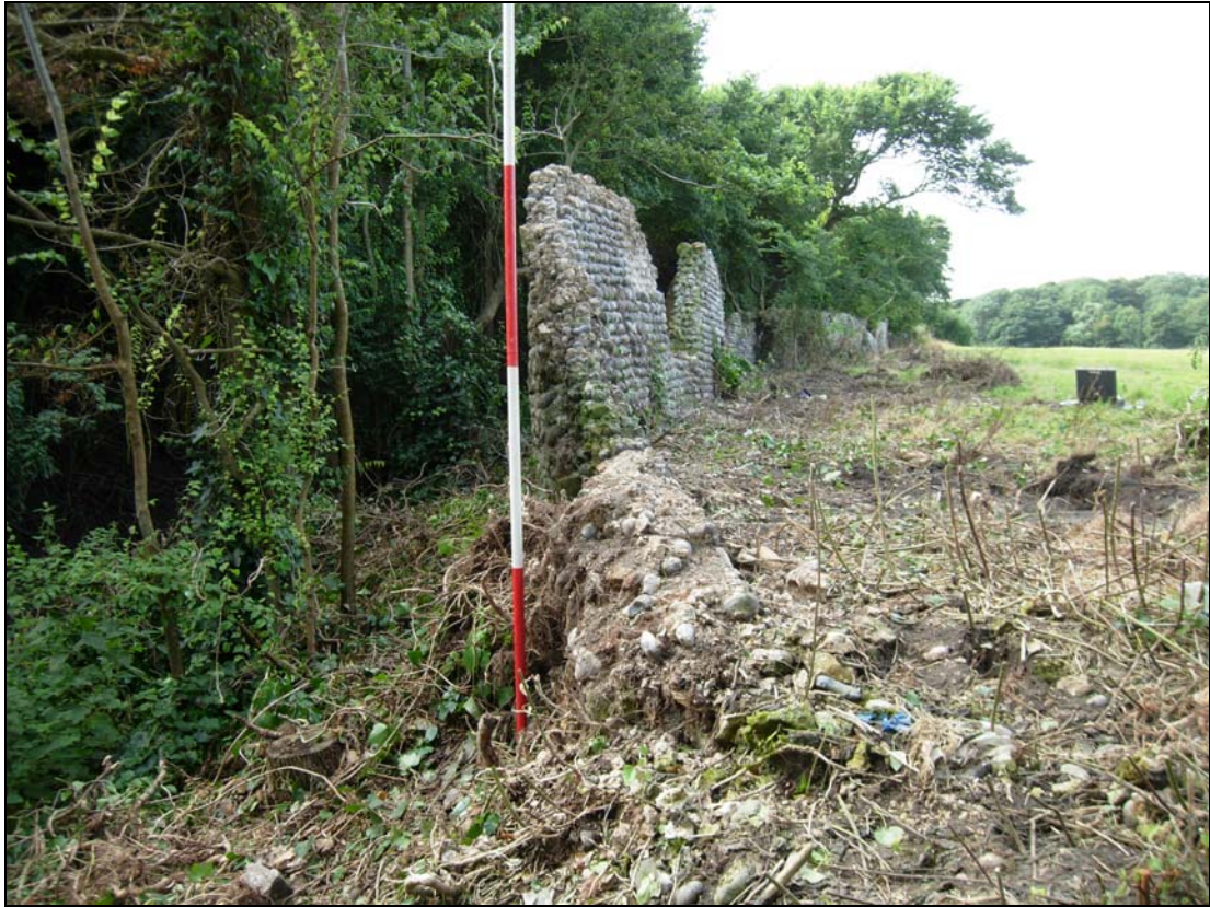
Plate 1. E. precinct wall: surviving stub from N.
