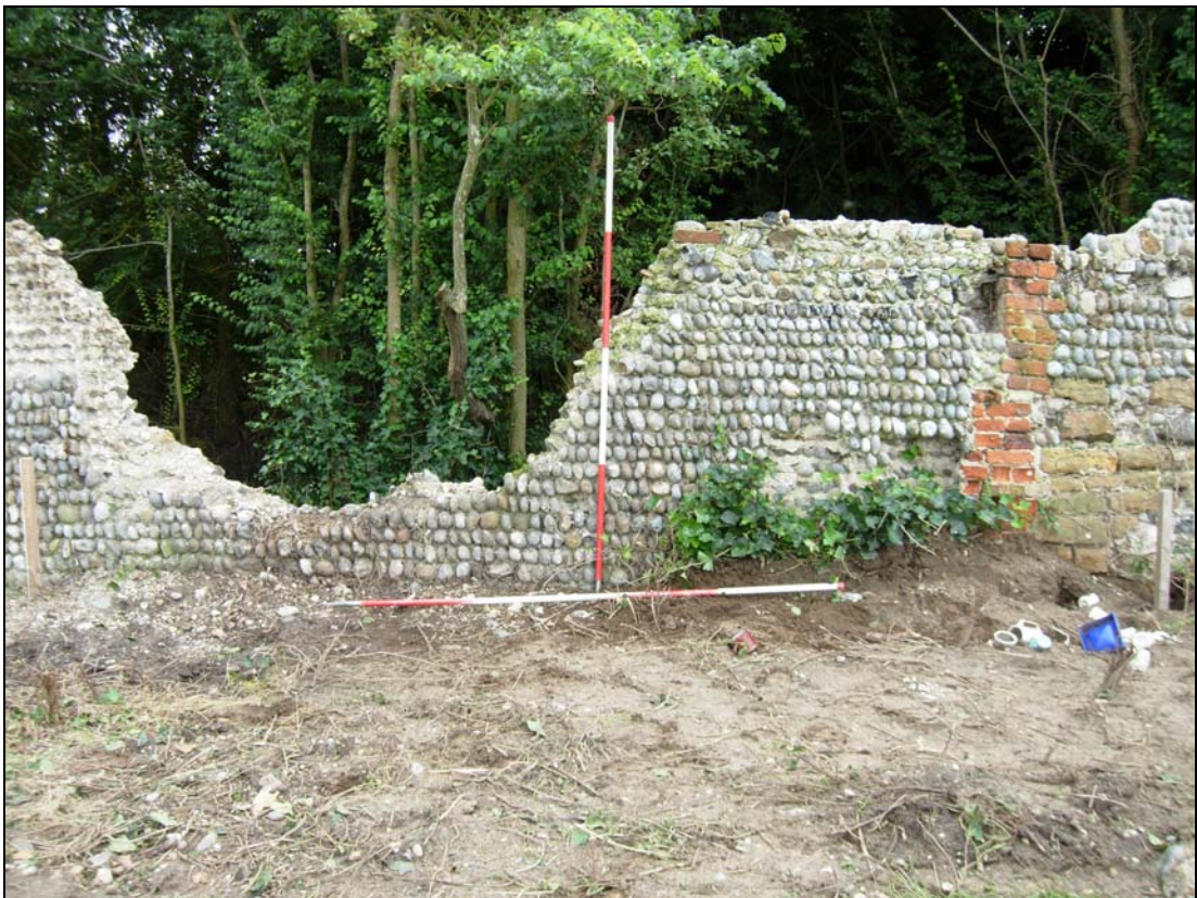
Plate 12. E. precinct wall: Stint 5 – 10m
