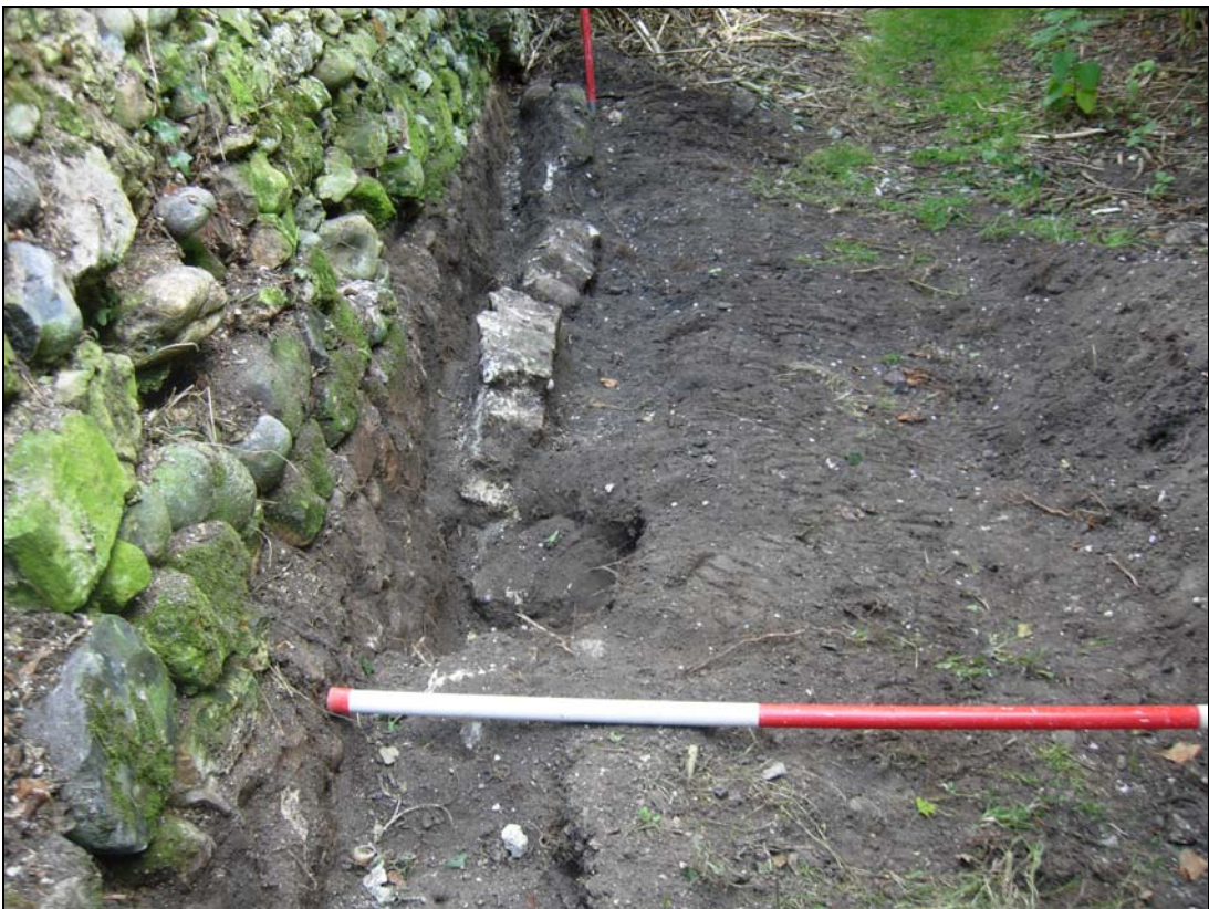
Plate 62. S. precinct wall: W. end, detached facing
