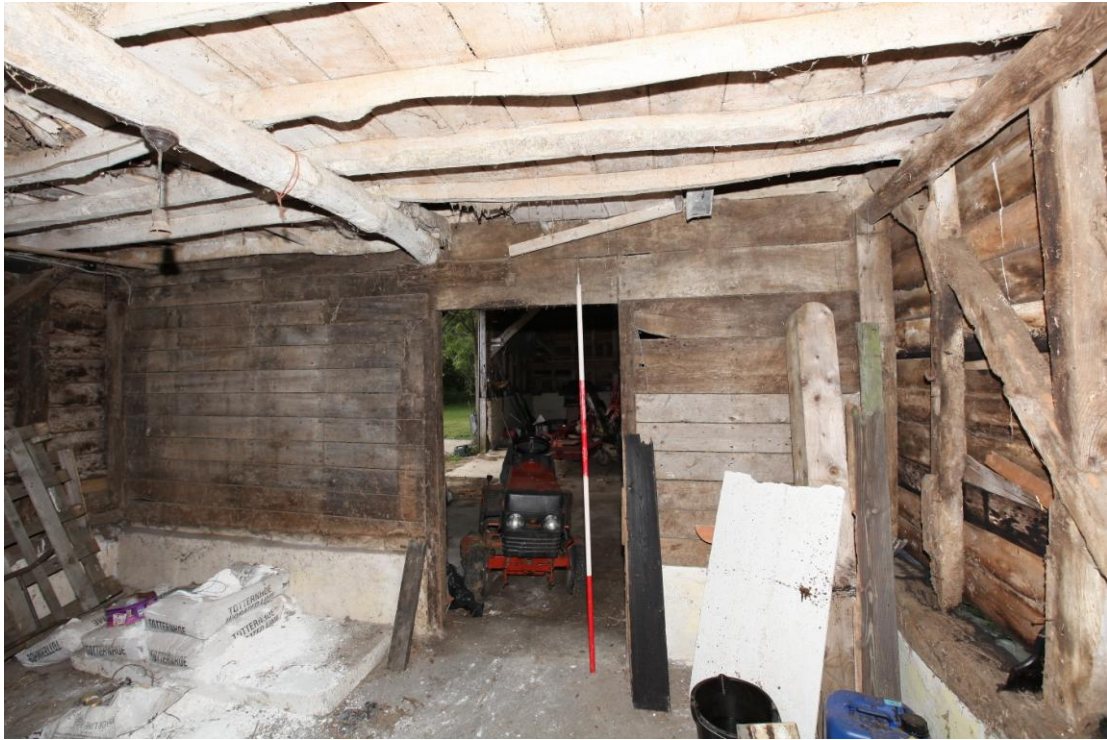
Illus. 9. The interior of the original stable bay (1b) from the east, showing the position of the missing manger and hay rack beneath the partial hay drop adjoining the internal partition against the threshing barn (1a) – now cut by a later connecting door.
