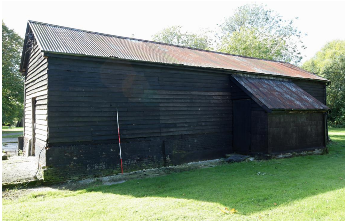
Illus. 2. The northern exterior of the barn from the remains of Allwood Green showing its corrugated iron roof, 20 th century weatherboarding and cement-block lean-to porch (1c) with a modern door in its eastern side-elevation.
