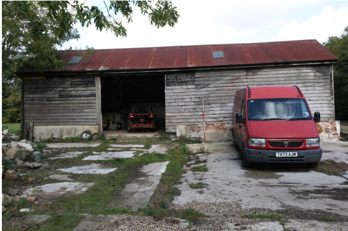
Illus. 3. The southern exterior bearing the roof scars of the two demolished 20 th century sheds shown in illus. 1 above with the original entrance in the central bay of the threshing barn (1a) to the left (lacking its doors).
