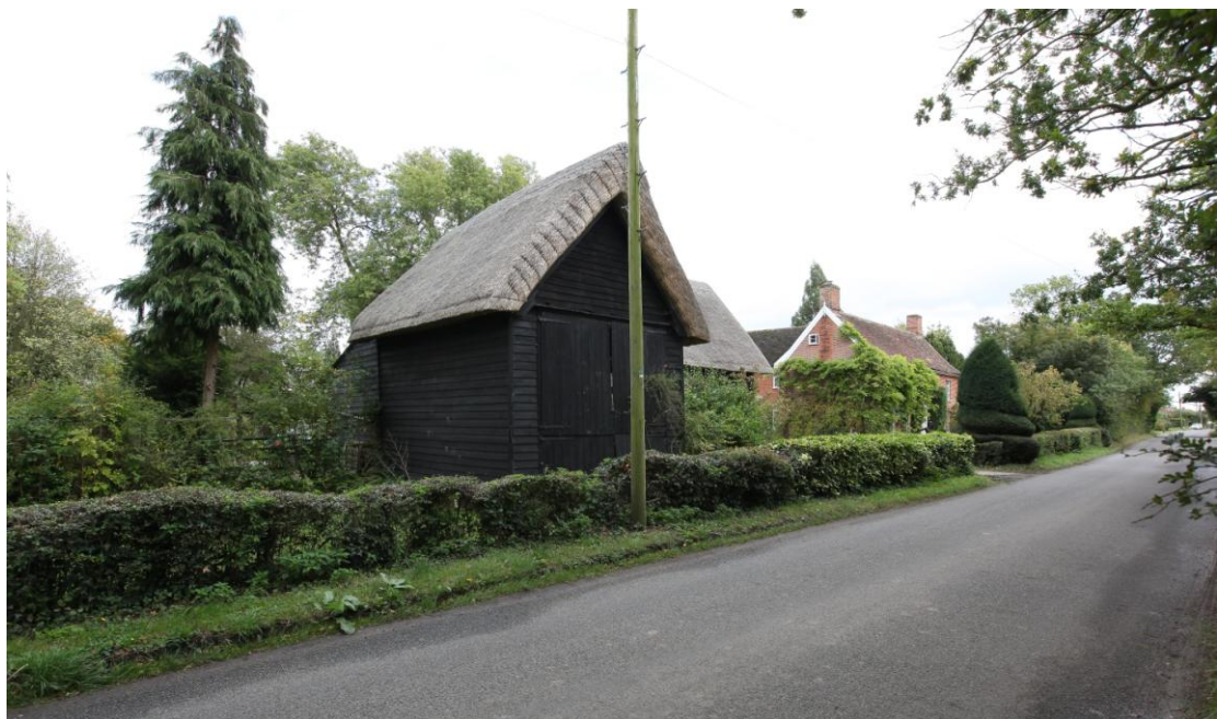
Illus. 2. A general view from the Eye Road to the north, showing the barn's porch (1) to the left and the farmhouse in the rear. The majority of the barn which this porch once abutted has been demolished, resulting in a highly distinctive building which forms the entrance to the village when approaching from this direction and makes a very significant contribution to the local landscape.
