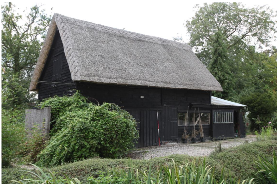
Illus. 4. The barn southern range from the south-east, showing the left loading hatch and the 19 th or early-20 th century weatherboarding which survives in the southern gable.
