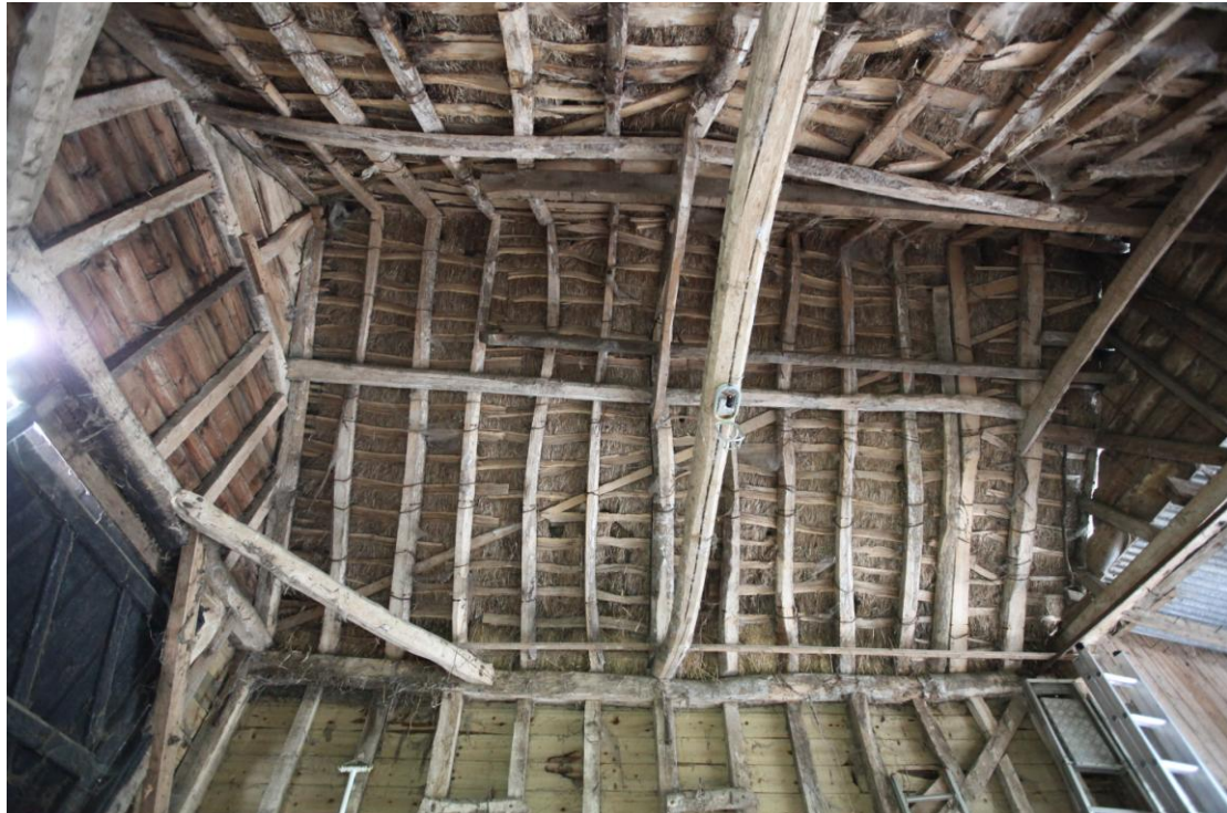
Illus. 8. The intact original clasp-purlin roof structure of the porch (1) showing its nailed collars and a central tie-beam without braces. These features are typical of the early-19 th century.
