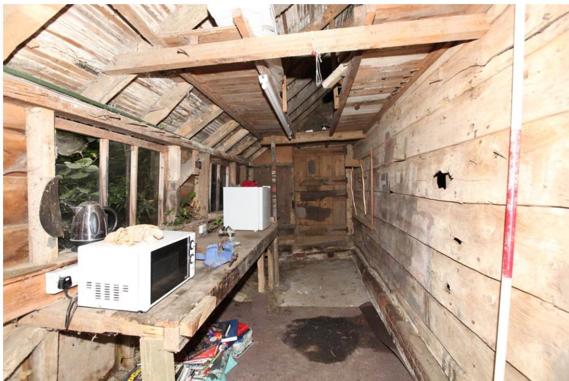
Illus. 10. The interior from the south of the 19 th century lean-to shed (4) in the angle of the porch (1) and the southern bay of the barn (2). The windows to the left are insertions of the 20 th century but the impressively wide boards to the right appear to be original to the barn.
