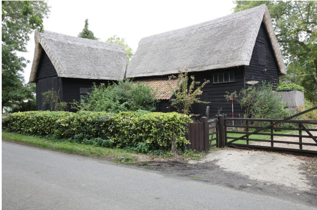
Illus. 3. The barn from the south-west, showing its distinctive L-shaped profile with two substantial thatched roofs adjoining corner-to-corner at right-angles. The pantiled western lean-to shed (4) is visible in the centre. The thatch is recent and most of the weatherboarding in this elevation was renewed as part of a heavy mid- to late-20 th century refurbishment. A number of modern windows which would otherwise detract from its traditional appearance are hidden by shrubs.
