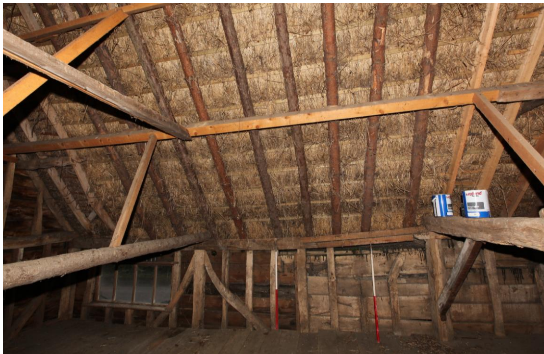
Illus. 14. The western interior of the former stable (3) showing the recently replaced rafters and purlins in the roof with the corner of the original barn (2) with a shaped terminal to its roof-plate on the right. The distinctively curved primary wall braces to the left are nailed to the post and the studs are tenoned but not pegged to the roof-plates unlike those of the earlier barn.
