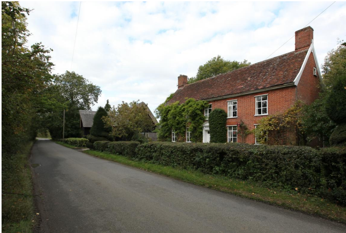
Illus. 1. A general view of the site from the Eye Road to the south showing the imposing Georgian brick facade of the grade II-listed farmhouse to the right with the barn in the rear to the left.
