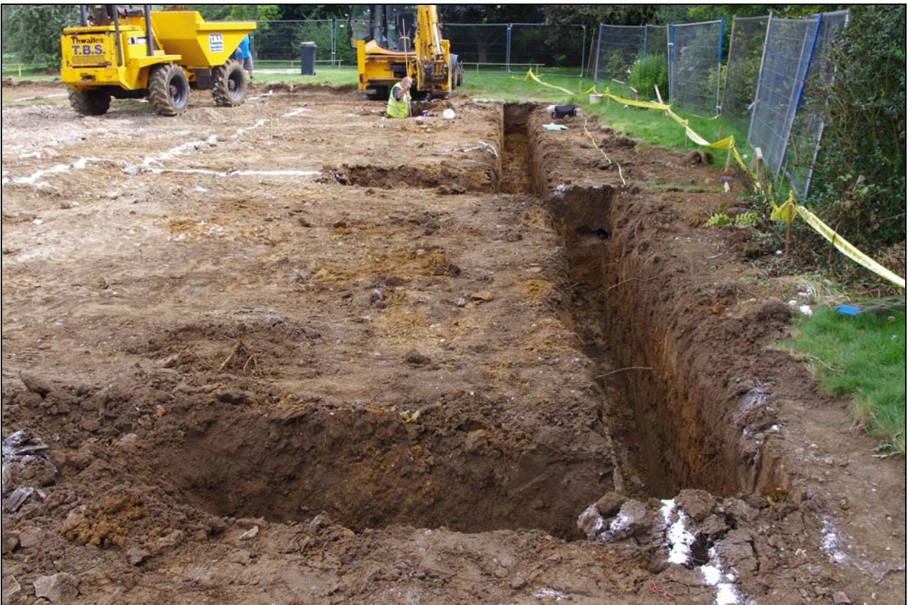
Plate 6. Excavation of House Plot 2, showing site conditions, facing ENE
