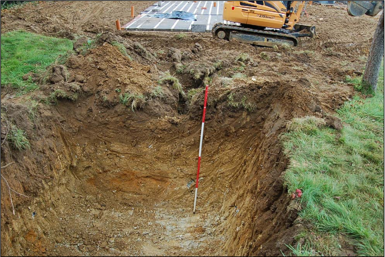
Plate 5. Rainwater harvesting tank pit, by House Plot 1, facing ENE, 2m scale
