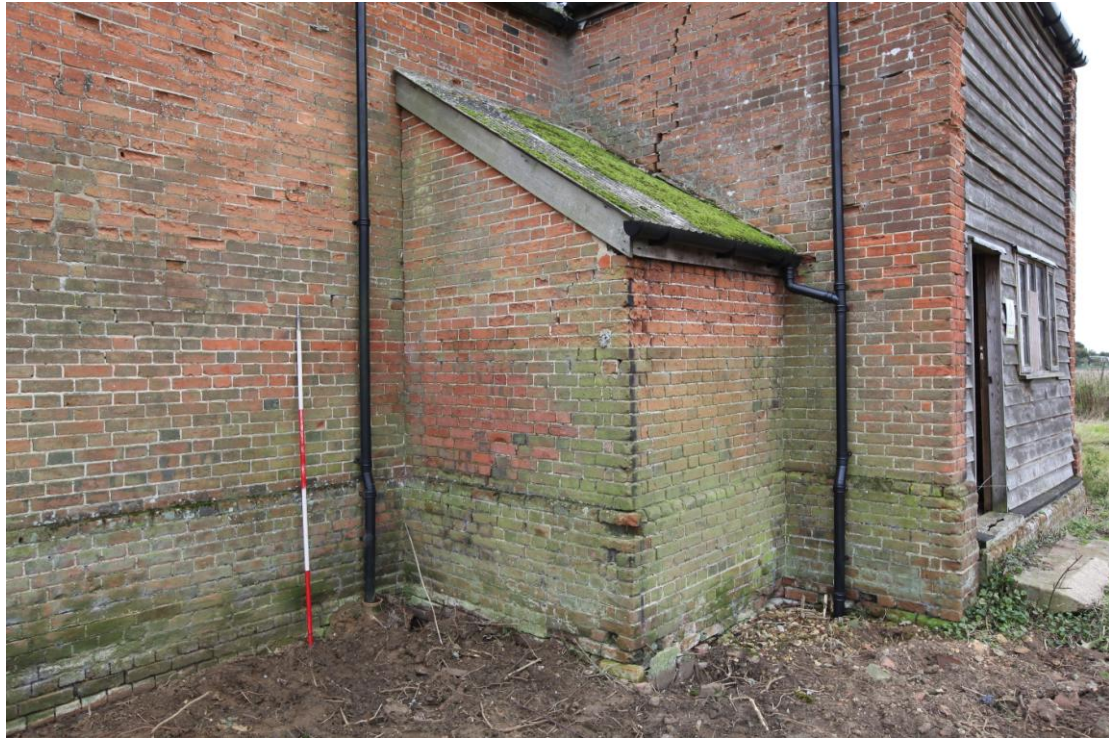
Illus. 3. The lean-to shed to the north of the porch showing its largely original brickwork (keyed to both the porch and barn) to a height of 1.8 m, with the lighter bricks of a seven-course lift beneath the eaves of the present 20 th century roof structure. The later brickwork is not keyed to the barn.
