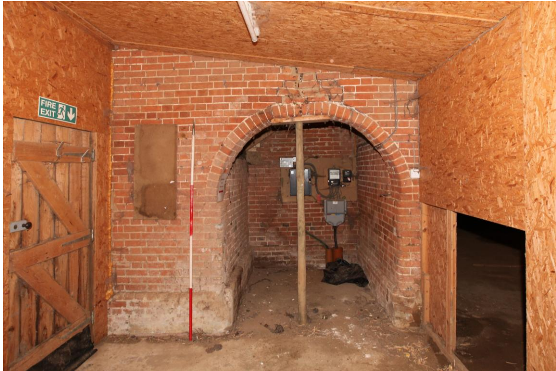
Illus. 5. The interior of the porch from the south, showing the original arched opening to the integral lean-to shed. Two wooden blocks are set into the brickwork of both piers, presumably to secure the jambs or rails of a boarded hatch or partition, and the shed is likely to have operated as a grain store adjoining the threshing floor. The fire-board ceiling and partition to the main barn on the right are late-20 th century insertions.
