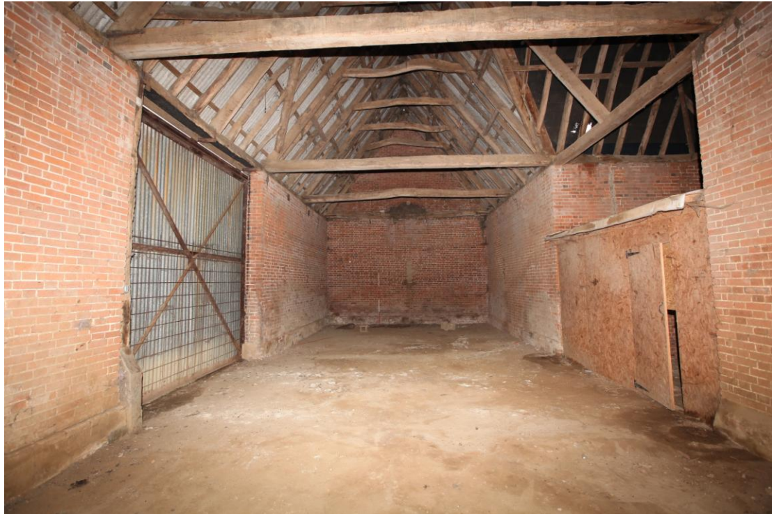
Illus. 7. The interior of the barn from the north with the original full-height entrance in the centre of the eastern elevation to the left, immediately opposite the western porch with its modern fibre-board partition on the right. The floor is of concrete throughout.
