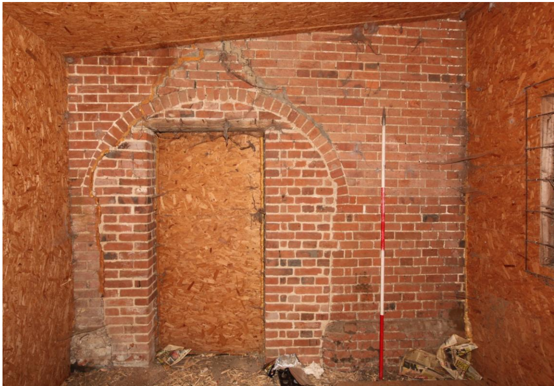
Illus. 6. The interior of the porch from the north, showing the identical arched aperture to the demolished southern lean-to shed and its subsequent reduction to form the narrow doorway in illus. 4 above.
