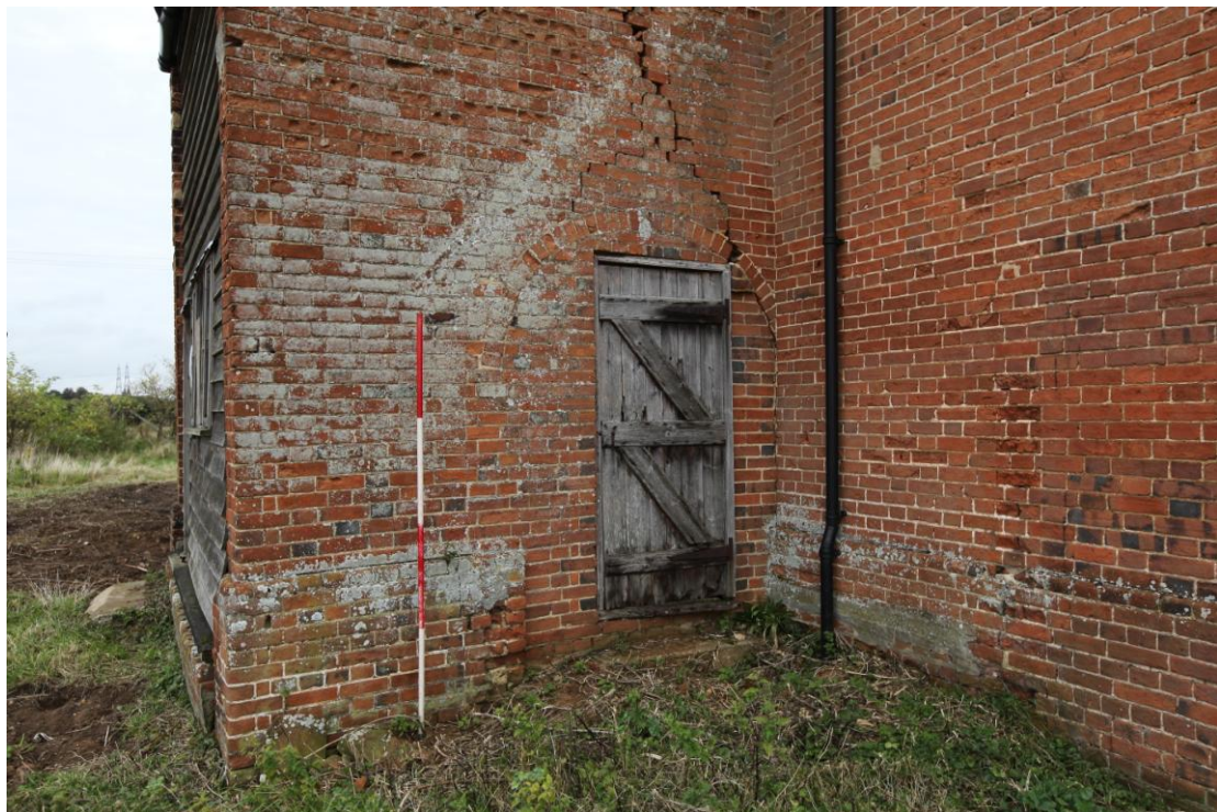
Illus. 4. The southern elevation of the porch showing the arched aperture and roof scar of a demolished lean-to shed which reflected its remaining counterpart to the north. The scar of its southern wall is visible in the brickwork of the barn to the right. The narrow doorway is a later insertion into the arch.
