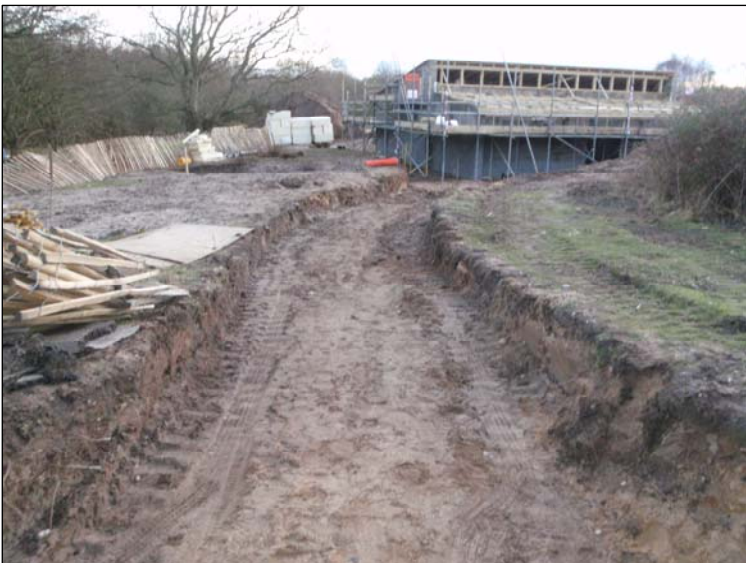
Plate 4. General view of the stripped access road
