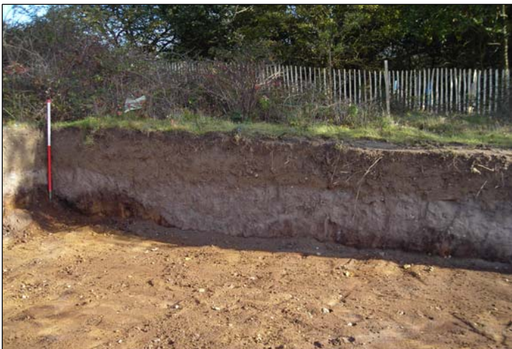
Plate 1. Ditch profiles exposed in the NW-SE section of the building footprint
