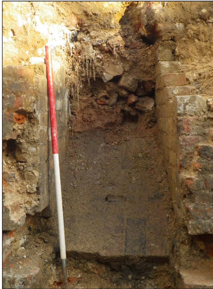
Plate 20. Coal chute 0131 inserted in the east wall of the northern cellar extension. 1m scale.
