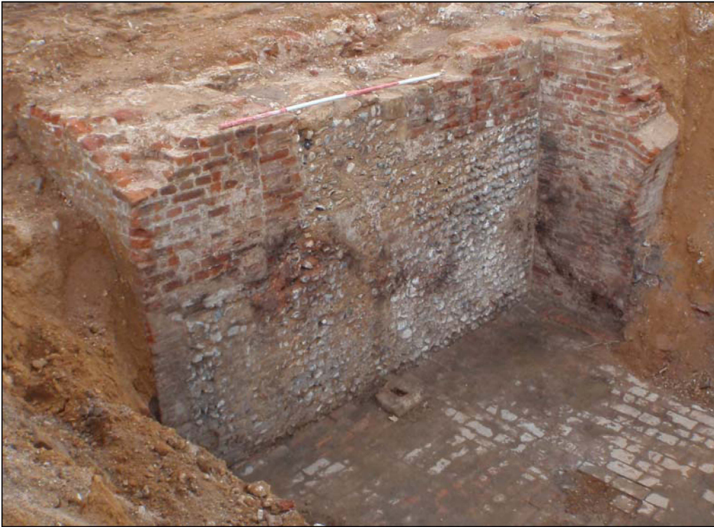
Plate 2. East wall of the cellar 0114, looking south. The northern edge has been finished with bricks where the early cellar wall returned for the post-medieval cellar steps. The Norman flint coursing is clearly visible and continues behind the later brick arch 0122 visible to the right of the picture. Although not in its original position, a padstone with a slot for a tenon can be seen against the wall and is matched by the ghost of a setting in the middle of the brick floor. 1x2m scale.
