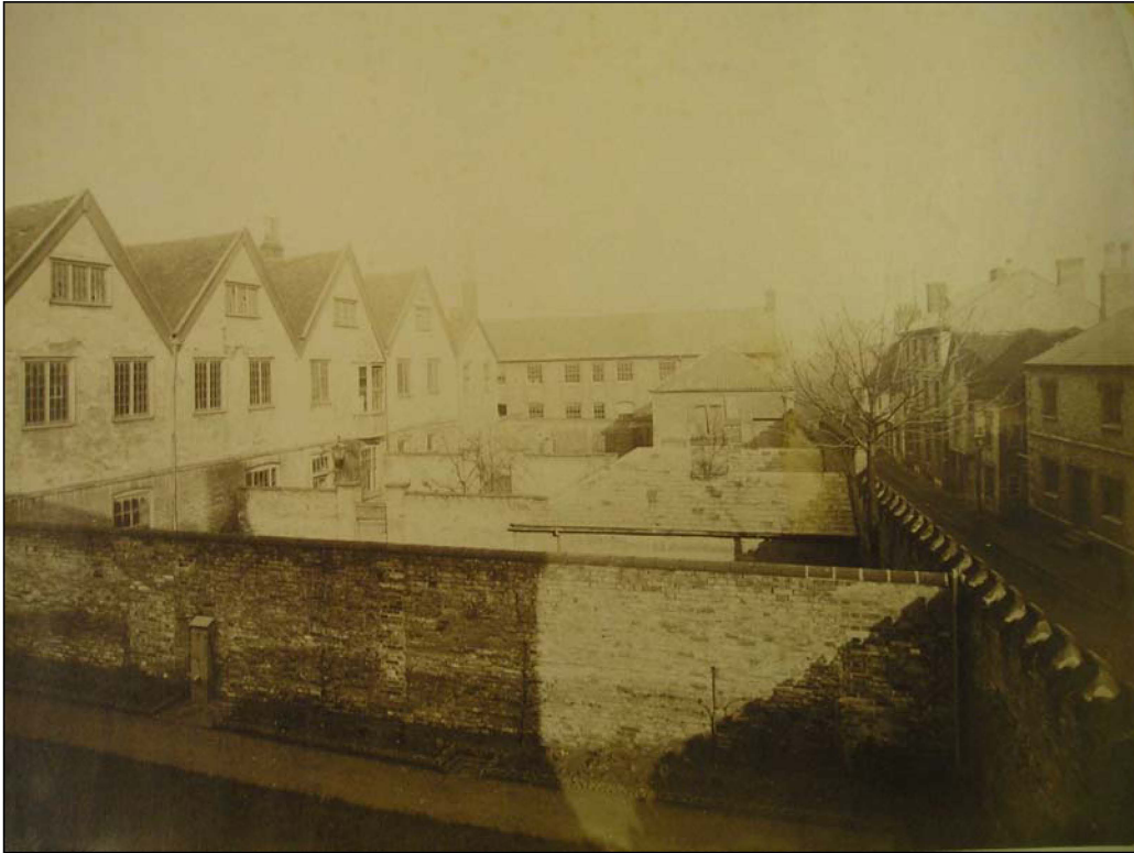
Plate. View of the workhouse (ref. K511/476)
