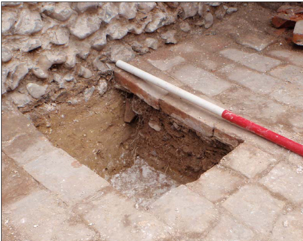
Plate 5. Sondage through floor. The clay foundation for the east wall 0117 is visible, also showing beneath a later tile floor are the remains of a clay floor 0093 laid directly over natural chalk. The scale bars are at 0.5m.
