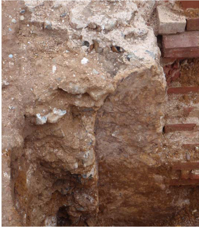
Plate 11. Looking west onto the top of the inserted cross wall 0121. Showing the impression of a wide flat 'Tudor' arch in the mortar.
