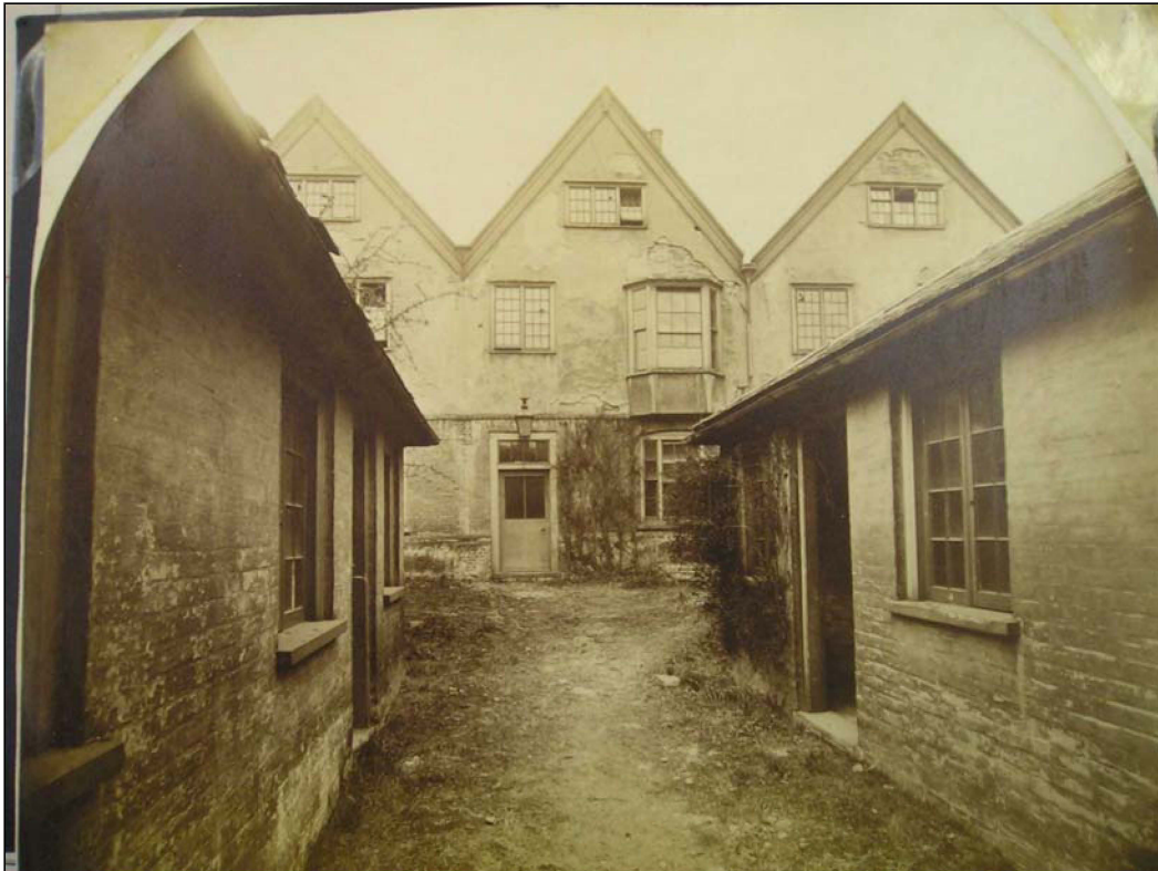
Plate. View of the main workhouse building (ref. K511/478)
