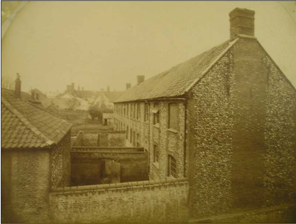
Plate. Buildings on the north side of the site (ref. K511/479)
