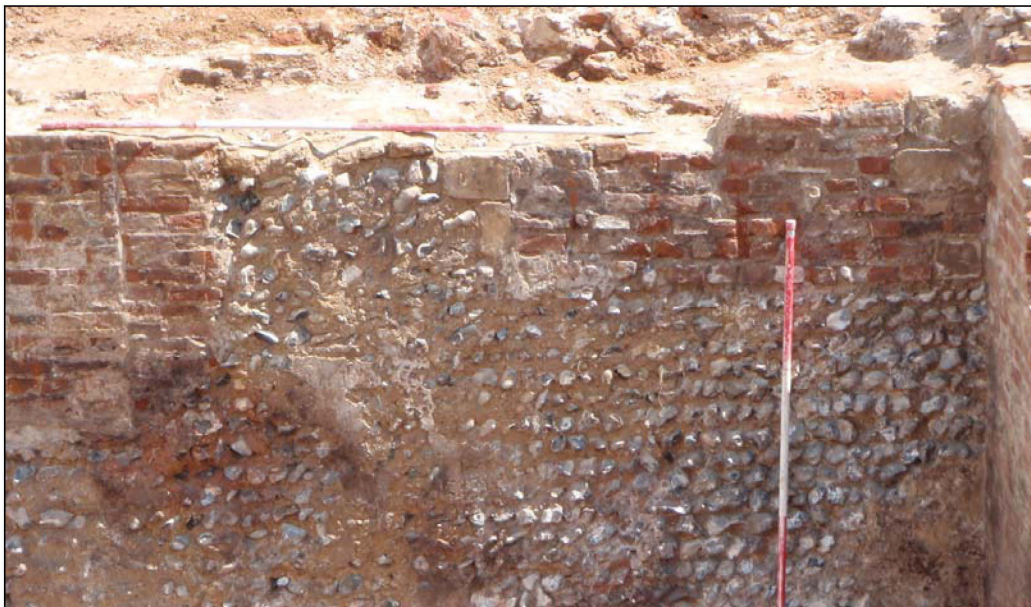
Plate 3. East wall 0114 detail. Showing in situ ashlar blocks in the centre of the picture indicating the edge of an opening 0118 later in-filled with bricks. Overlapping limestone rubble is visible beneath the horizontal ranging pole. The scale bars are at 0.5m.
