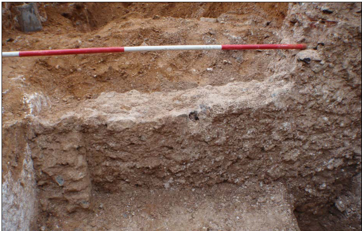
Plate 10. Inserted cross wall 0121. Blocking off the corridor leading into the main cellar (the wall was later punched through for a set of steps for a post-medieval building). The photograph is taken looking east into the rough back face of the cross wall. The scale bars are 0.5m.
