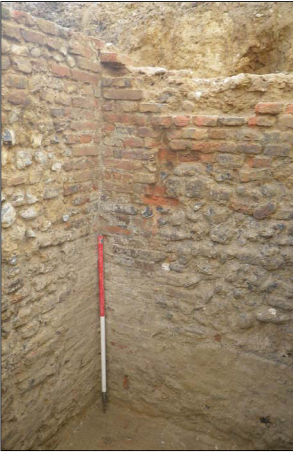
Plate 13. Detail of south-west corner of extension 0124. 1m scale.
