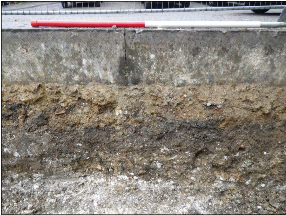
Plate 1. Section 1; Trench profile at west end of exterior footings, facing south-west (1m scale).
