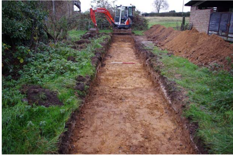
Plate 1. General view of the evaluation trench, looking north (1m scale)
