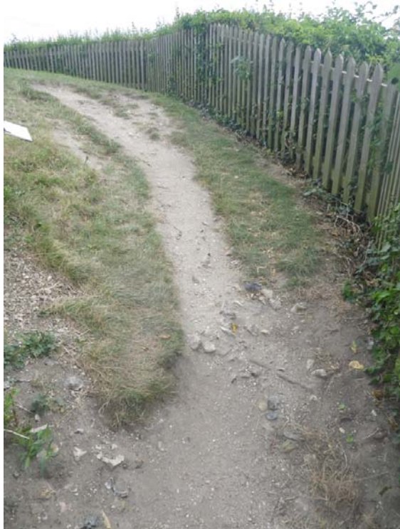
Plate 9. Erosion to the path exposing buried flint foundations
