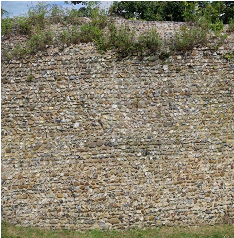
Plate 13. The flints of the bailey wall laid in strong horizontal courses that follow the rise and fall of the wall's contours. The flints appear banded, divided by 'string courses' of flints which have been sorted for size and shape and which include elongated oval flints which have been laid in a herring-bone pattern. The 'string-courses' are evenly spaced bands at under 1m apart and presumably indicate building lifts (Higher View photograph).
