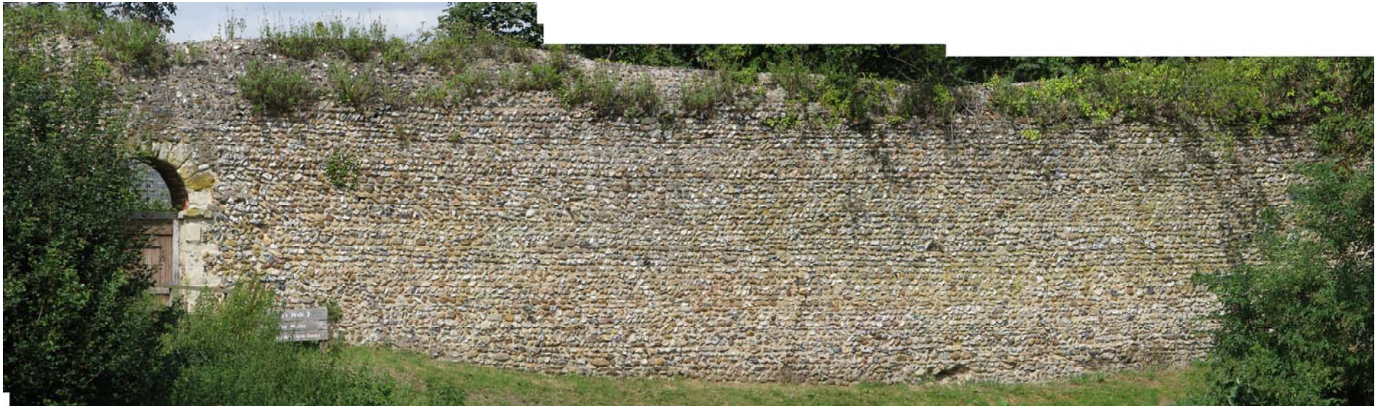
Plate 12. The south face of the bailey north wall. It's is over 4m high and 50m long and built without supporting buttresses; it is a striking example of Norman wall building. The door on the left is a later insert the rusticated block work is a Palladian style and probably dates to the 17th-18th century (Higher View photograph).
