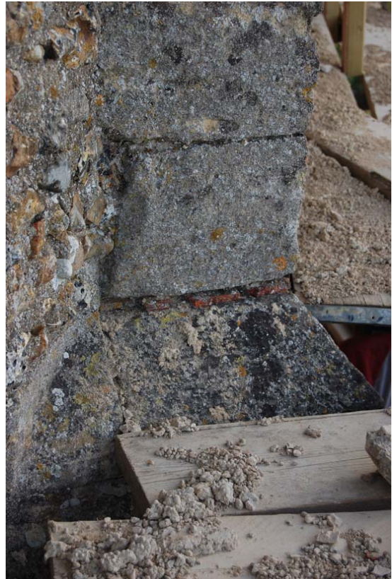
Plate 10. Post-medieval tile inserted into the joints of the buttresses
