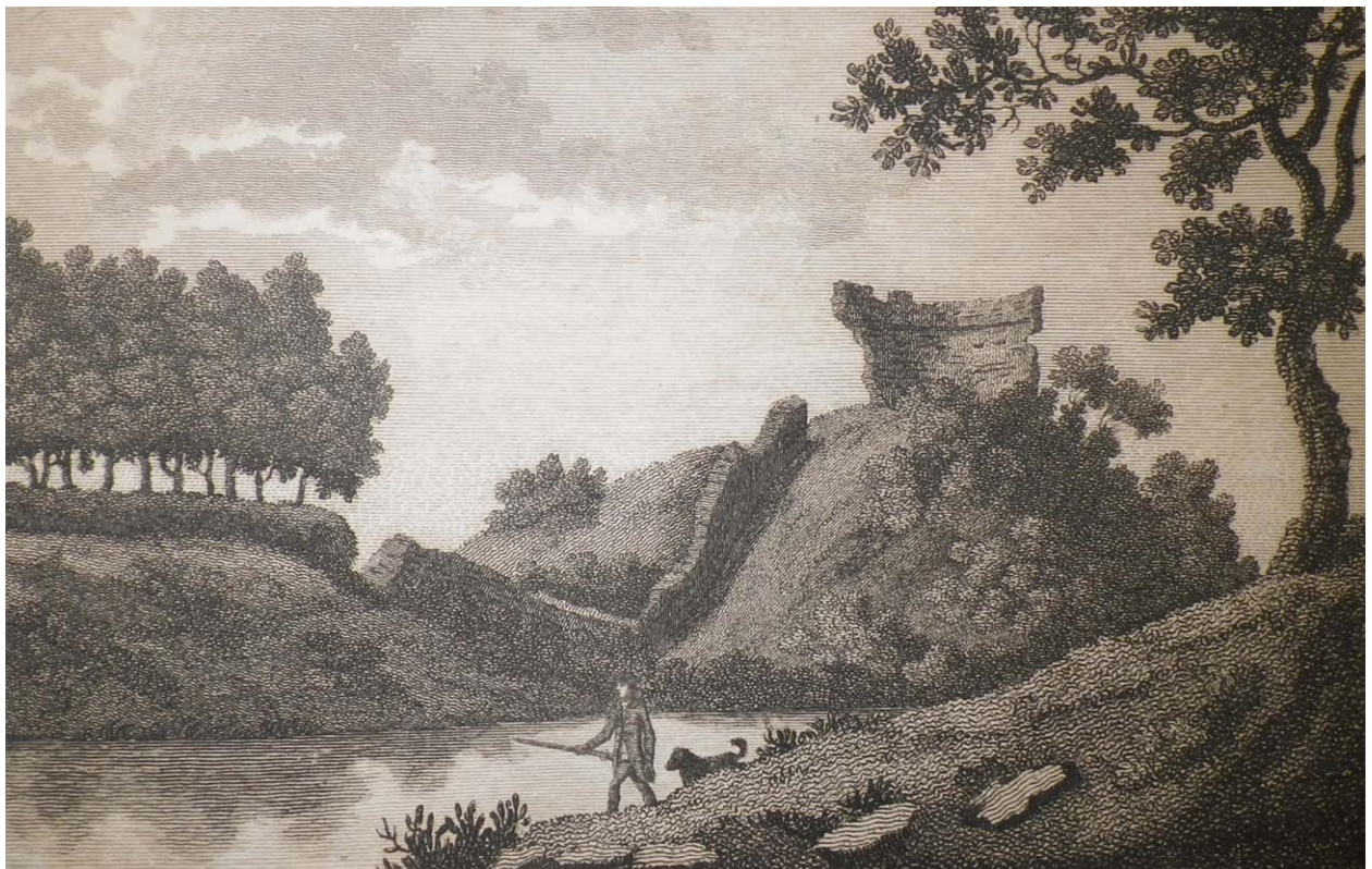
Figure 6. An engraving of Clare Castle by J Newton published 1787 (BRO ref 1511/67/13) showing clearly the parapet with crenulations and a row of putlock holes below
