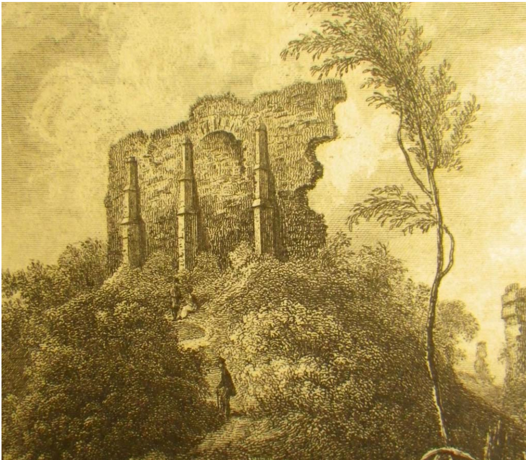
Figure 8. An engraving of the castle keep by J Haworth 1840 (Bury RO ref 1511/67/09). Note the arched feature between the buttresses, this is no longer visible on the exterior surface and was not identified within the core on the interior of the wall. The parapet is truncated with no indication of the crenulations
