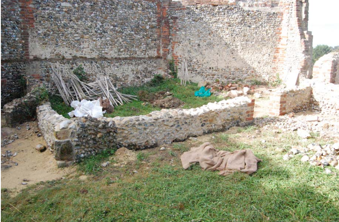
Plate 18. The same wall following the remedial work.
