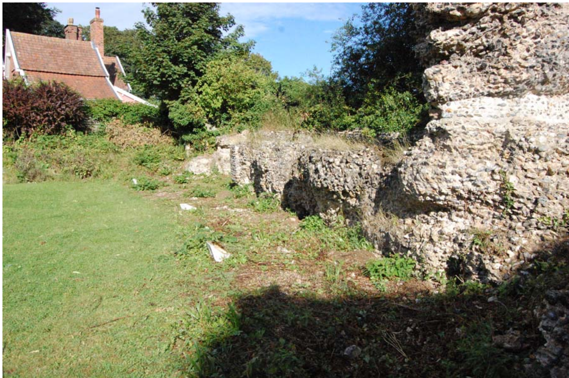
Plate 4. South exterior elevation bailey wall looking NW. None of the original Norman face-work survives and the core fabric is exposed. This is scarred with horizontal 'gouges' seen running E-W across the face and in profile in the elevated section in the foreground; similar gouges were observed running N-S across the face of the partition wall.
