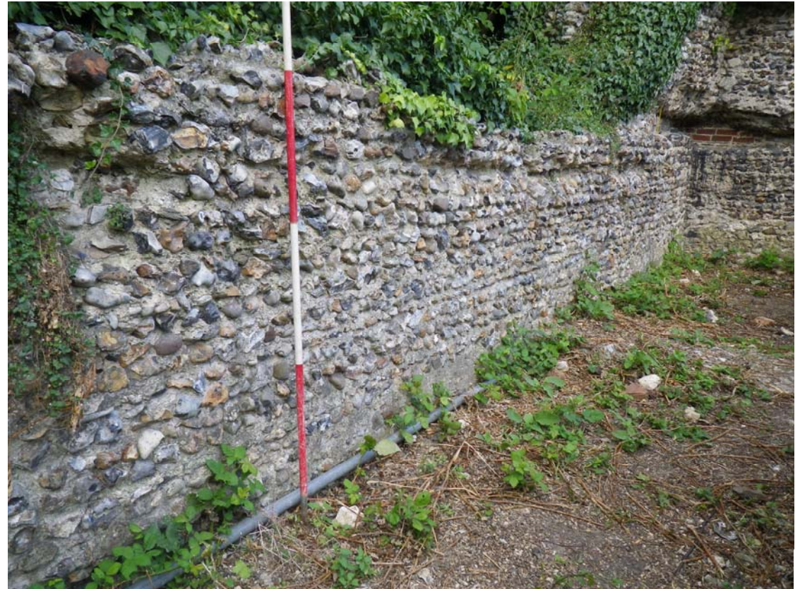
Plate 8. Interior (south) face of the north wall of chambers 1 and 2 showing the flints laid in neat horizontal courses typical of the work of Norman masons.
