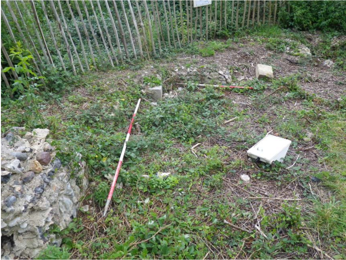
Plate 15. Truncated remains of the east tower. The ranging pole are aligned with the tower walls, the block of stone where the pole meet is an in-situ quoin.
