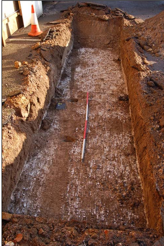
Plate 3. Trench 3, facing east showing modern service run to left of scale (2m scale)
