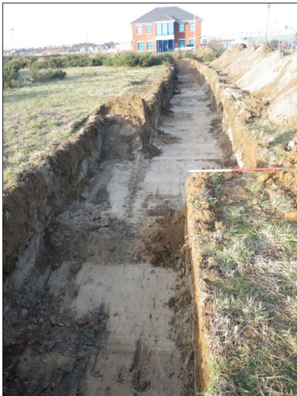
Plate 1. Trench 1, looking NNW
