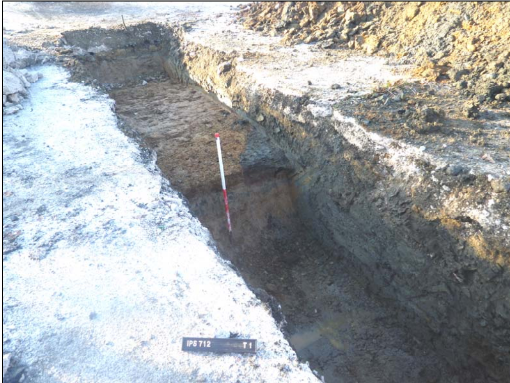
Plate 1 Trench 1: edge of ditch 0008
