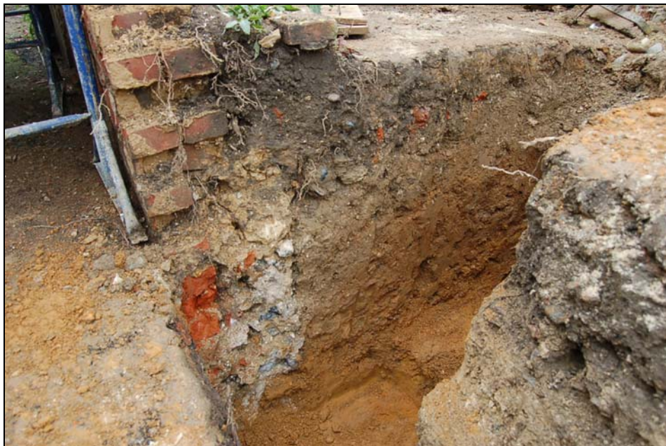
Flint wall under existing brick wall (footpath to left of picture)
