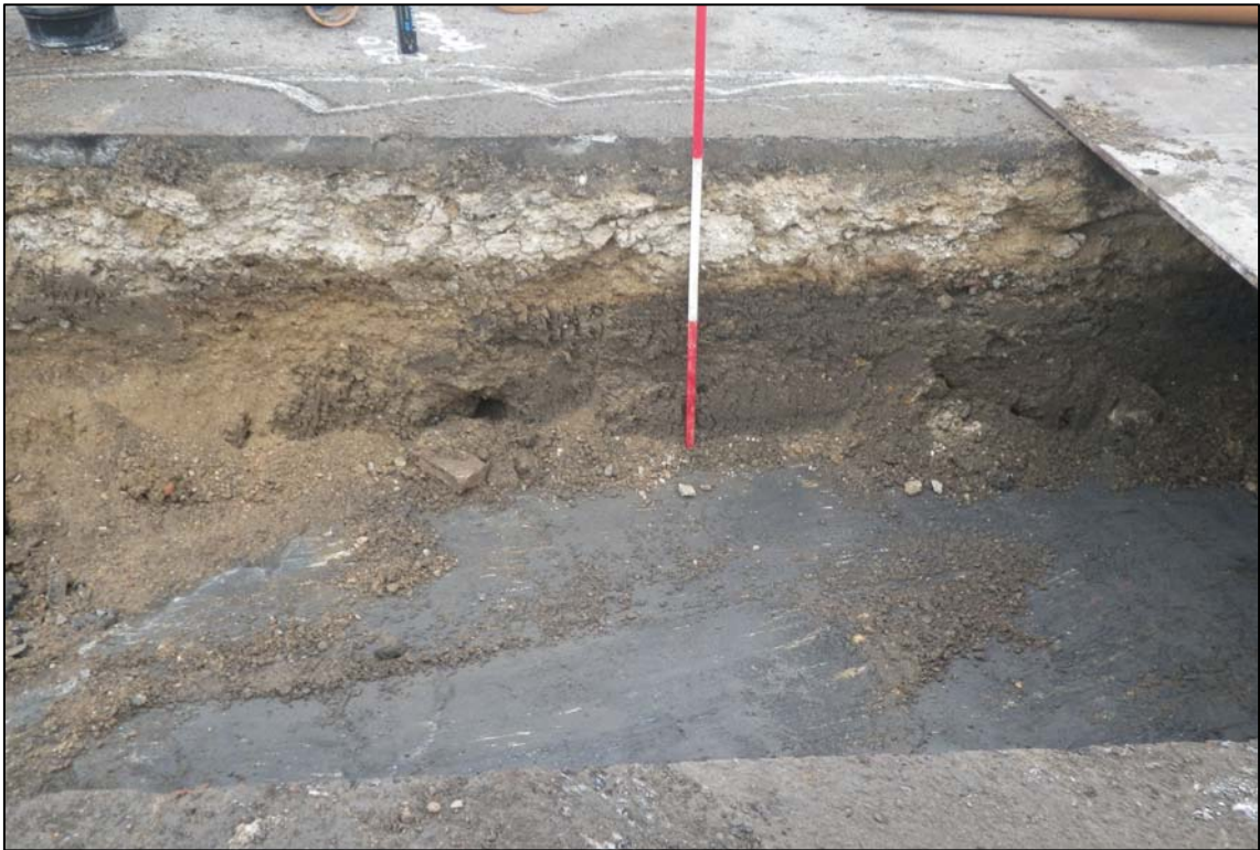
Plate 1. Concrete floor at west end of the building, camera facing north-east (ref. HSS 03)
