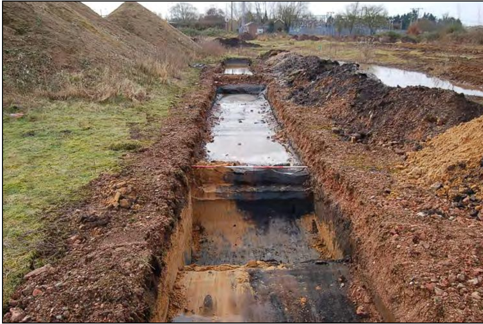
Plate 12. Trench 14 facing south showing machine sondage (2m scale)
