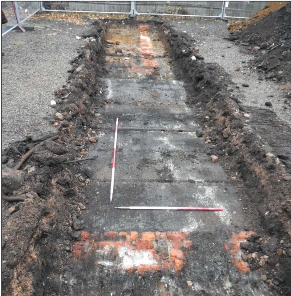
Plate 8. Trench 2 view facing north, Wall 0054 in foreground (ref. HSV 78)
