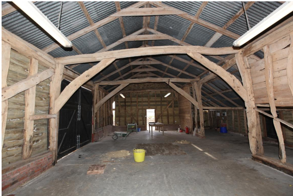
Illus. 8. The interior of the barn from the east showing the profiles of its original arch-braced tie-beams. Both gables were entirely rebuilt in the 19 th century and the roof is a 20 th century replacement. The original roof is likely to have been steeply pitched at 55 degrees for thatch.
