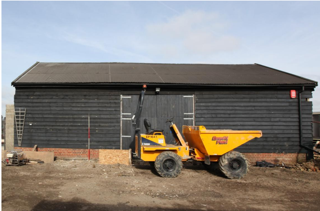
Illus. 3. The southern exterior of the barn (1) showing its modern brick plinth and stained weatherboarding. The central doors are also modern but occupy the same position as the original full-height doors which faced away from the farmhouse.
