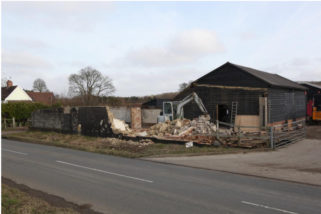
Illus. 1. The site from Willisham Road to the west, showing the barn (1) to the right, the grade II-listed farmhouse to the left and the remains of the mid-19 th century shed of shuttered clay (2) in the foreground.
