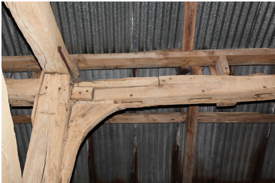
Illus. 10. A detail of the northern roof-plate of the central bay showing the 15 th or 16 th century type edge-halved and bridled scarf joint with double tenon pegs to the left and the studs of the removed back wall to the right. The mortise on the extreme right is central to the bay and is significantly smaller than its counterparts, having secured a short stud above the lintel of the original low, narrow rear doorway. The knee-brace on the left is a nailed insertion.
