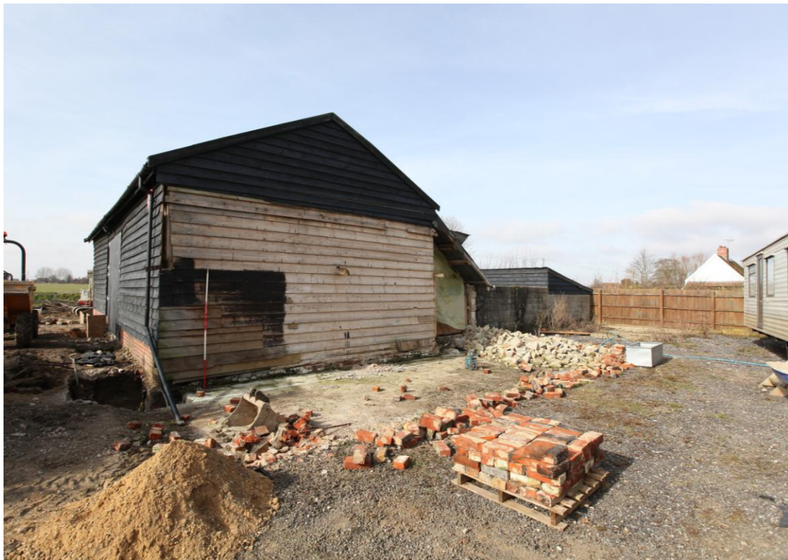
Illus. 6. The barn (1) from the east showing the scar of a recently demolished shed adjoining its gable with its rear lean-to and the shelter-shed (3) and farmhouse (5) visible to the right.
