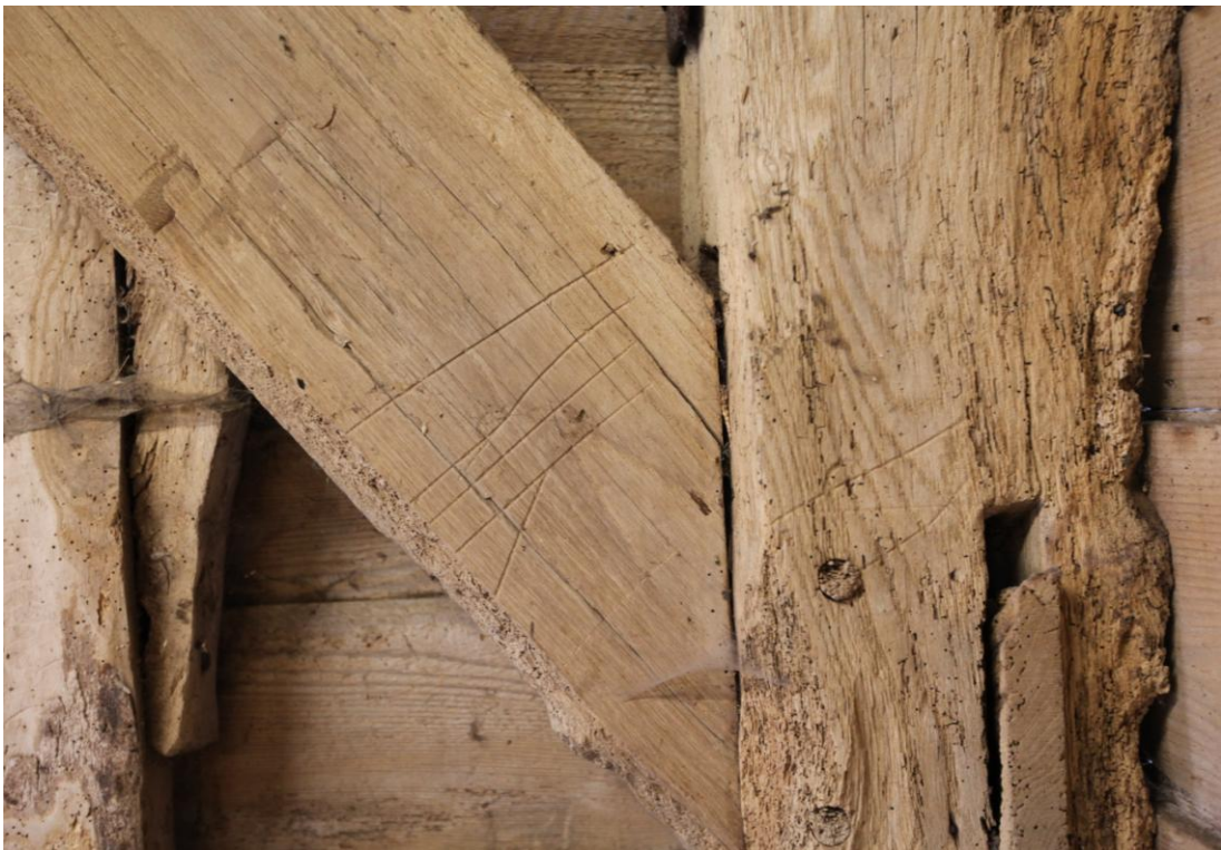
Illus. 12. A detail of an incised carpenter's Roman numeral to the northern internal brace of the eastern bay (to the right in illus. 11 above).
