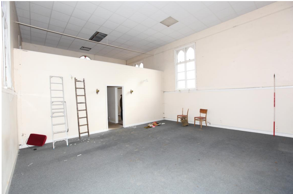
Illus. 10. The main hall (1) from the west showing the circa 1970s partitions and ceiling tiles. Wooden wainscot may survive behind modern boarding under the dado rail.
