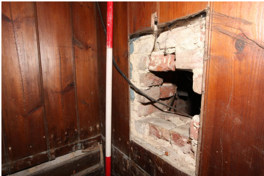
Illus. 8. A detail of the south-western internal corner of the wainscot panelling which surrounds the dais (1a). The aperture on the right connects with the small shed shown in illus. 3 and reveals the original painted plaster beneath the later panelling. The shed may have housed a generator.
