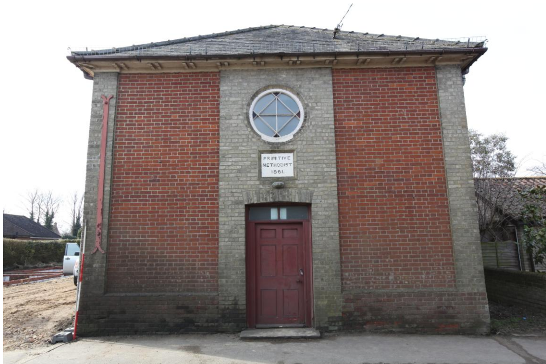
Illus. 4. The eastern external gable showing the six-panel 19 th century central entrance door a stained glass roundel and foundation plaque above. The plaque appears to consist of painted cement and reads 'PRIMITIVE MEHODIST 1861.' It may have been salvaged from the original eastern gable, which was set back from the road behind a small garden.
