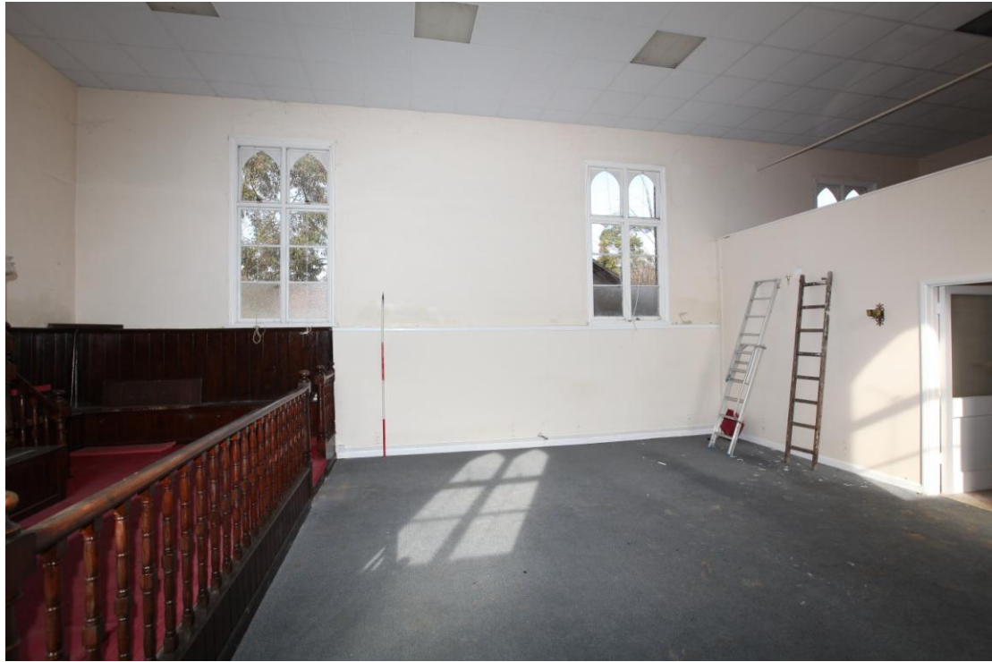
Illus. 9. The northern interior of the main hall (1) showing the dais to the left and the circa 1970s partitions forming a balcony above a kitchen and ‘committee room’ on the right. These partitions interrupt the eastern windows and the interior appears to have contained only a single large hall initially (perhaps with an internal porch of which no trace remains).
