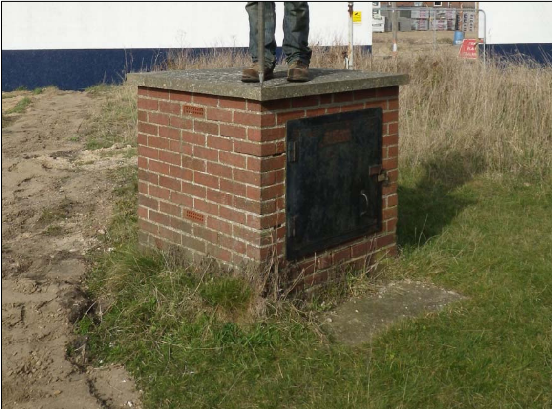
Plate 7. brick structure, camera facing northwest (ref. HTA 13)
