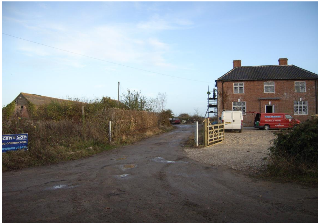
Illus. 1. The entrance to the site from Smiths Road to the west showing the grade II-listed red-brick farmhouse to the right and the farm buildings to the left.
