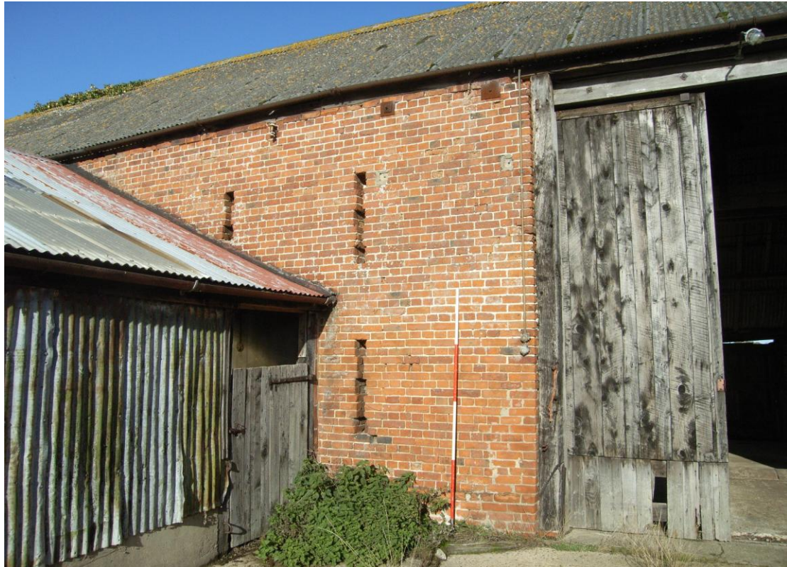
Illus. 7. The southern exterior of the two western bays of the threshing barn (1a) showing three of their six ventilation loops (the rest obscured by the 20th century covered cattle yard (4) to the left) and the original entrance to the right.
