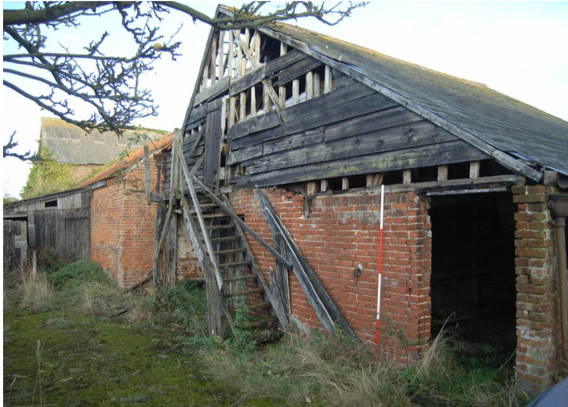
Illus. 13. The western gable of the granary (5) from the south-west showing the partly collapsed external stair to the grain floor and the entrance to the western section of a lean-to southern storage shed.
