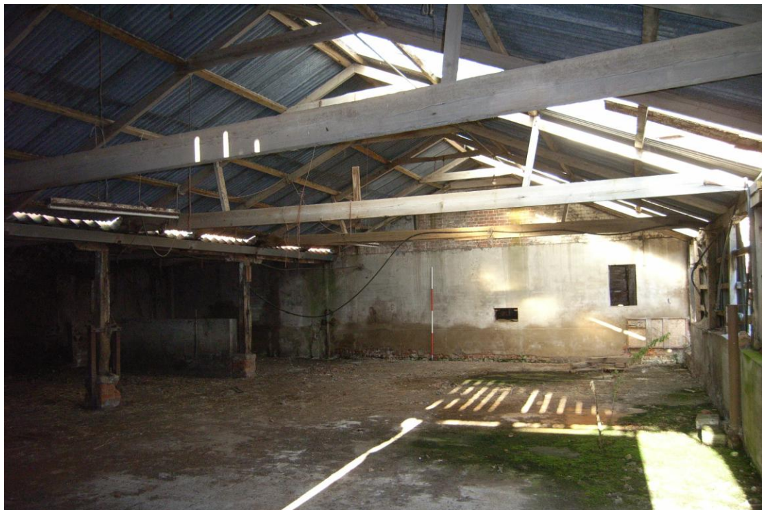
Illus. 12. The interior from the south of the 20th century covered cattle yard (4) showing the 19th century shelter-shed (3) to the left and the partly cement-rendered brickwork of the barn (1) in the rear.
