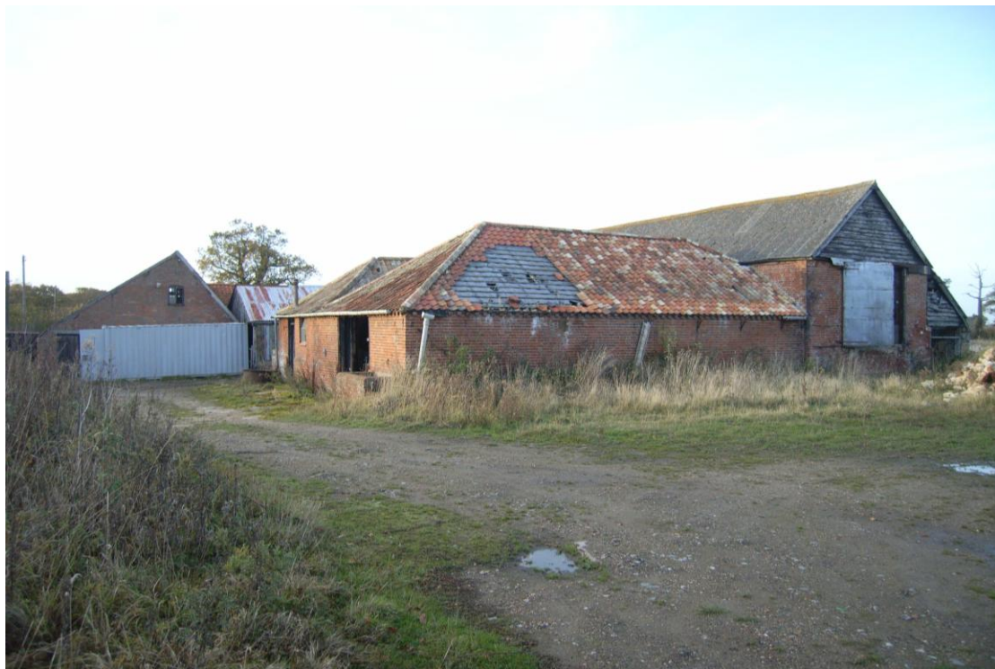
Illus. 2. A general view of the group from the south-east showing the asbestos-covered brick barn (1) in the rear to the right, the pantiled 'double-pile' cattle shed (2) in the foreground and the brick granary (5) to the left.
