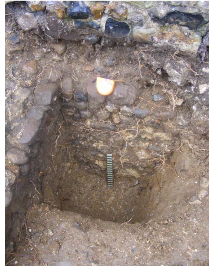
Plate 5. Excavation against the west side of the butters against the angle with the south wall showing the well-constructed foundation of the butters and south wall to the same depth.
