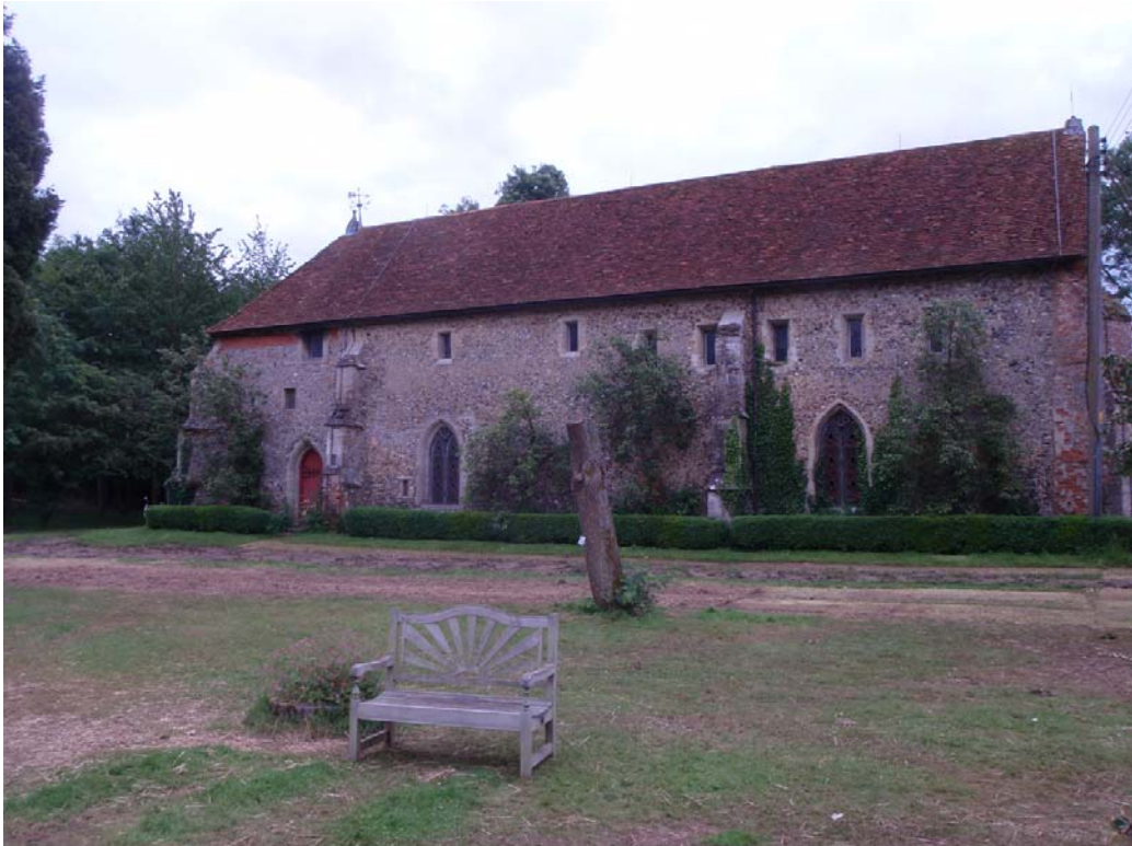
Plate 14. General view of the north side of the church. Note the first floor windows are at different levels suggesting that the central internal space may have been separated from the one within the west end (right) and which necessitated separate entrances (via the outshot stair on the south side and the west gable end door). On the ground floor the westernmost window is the only other original opening and together with its opposing window the only indication of how the ground floor was lit. The C19th arched window at the east end cuts a possible small square window at high level in the central area.
