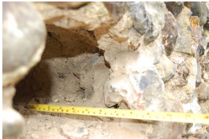
Detail of test hole A
