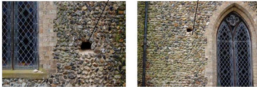
Locations of Test-holes A and B
