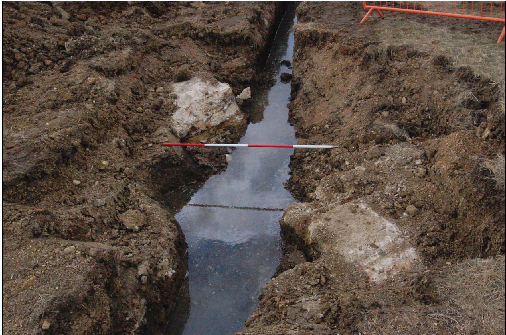
Plate 3. Modern truncation and footings present across development area, 2m scale (facing north).
