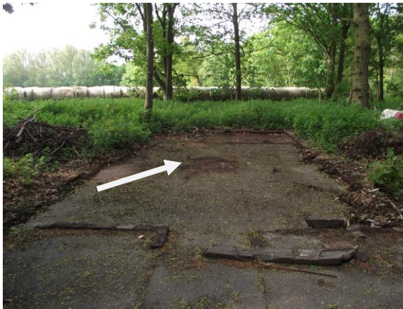
Fig 14 View of Northern section, showing section of vertical support, and internal wall lines. A small vertical pin was discovered (arrowed)
