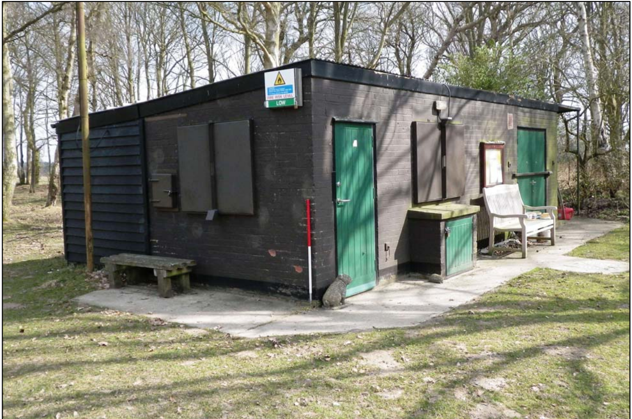
Plate 28. Building 29, camera facing east
