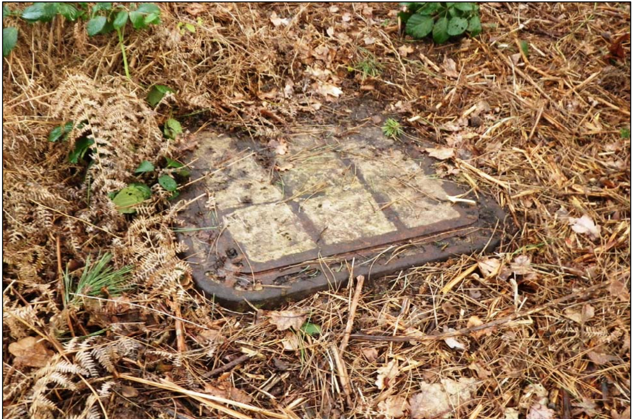
Plate 35. Amphibious Escape Training Facility - manhole cover (IX)
