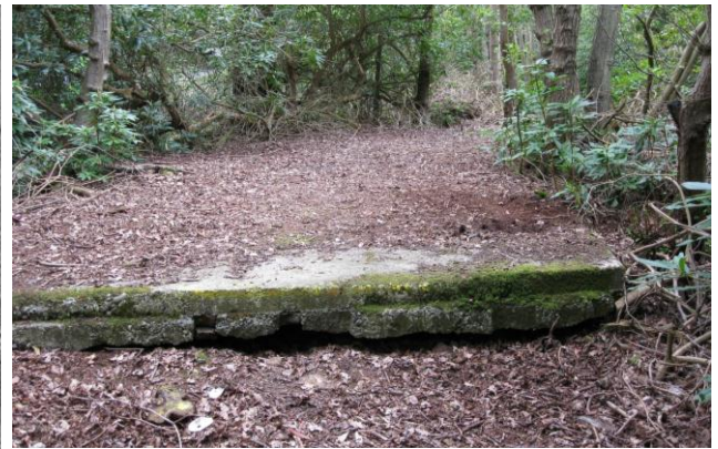
Fig 22 Surviving concrete raft formerly supporting Bailey Bridge at Lound Run
