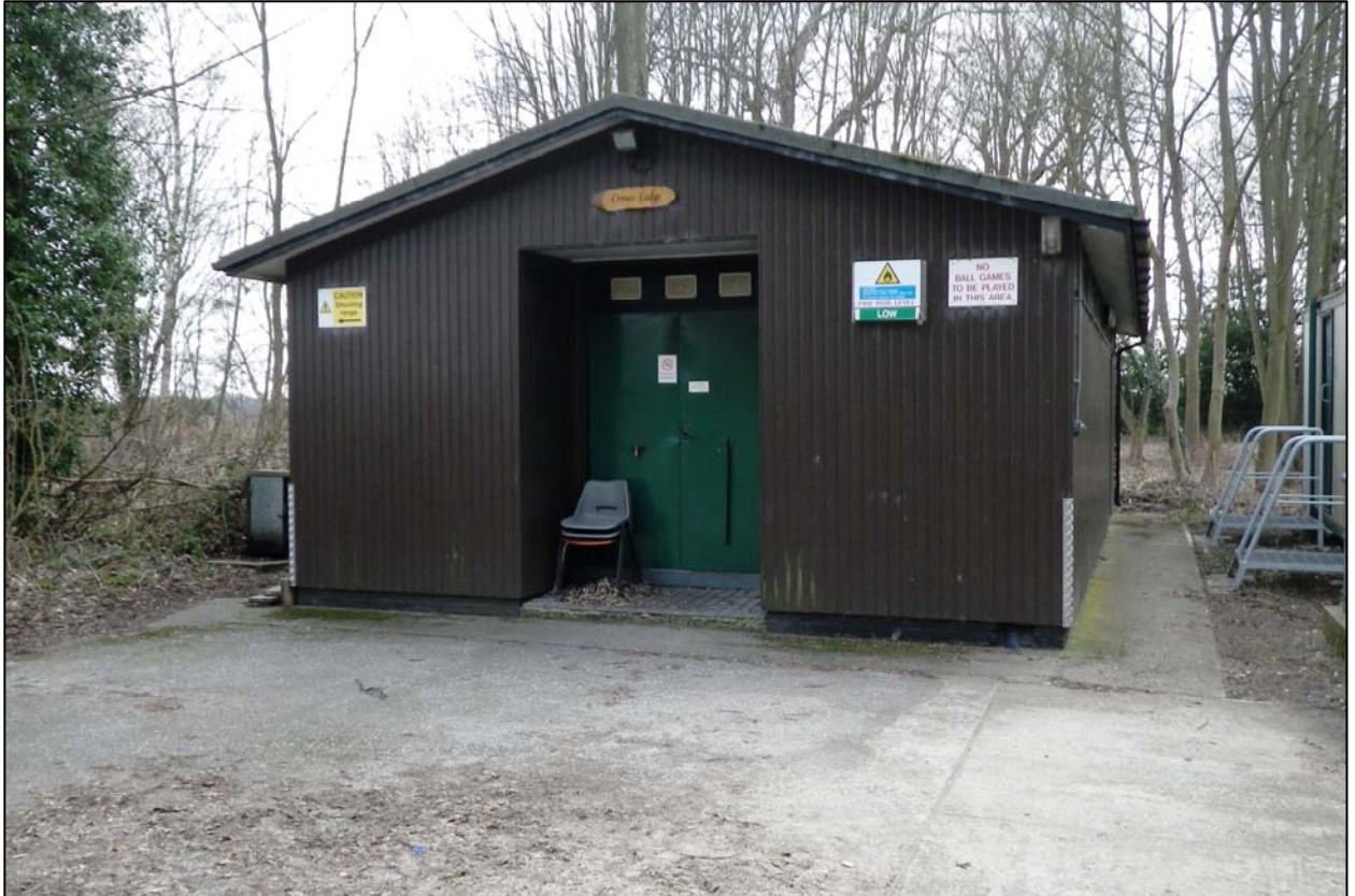
Plate 27. existing scout building (Building 28), camera facing south
