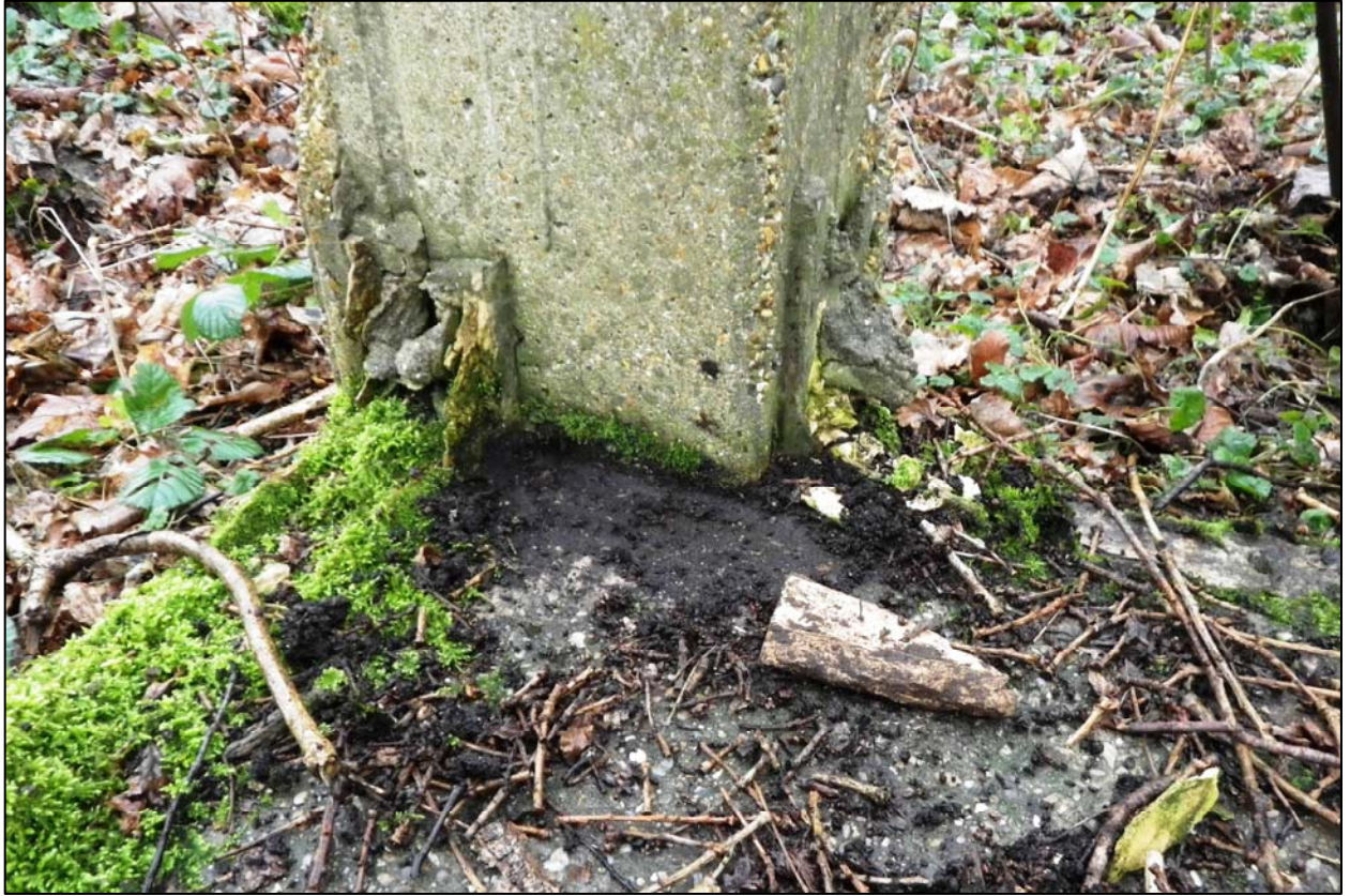
Plate 20. Building 22, upright in the north west corner showing remnants of the hollow ceramic blocks
