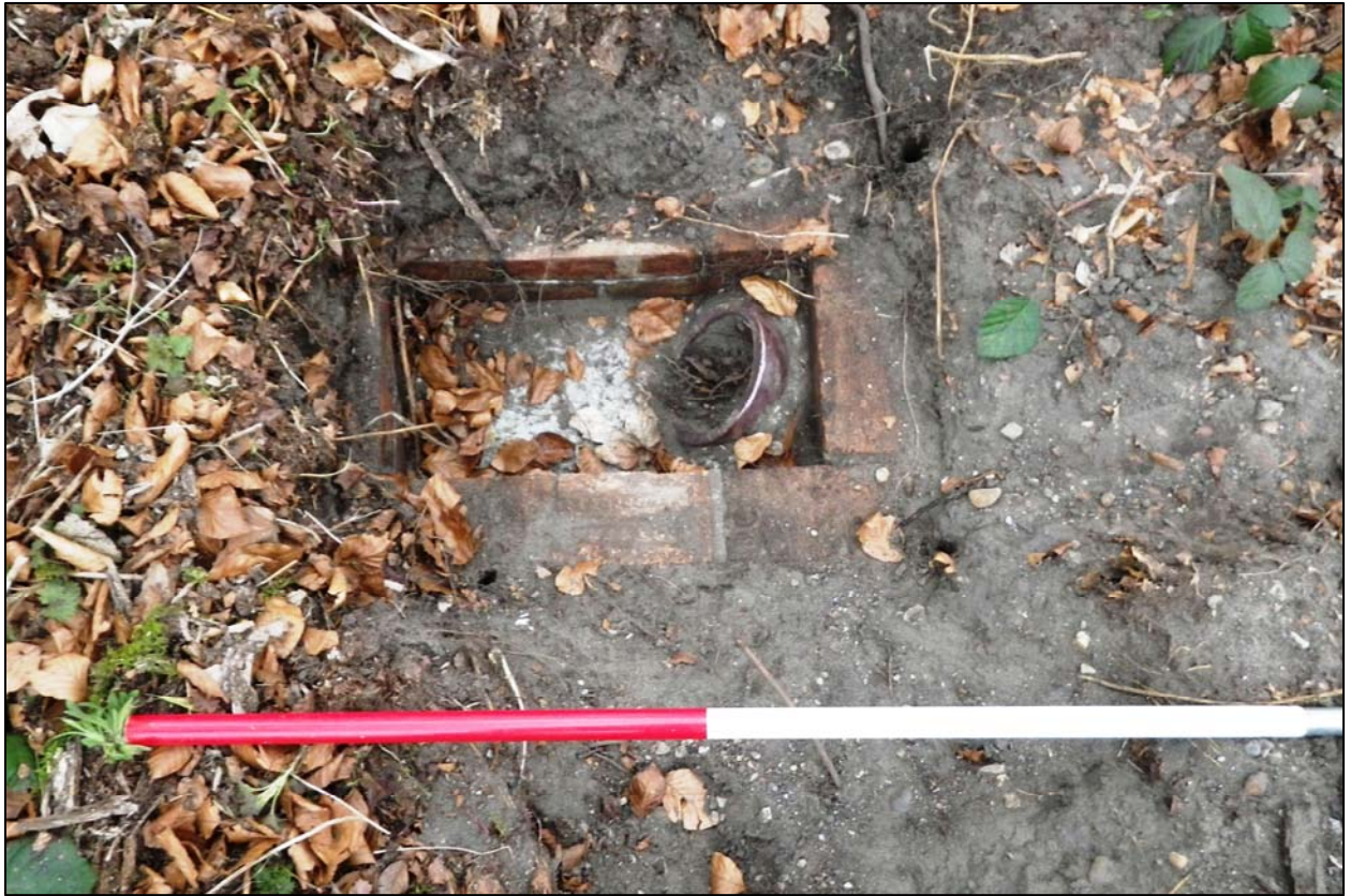
Plate 15. Building 15, drain access point , adjacent to the eastern wall of Building 15
