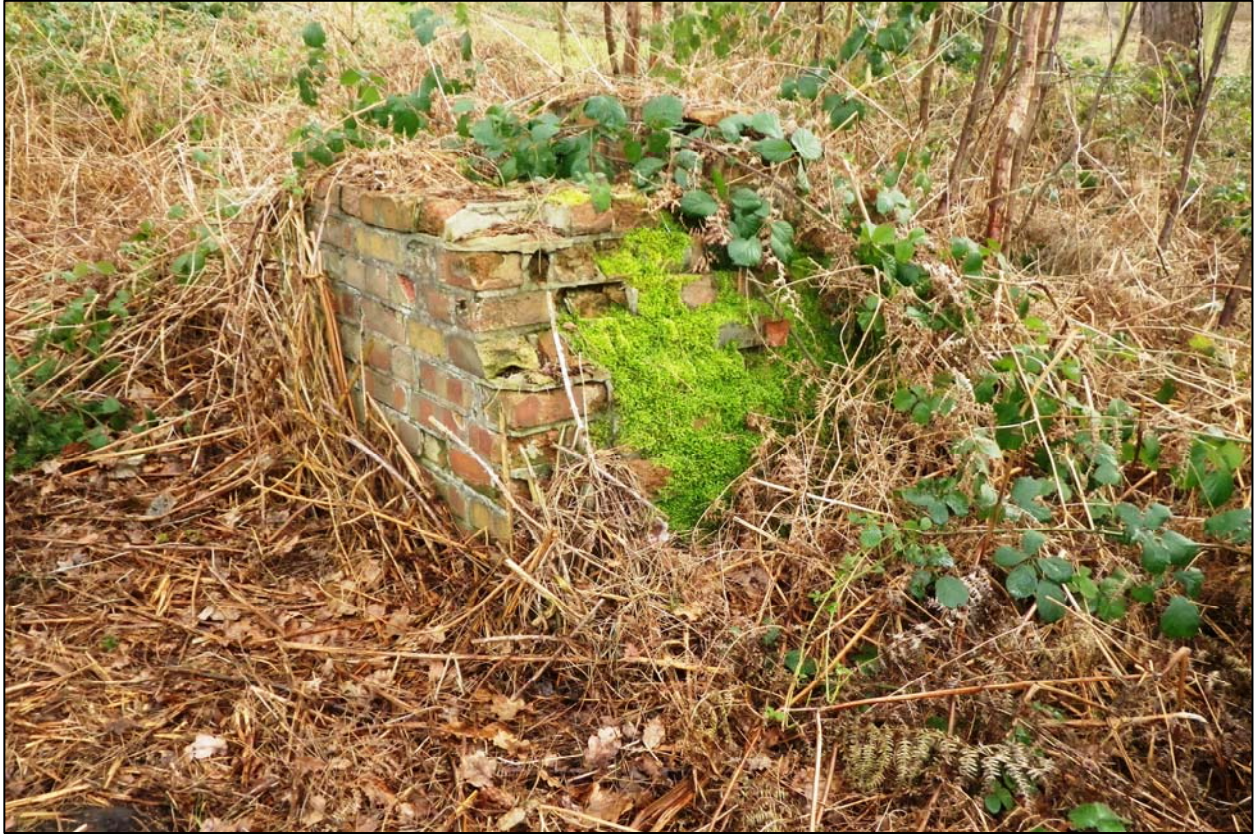
Plate 34. Amphibious Escape Training Facility - exterior of the brick lined shaft (VIII)
