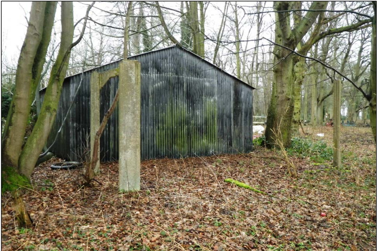
Plate 21. Building 22, camera facing south
