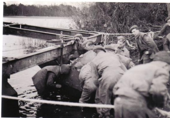
Fig 36 Crews from SADE fitting rudder to Swimming Ark [SEPA 6589/03/12]
