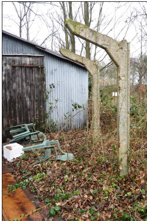
Plate 19. Building 22, showing uprights of former structure, camera facing north west
