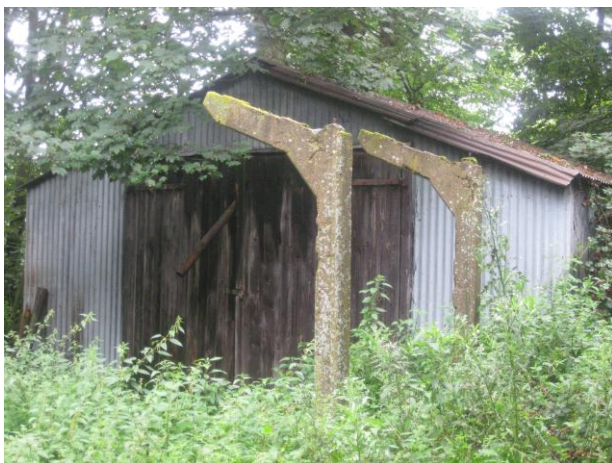
Fig 7 Remains of the Cook House. Some of the original supports have been re used to make the present day corrugated iron shed
