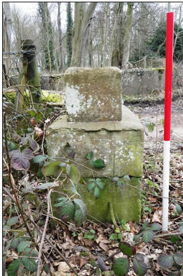
Plate 25. east end of eastern flanking wall (25)
