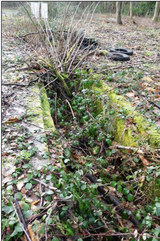
Plate 30. Tank park area - service pit in Building 2
