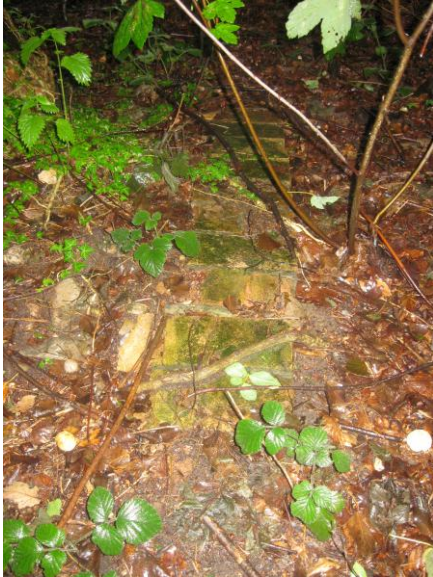
Fig 9 remains of brick footings
