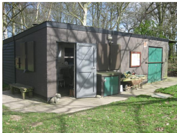
Fig 8 Re-used Military Structure, used to formerly house a machine, assumed to be the site of the Generator
