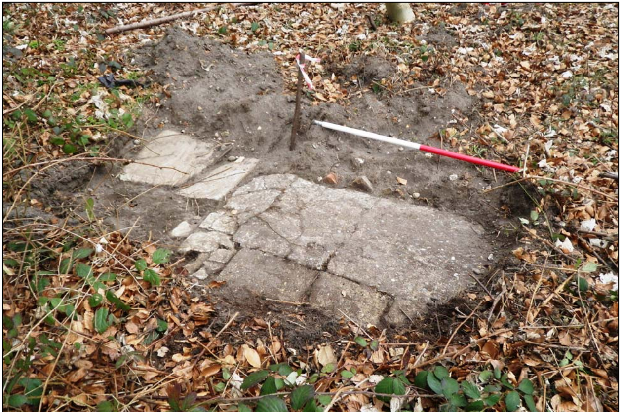
Plate 12. Building 13, south east corner showing floor slab and external paving slab
