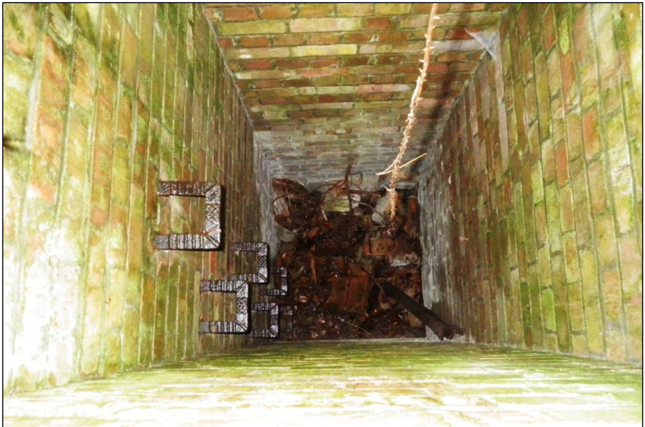
Plate 33. Amphibious Escape Training Facility - view down brick lined shaft (VIII)
