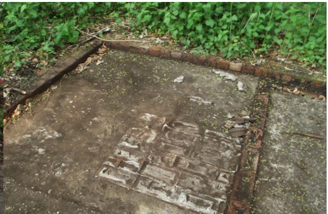
Fig 15 View of Foundations for Water tank (far side – circular) and 78cm square base for an additional structure.
