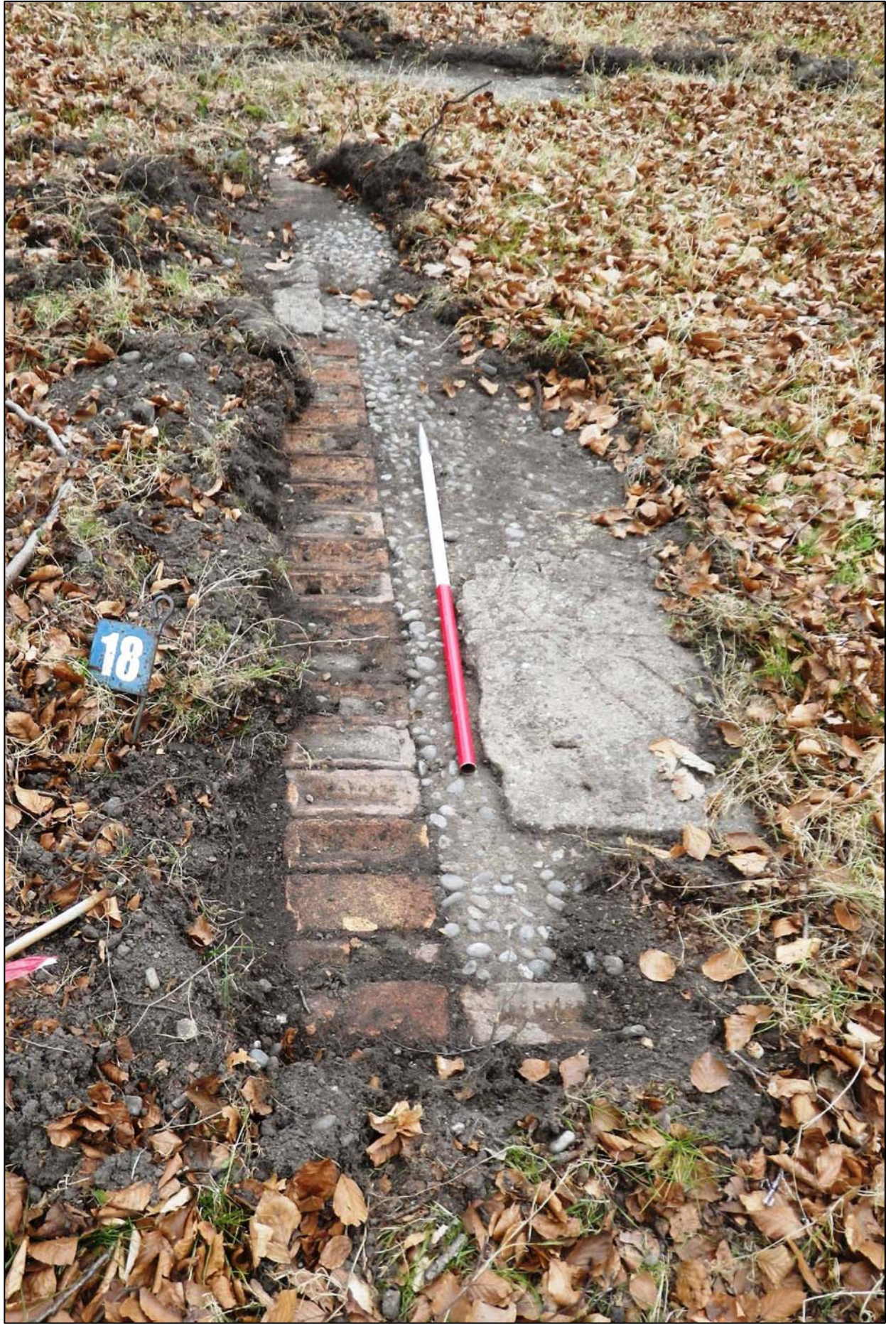
Plate 17. Building 18, western end of structure
