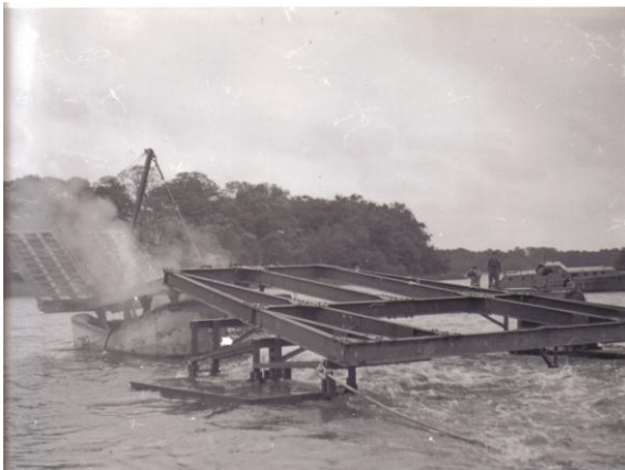
Fig 23 Trails associated with the Swimming Ark or Hopper in 1945, enabled other DDs to climb over it, out of steep sided canals. SEP 6680/31
