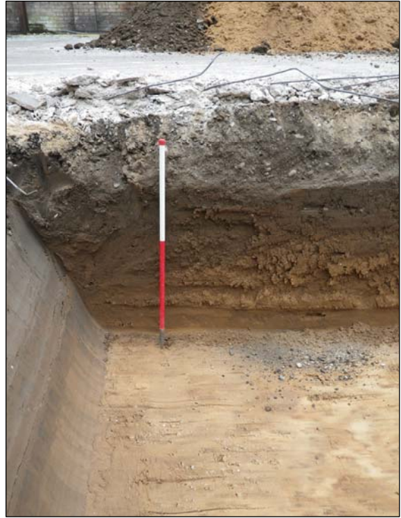
Plate 2. Trench 1, soil profile
