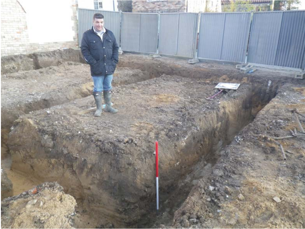
Plot 2 looking south-east. Scale bars at 0.5m
