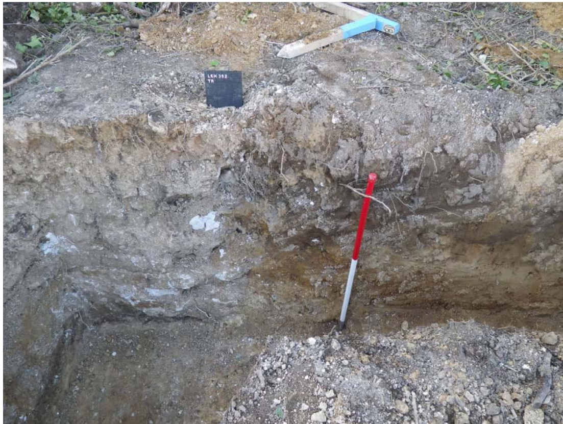
Plate 12. Section 5, north-west face of cellar 0028 showing clunch walling. Scale bar at 0.5m
