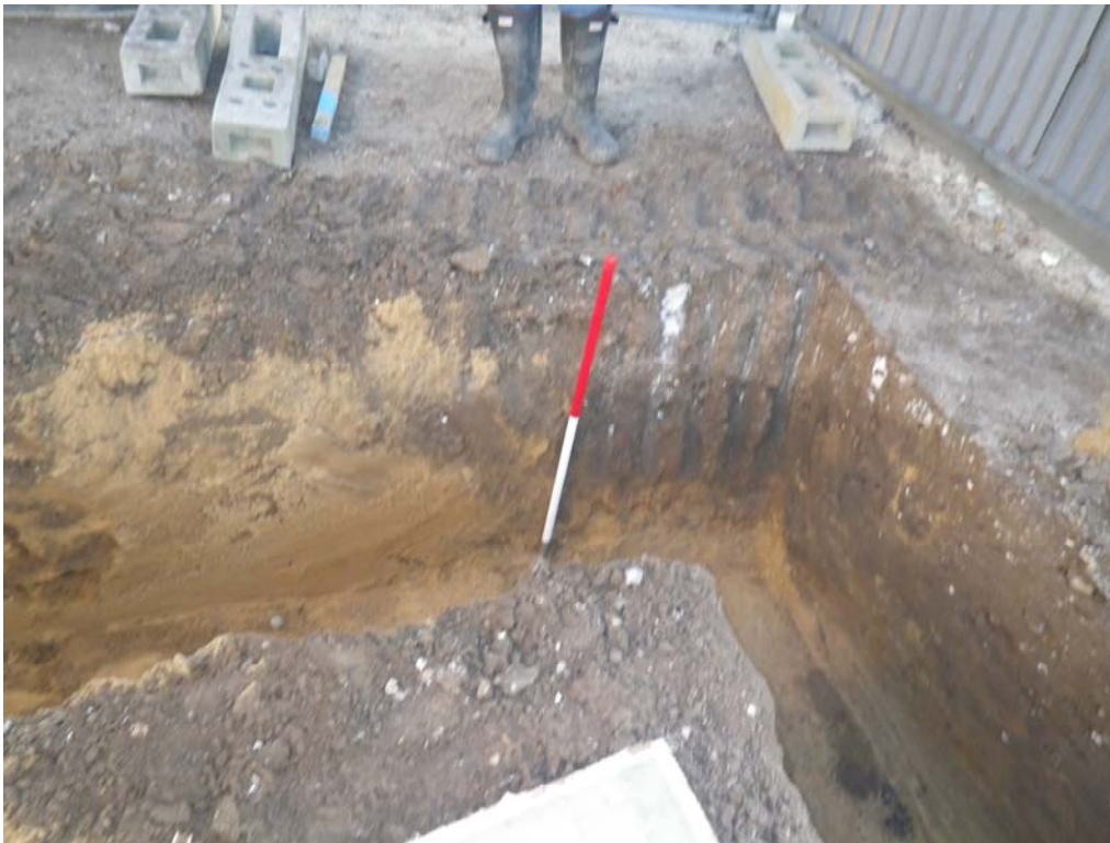
Plot 2 south-west corner. Scale bars at 0.5m
