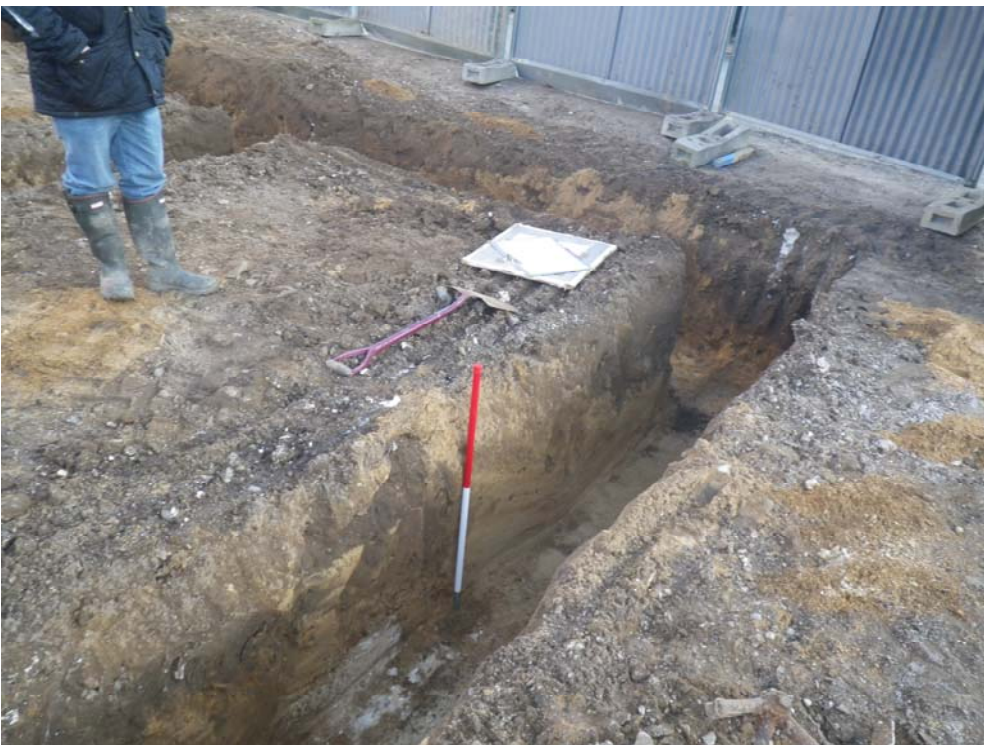
Plot 2 south-west corner, looking south. Scale bars at 0.5m
