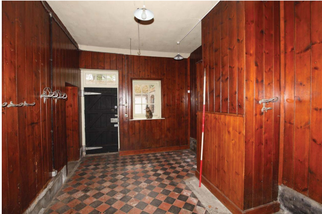
Illus. 13. The interior of the tack room extension from the north showing its boarded walls with modern tack hooks and a blocked gable fireplace to the right.
