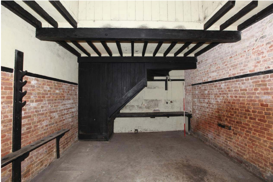
Illus. 11. The loft stair against the rear (northern) wall of the central coach house with its tack hooks and holes to the left. The projections of the ceiling at top-right and top-left provided access to the secondary doors between the attic over the coach house and the lofts of the two stables.
