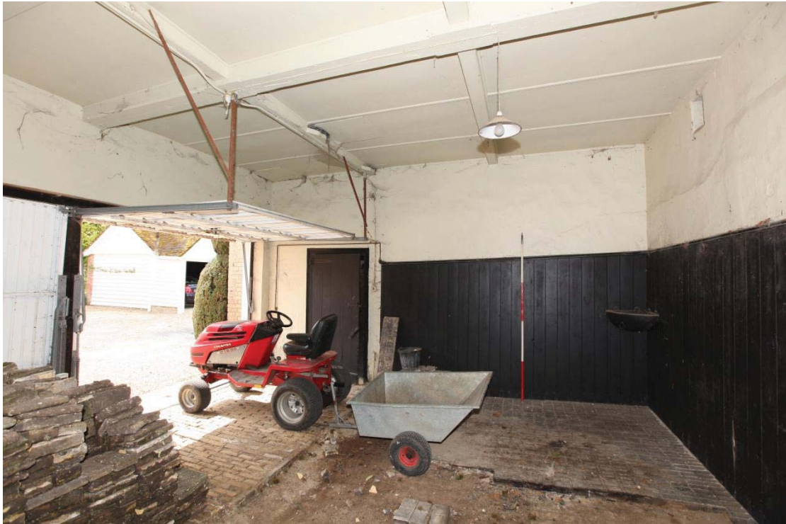
Illus. 9. The interior of the garage from the east showing the remaining wainscot boarding and corner manger of two loose boxes matching those of the western stable, with the floor bricks of its southern passage to the left. The scars of two earlier stall partitions can be seen in the plaster of the rear wall to the right.
