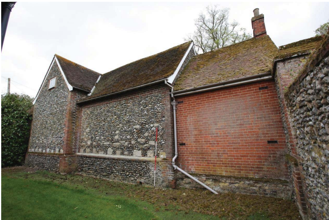
Illus. 6. The rear elevation of the building from the north-west, showing the later brick tack room on the right. The flint-rubble walls of the original structure are dressed in red brick to the rear (as opposed to gault brick to the south) and contain re-used blocks of dressed medieval stone that may have been salvaged when the parish church was rebuilt in 1854.
