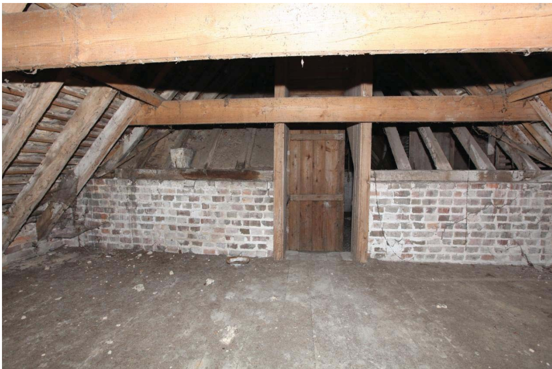
Illus. 16. The eastern loft above the garage, viewed from the east and showing the inserted doorway to the attic of the coach house; the door's pine jambs interrupt the original brickwork.
