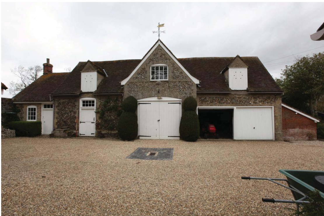
Illus. 4. The southern facade of the coach house and stables showing the lower roof of the tack room extension to the left and the lean-to brick log store on the right. The original building was symmetrical with two stables and lofts flanking the central gable of the coach house. The eastern stable on the right was converted into a garage during the 20 th century but evidence of its original central door can still be seen.
