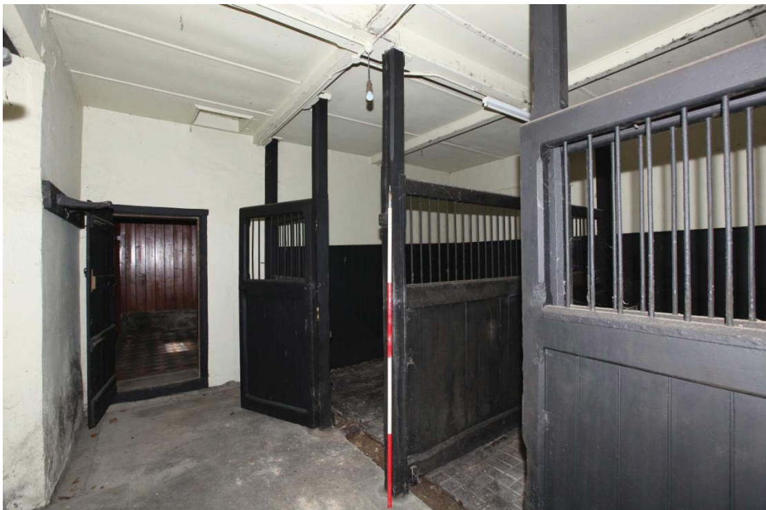
Illus. 12. The western stable seen from the east showing the well-made doors and partitions of its two loose boxes, all with neatly chamfered timber and pegged joints. The boxes probably date from the end of the 19 th century and are impressive survivals, but replaced three earlier stalls as indicated by the scars of their partitions on the back wall. The door on the left open into the tack room extension.
