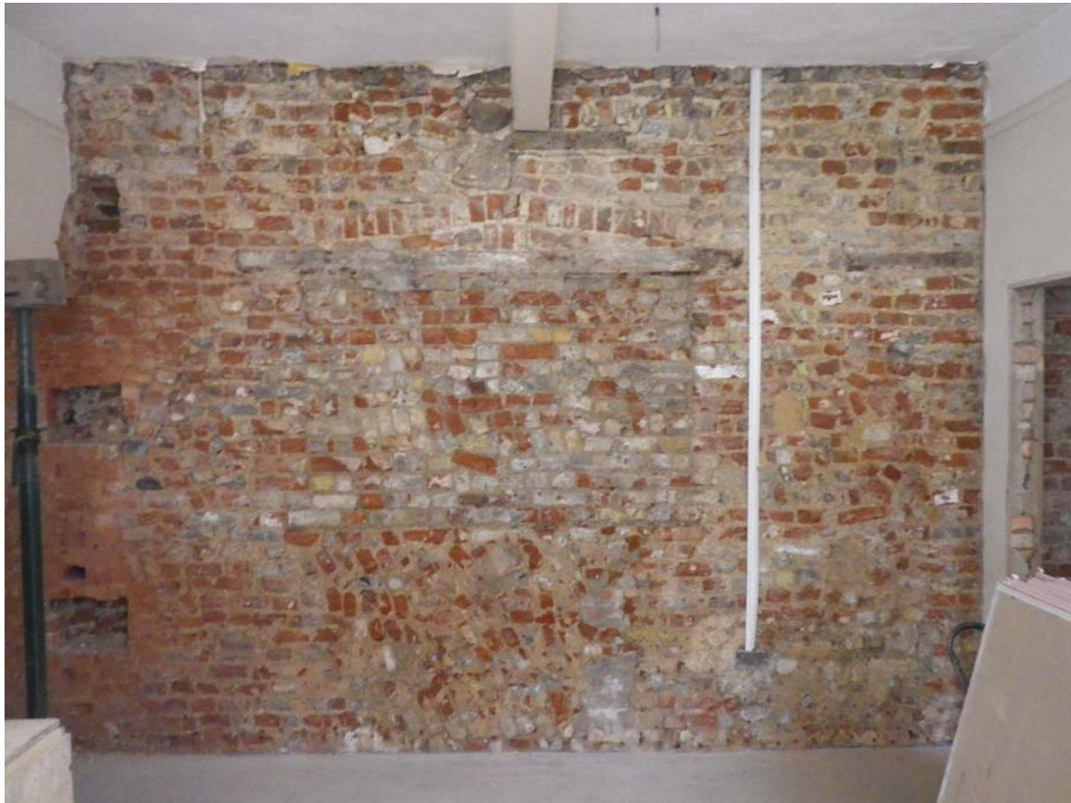
Plate 2. Wall 0010 showing blocked up double window with softwood lintel, facing north
