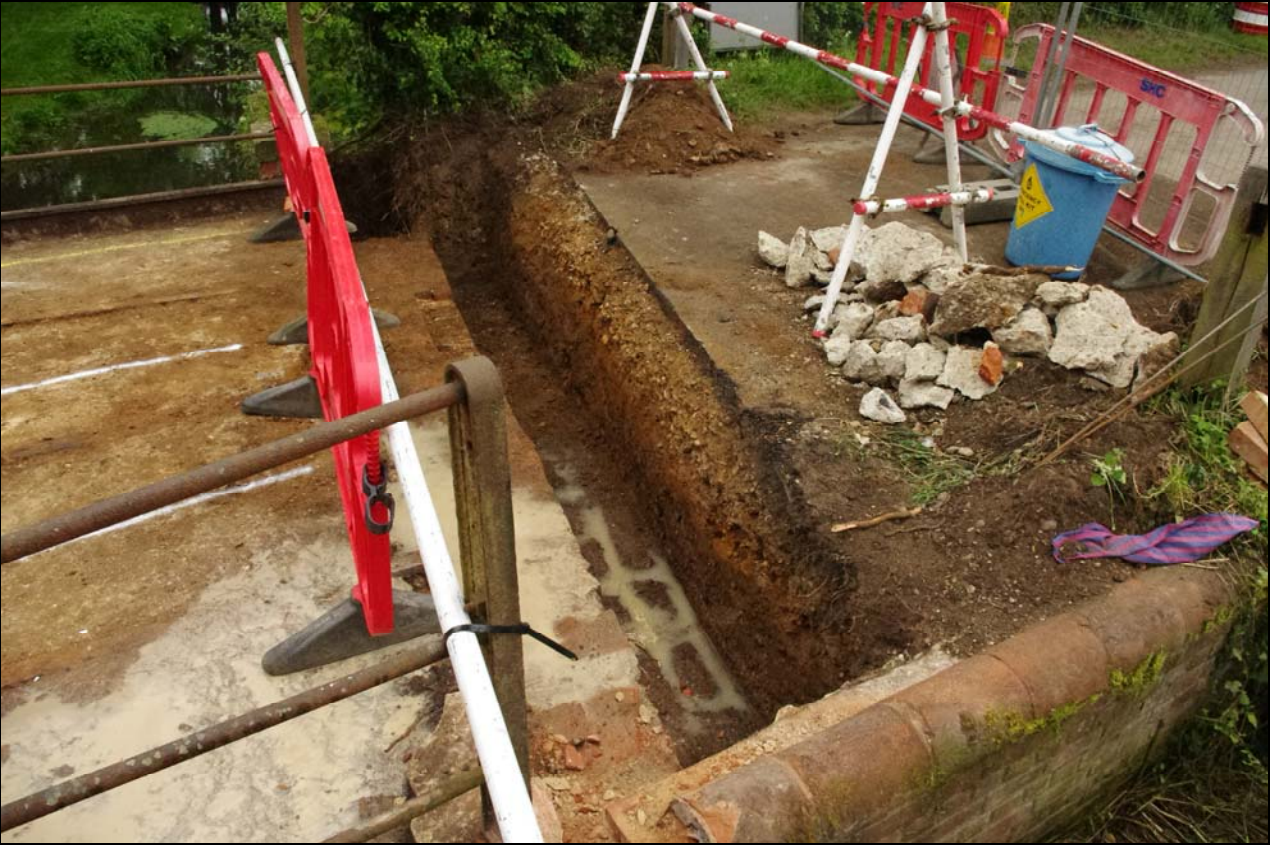
Plate 2. Trench 2 and newly exposed brickwork running behind brick piers, facing north
