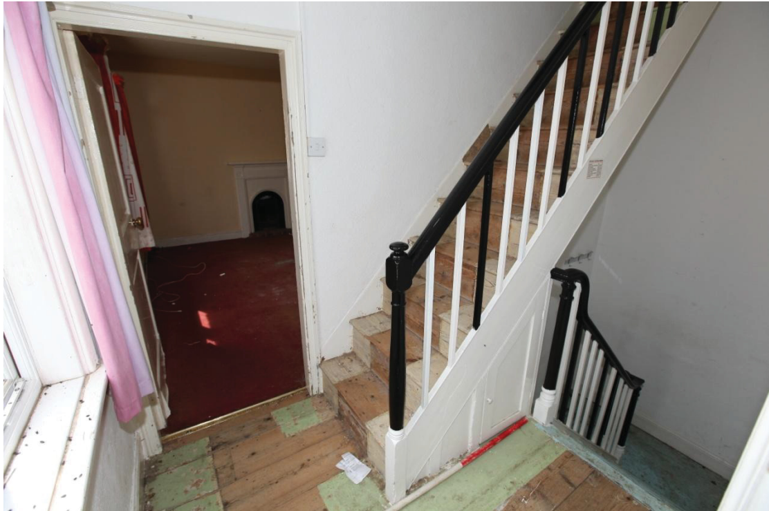
Illus. 15. The second landing of the original central stair in the dwelling house seen from the east. The stair descends to the entrance lobby on the right (illus. 12) and rises to the attic rooms. The bedroom to the west (left) contains an arched late Victorian coal grate and is linked to the kitchen of a modern flat, both of which lie above the ground-floor WC.
