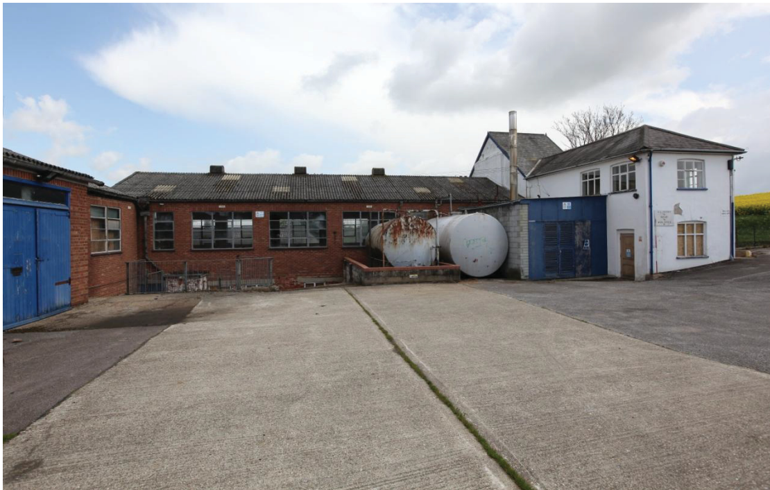
Illus. 2. The exterior of the red-brick dye house from the site of the 19 th century headwater pond to the west (now a car park) showing the high gable of the manager's house on the right and the 1960s sheds to the left. The dye house retains only the basement storey of the three-storey 19 th century mill, which continued the roof of the manager's house, and in its present form dates only from 1961.
