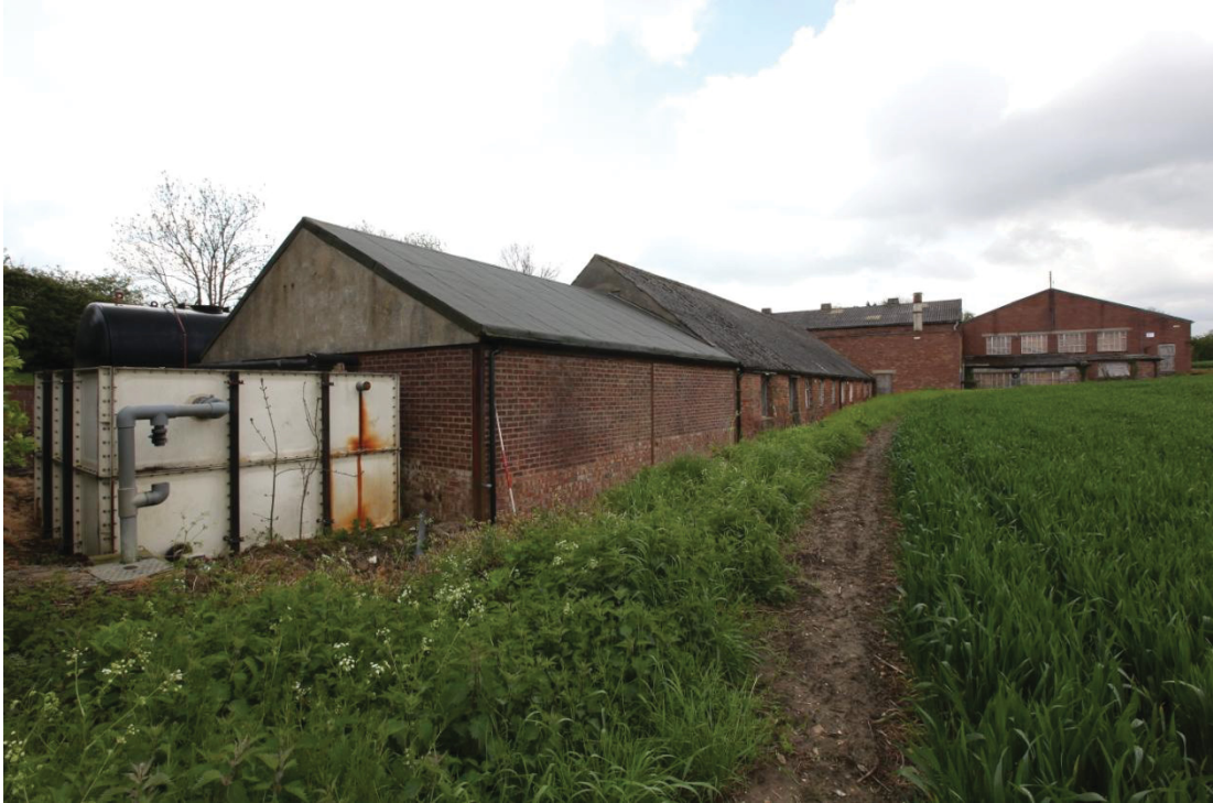
Illus. 5. The complex from the north-east. The long, single-storied 19 th century red-brick shed that latterly operated as the dye and yarn store lies in the centre with its lower 20 th century extension on the left, the mid-20 th century ‘old boiler room’ with its chimney in the centre and the 1960s sheds on the right.
