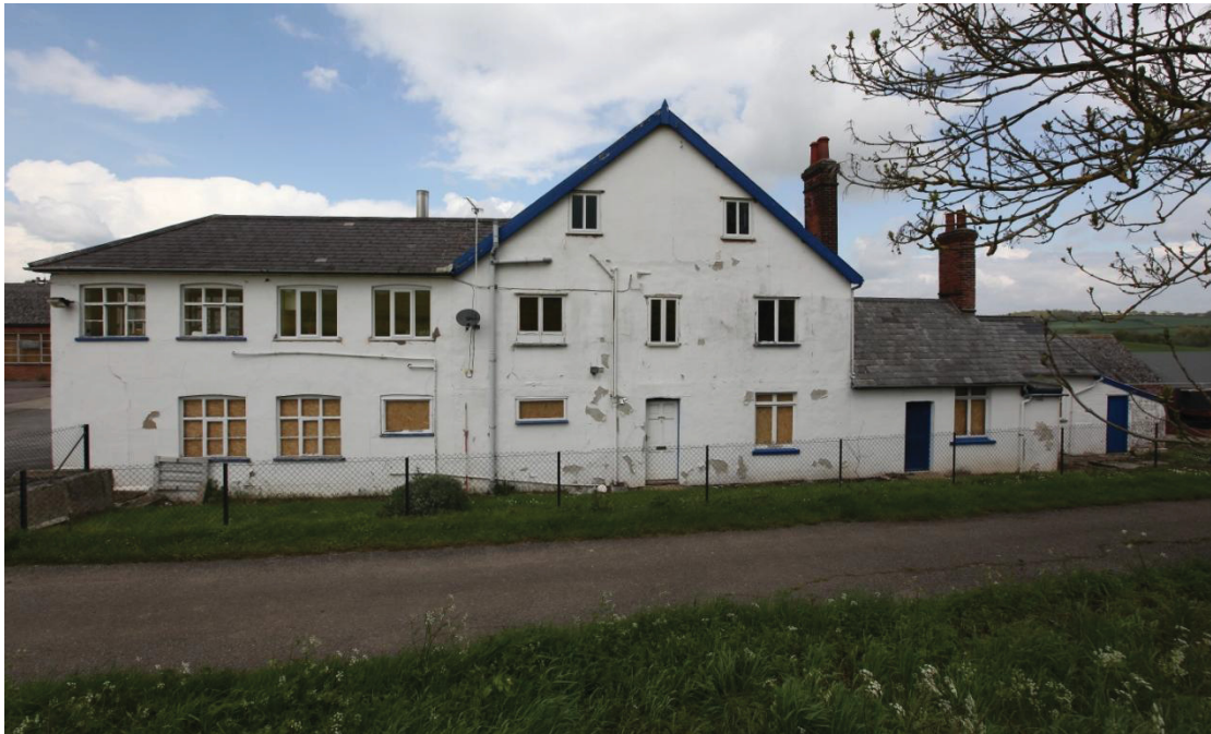
Illus. 1. The southern facade of the mill showing the wide gable of the original manager's house in the centre with its single-storied kitchen (most recently used as a lab) to the right and the later canteen wing to the left. The chimney to the right of the house was formerly matched by another to the left, and its fenestration was entirely renewed in the mid-20 th century.
