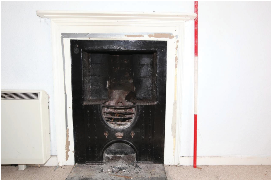
Illus. 16. A detail of the late Georgian swan's nest coal grate in the eastern gable of the first-floor bedroom above the office. This is typical of the 1820s and is likely to be original to the 1824 mill.
