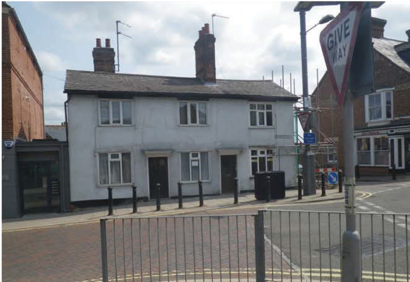
The front of Nos. 85 and 87 High Street viewed from the south. No 87 is to the left and the double fronted door cases are original and suggest an early 19th century date. The windows and slate roof are thought to be later replacements.
