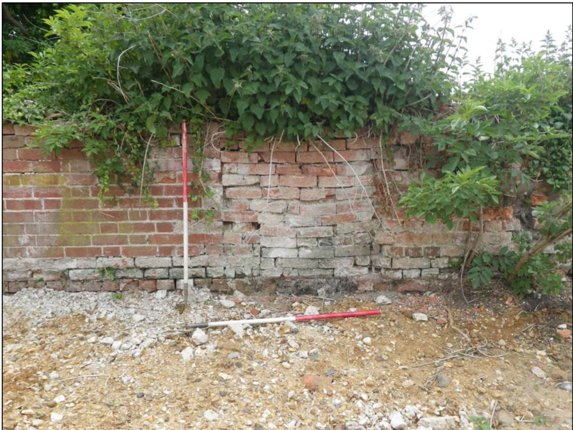
Plate 8. Trench 3, blocked doorway
