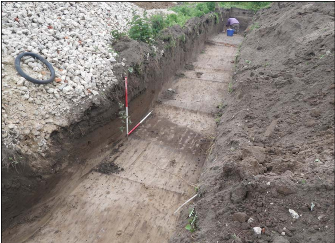
Plate 6. Trench 3, Ditch 0006 (note the large crushed concrete heap close to the edge of the trench)
