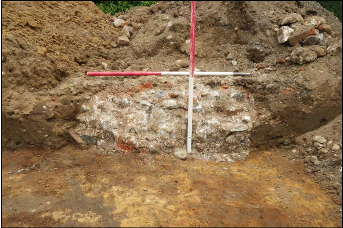
Plate 3. Trench 2, section across the tower mill foundation (0012) (Section 2)
