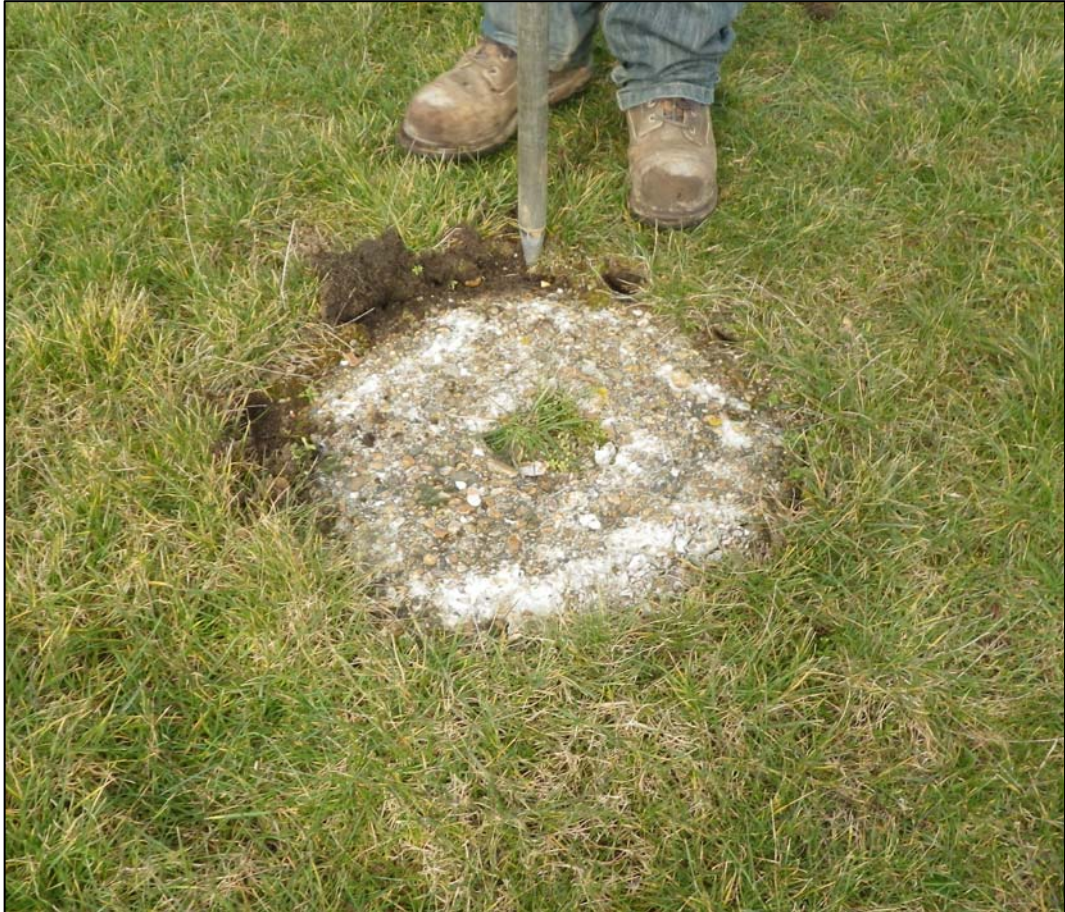
Plate 33. concrete filled post setting (0071)
