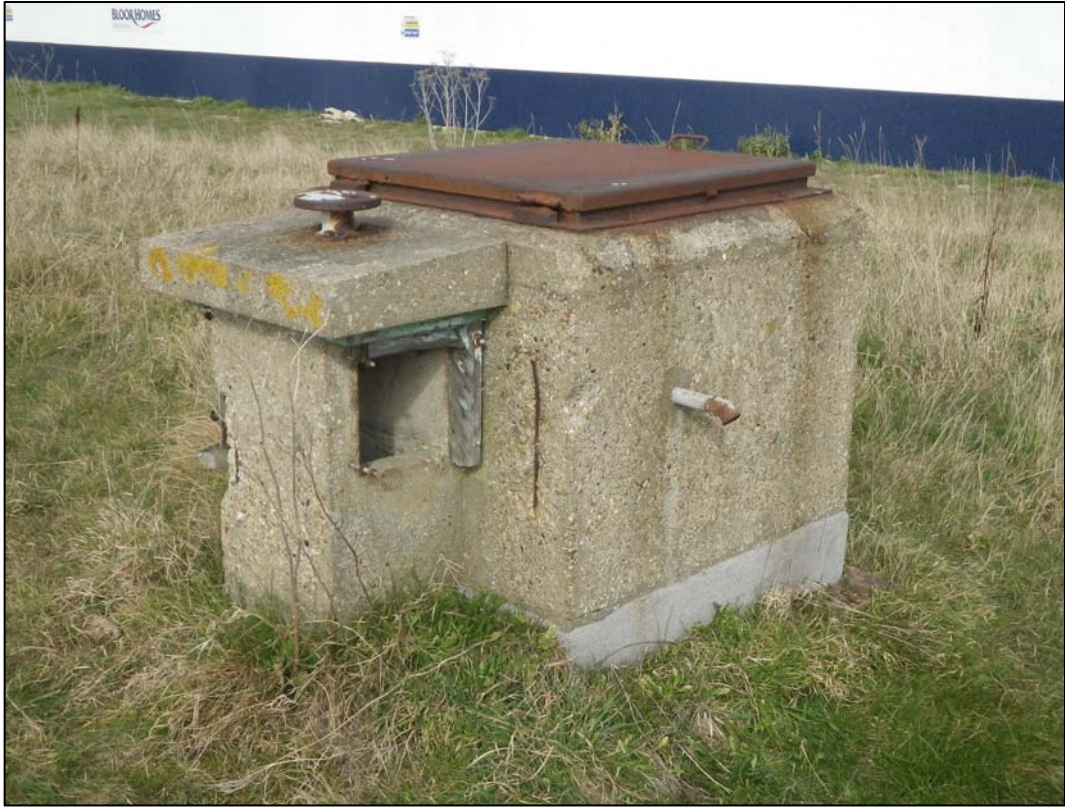
Plate 27. ROC post - entrance hatch and vent (0067)
