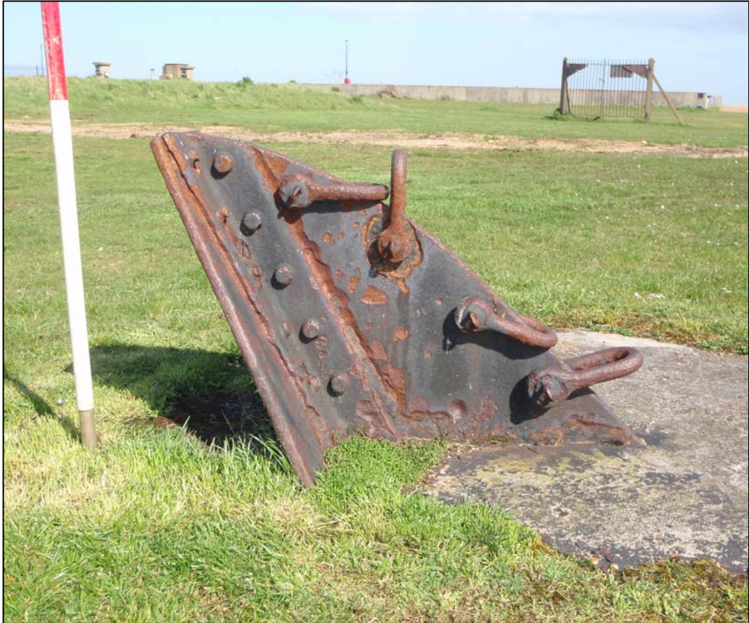
Plate 11. Anchor block (0053) showing steel plate bracket
