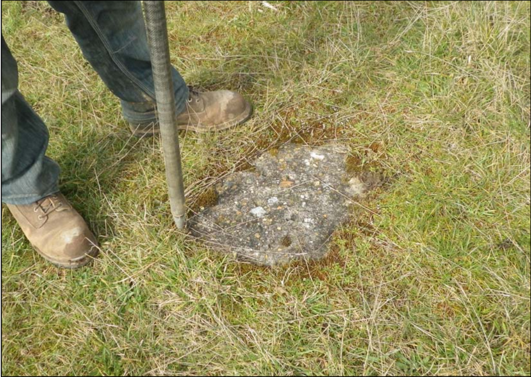
Plate 35. concrete slab, probable anchor block (0073)
