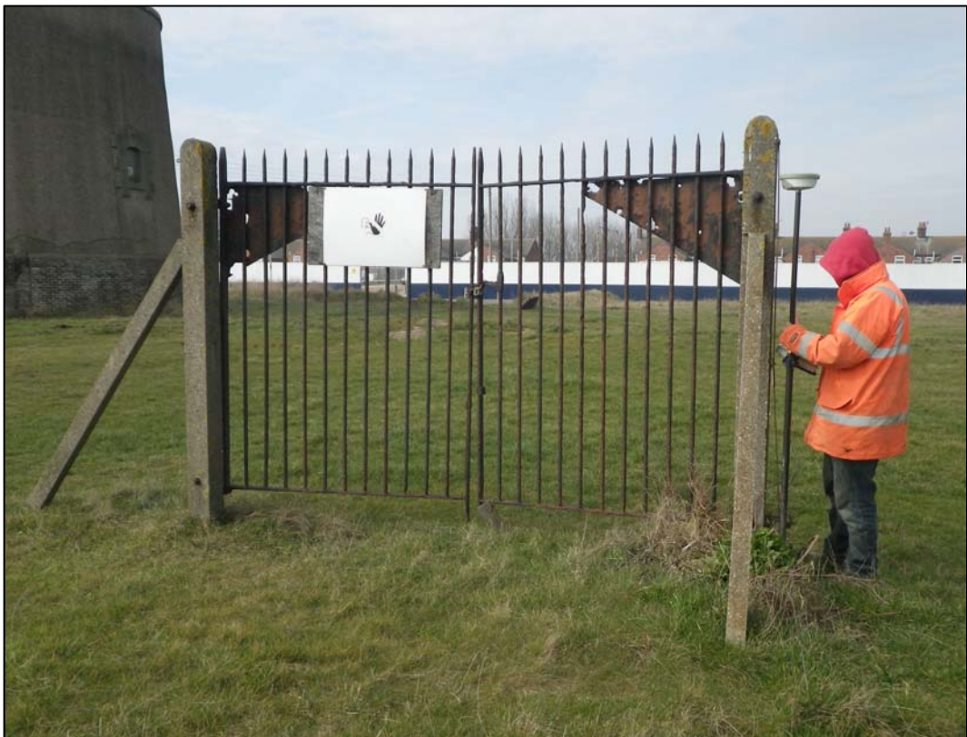
Plate 28. Pair of iron railing gates (0068)
