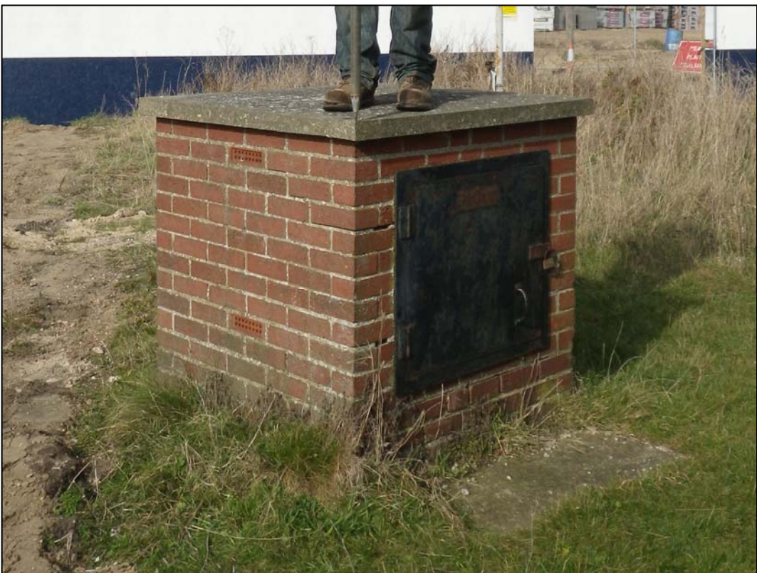
Plate 32. Brick built box or cabinet (0070)
