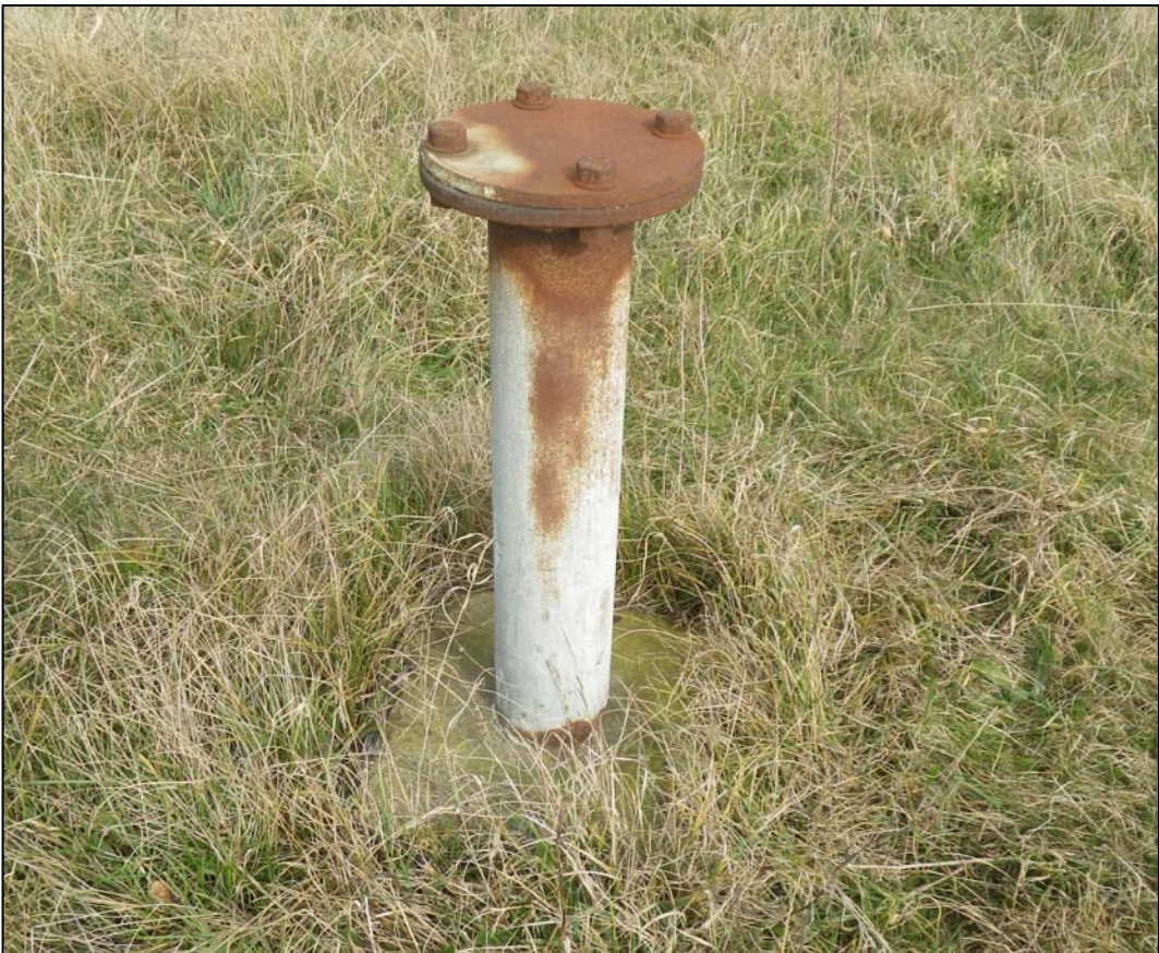
Plate 26. ROC post - mounting for a fixed survey probe (0066)
