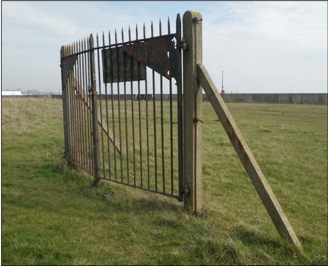
Plate 29. Pair of iron railing gates (0068)
