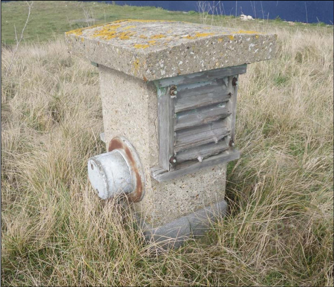
Plate 25. ROC post - main vent (0065)
