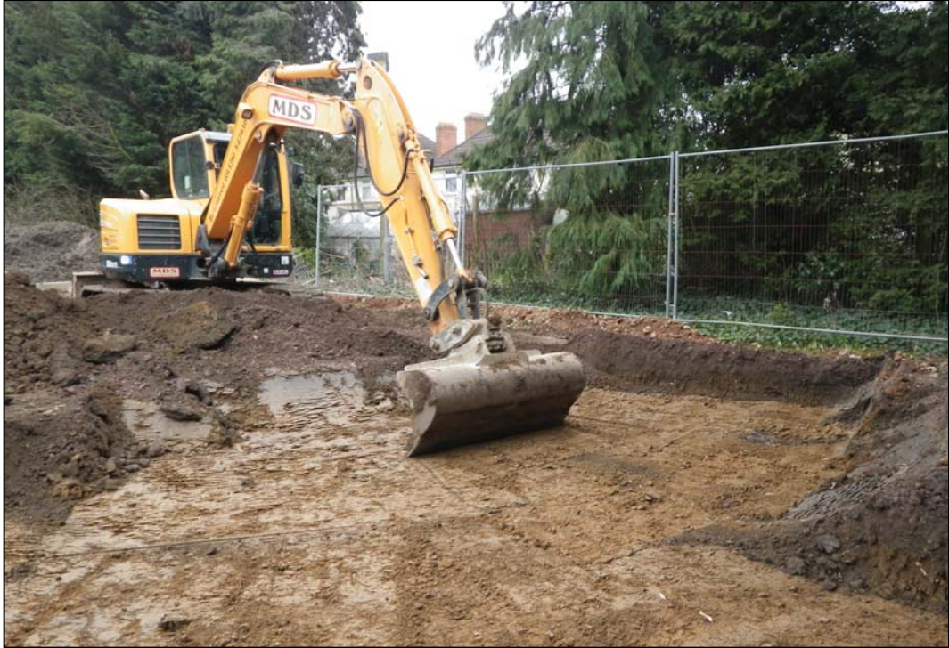
Plate 1. topsoil stripping of the excavation area (ref. HTO 60)
