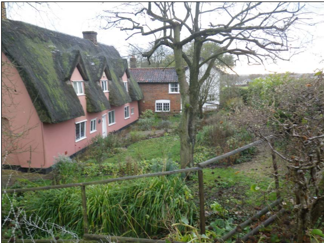
Plate 1 Looking south down onto Cherry tree Cottage
