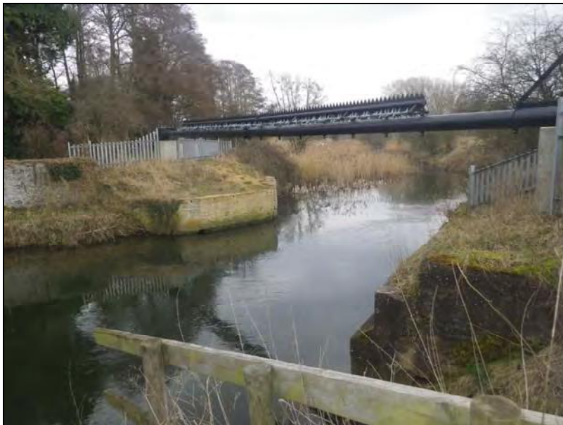
Photo 7. Temple Bridge (IKL 117)
