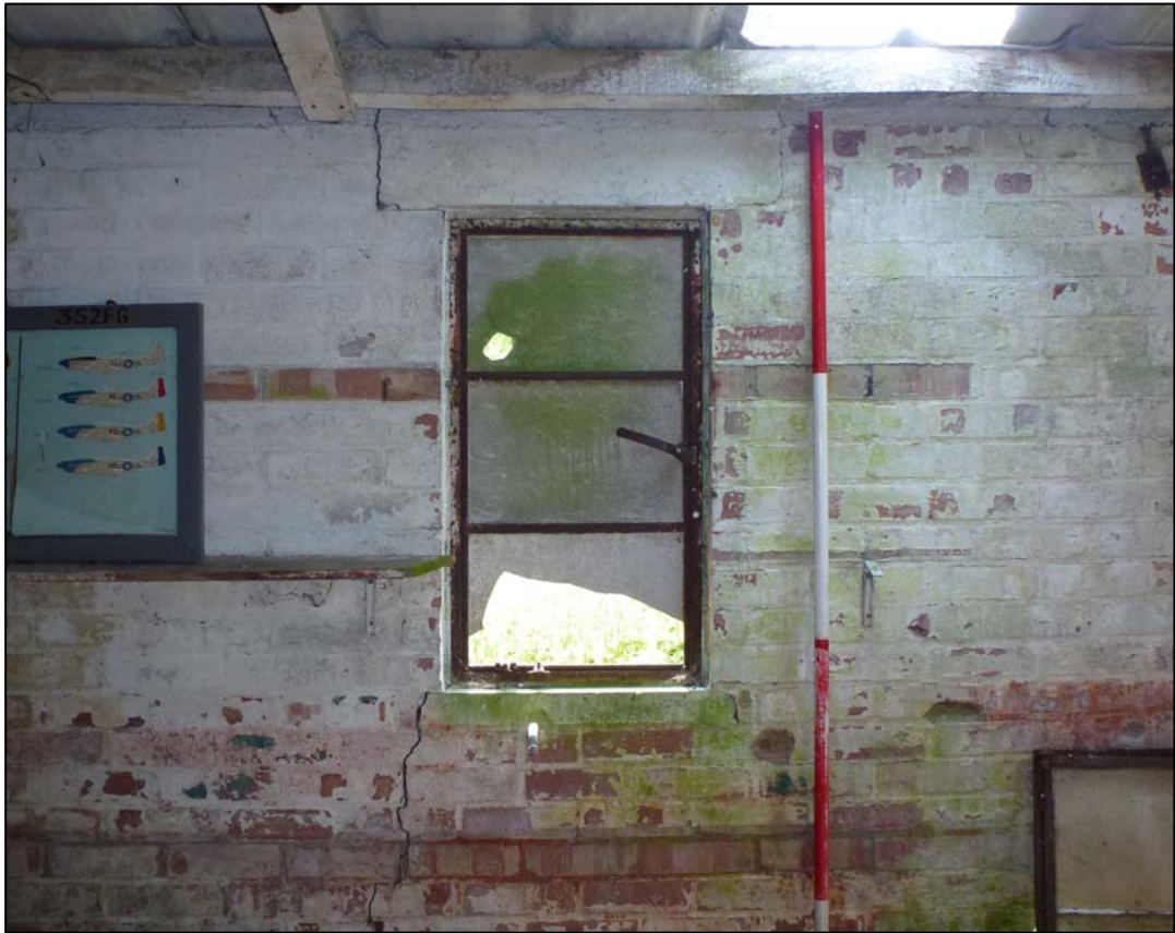
Plate 13. typical window frame, internal view (ref. HTR 23)
