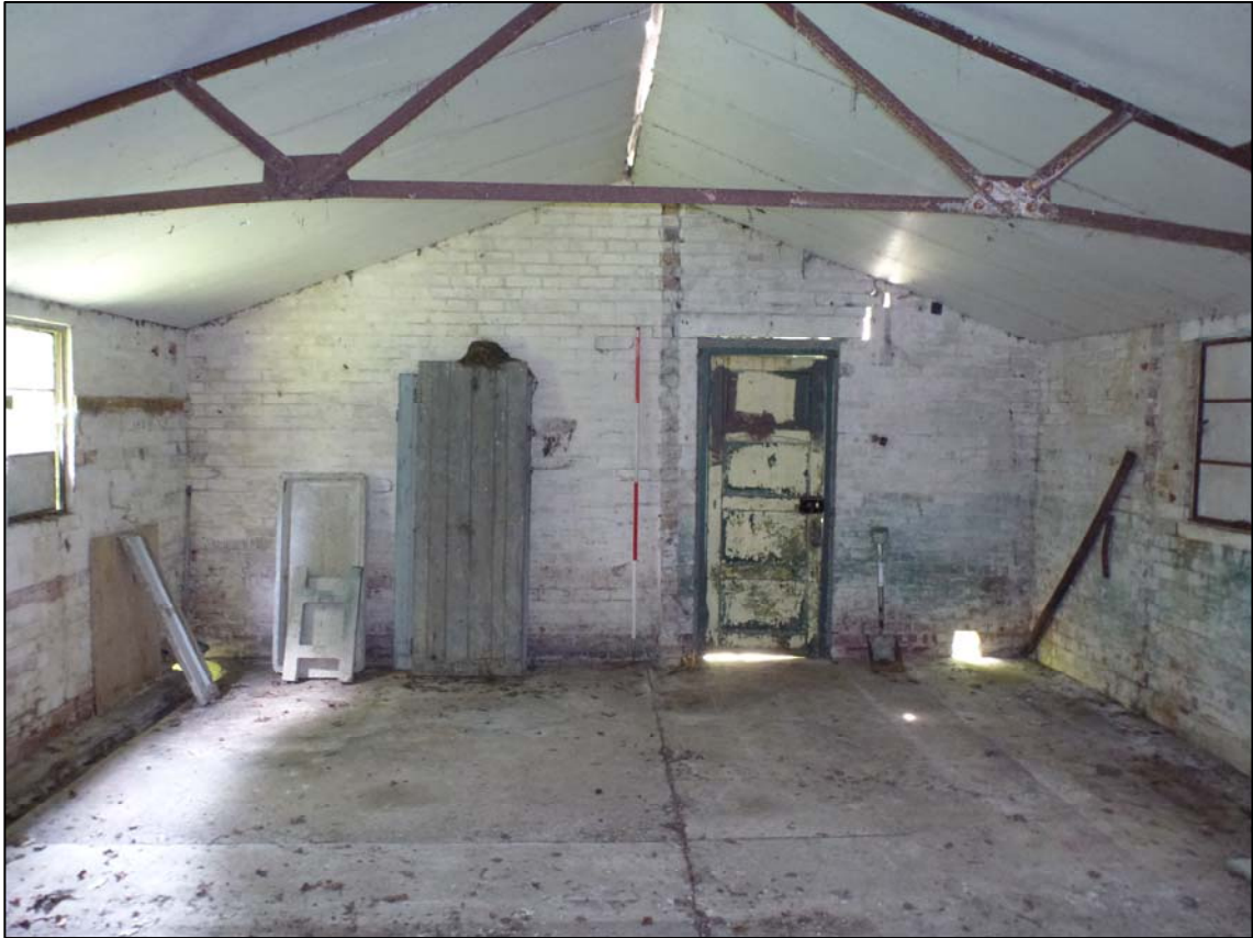
Plate 18. Building 1, Room 1, camera facing south (ref. HTR 05)
