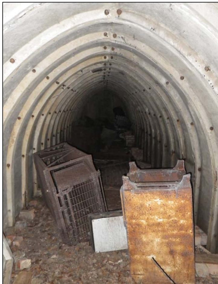
Plate 42. Shelter 2, internal view towards the rear wall (ref. HTR 50)
