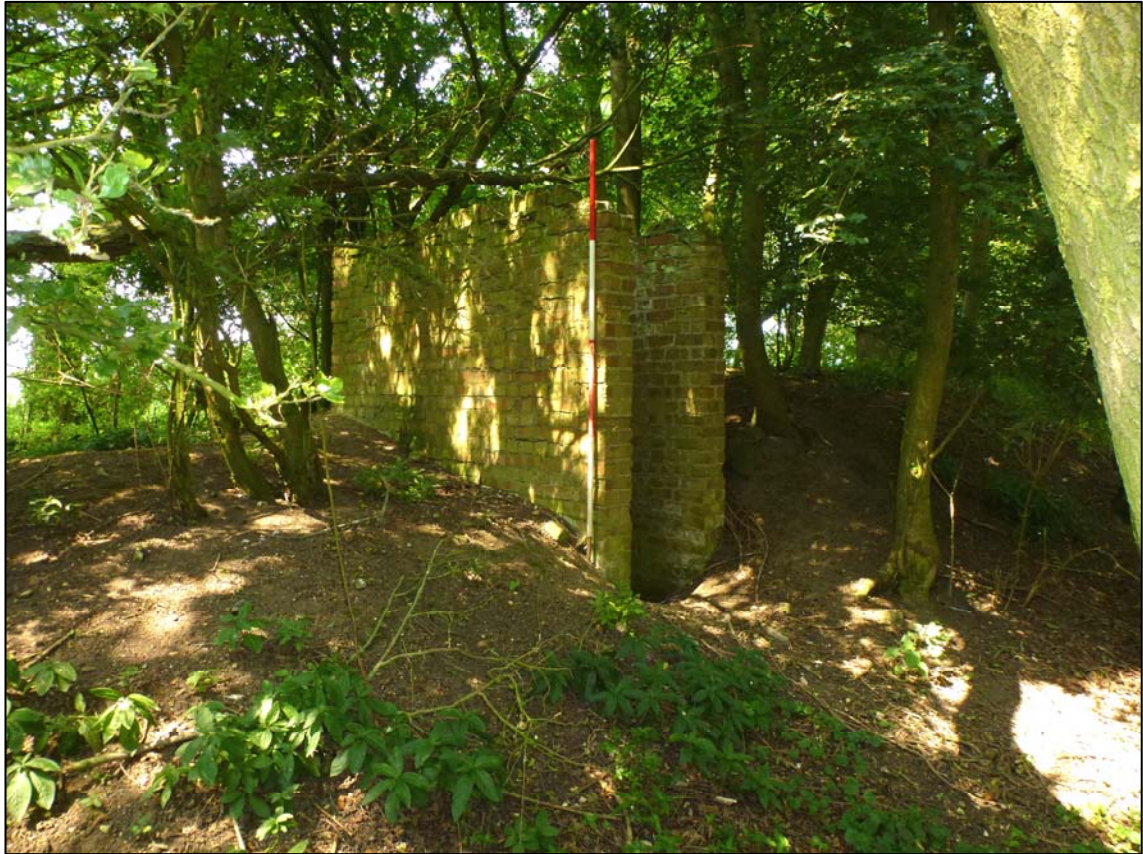
Plate 37. Shelter 1 showing the brick lined entrance (ref. HTR 44)
