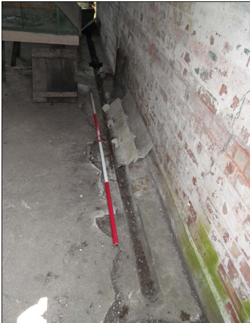
Plate 33. Building 2, drain in Room 2a (ref. HTR 17)
