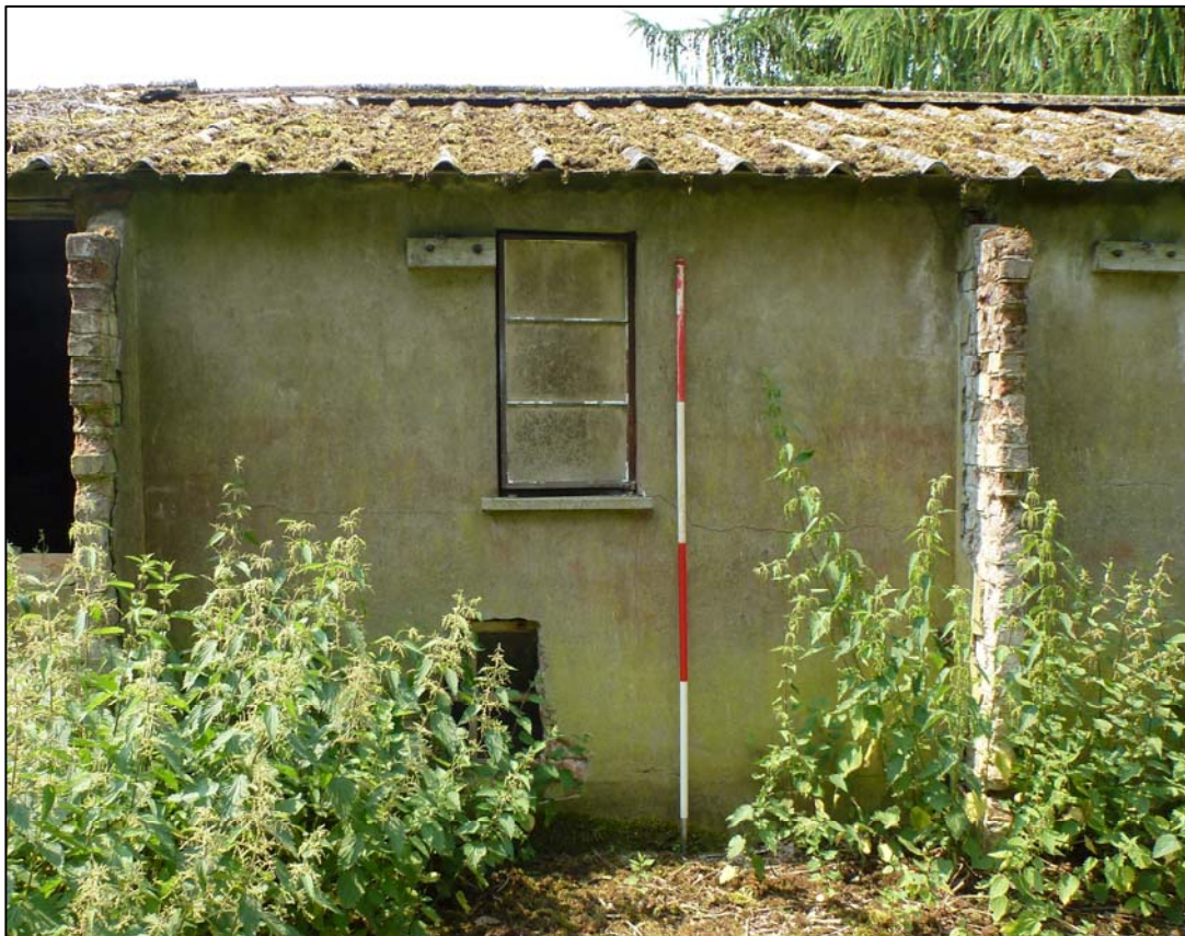
Plate 14. typical window frame, external view (ref. HTQ 18)
