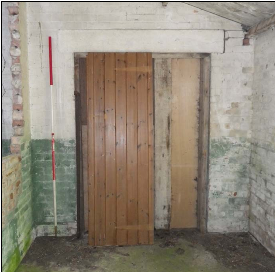
Plate 21. Building 1, Room 2, blocked opening to Room 1 (ref. HTQ 80)
