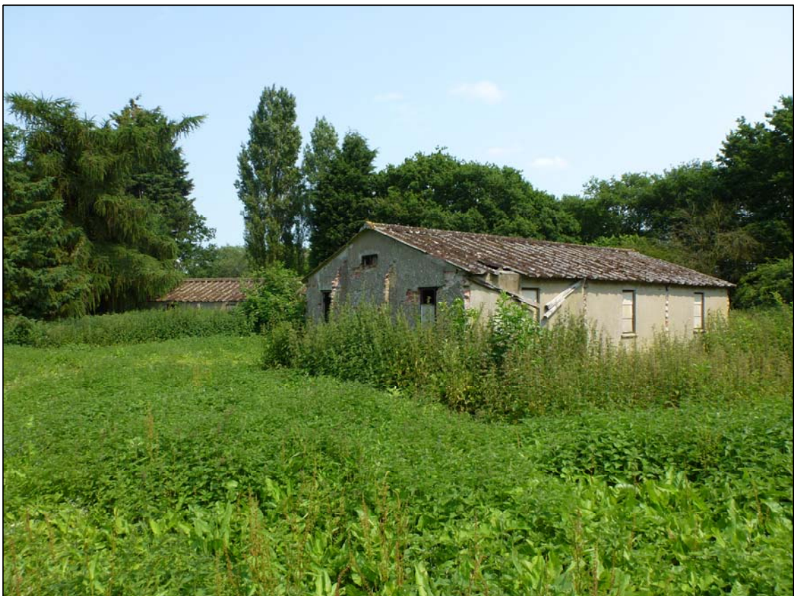
Plate 8. Building 2 (right) with Building 1 (background) -camera facing east (ref. HTQ 09)
