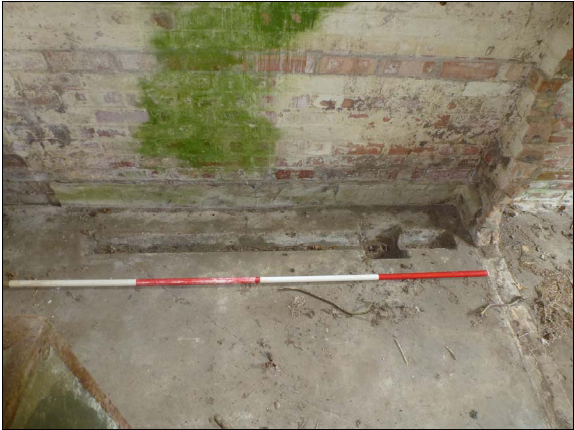
Plate 34. Building 2, drain in Room 2b (ref. HTR 24)
