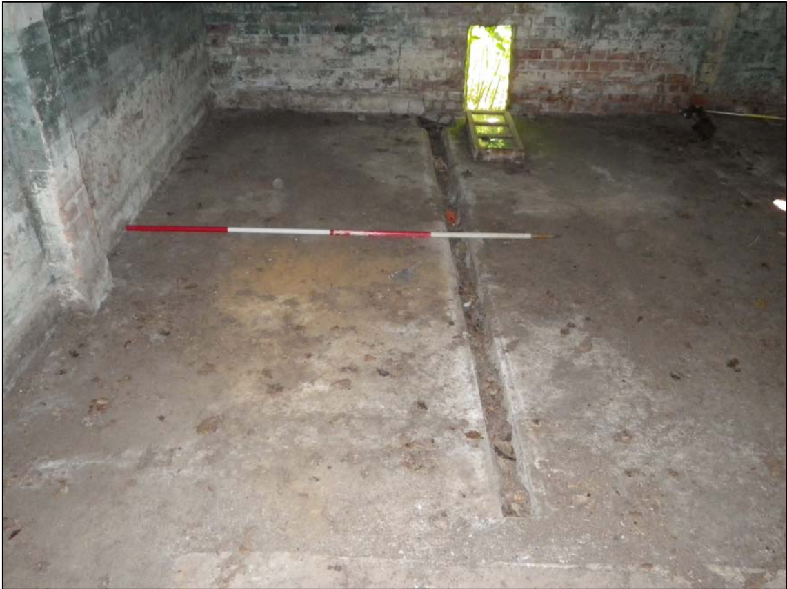
Plate 24. Building 1, Room 3, one of the two drains across the floor (ref. HTQ 68)
