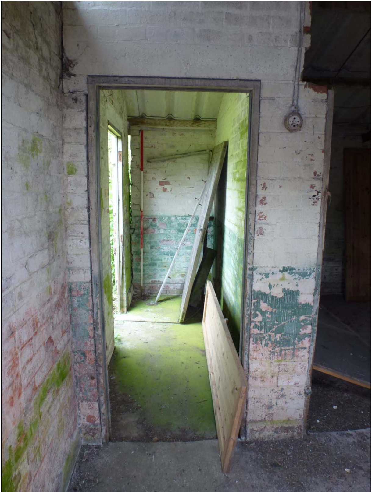
Plate 31. Building 2, Room 1, viewed through Door 4 (ref. HTR 21)
