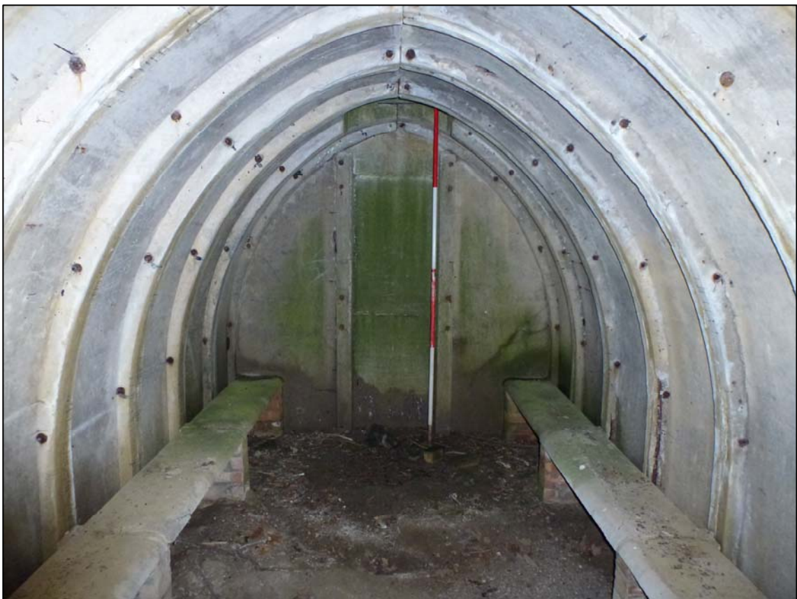
Plate 40. Shelter 1 internal view towards the rear wall, the entrance to the escape shaft is visible in the roof (ref. HTR 41)
