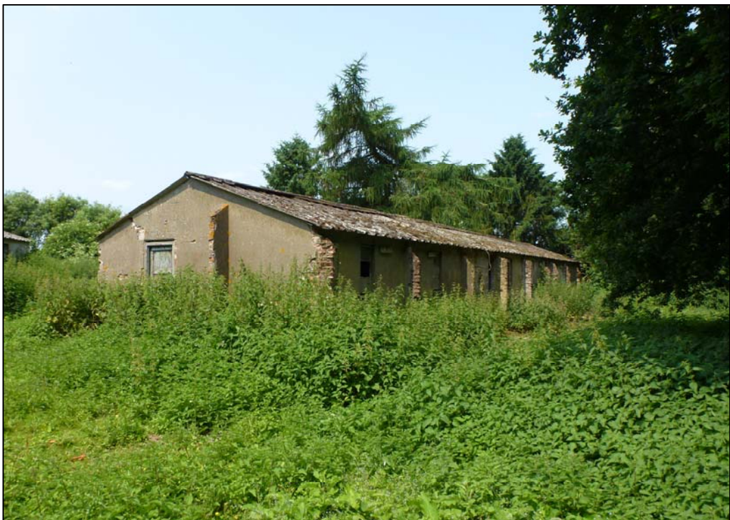
Plate 2. Building 1 -general view, camera facing north west (ref. HTQ 08)
