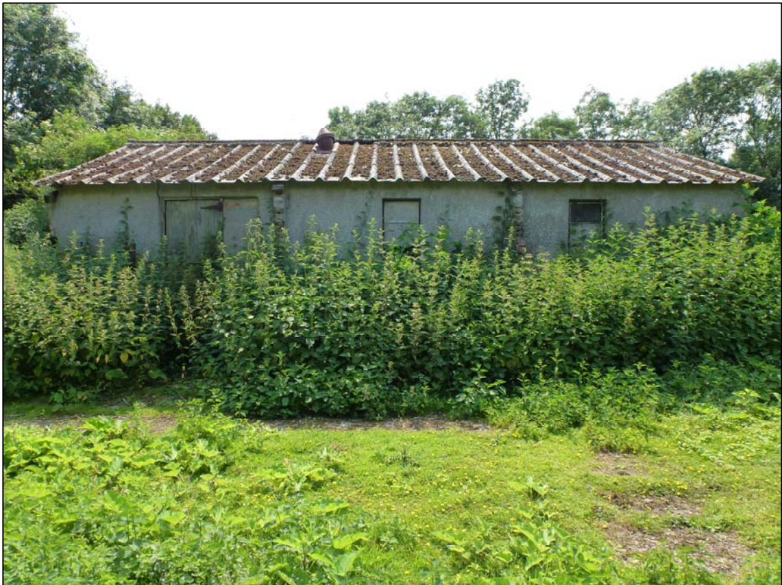
Plate 6. Building 2 -camera facing south west (ref. HTQ 38)
