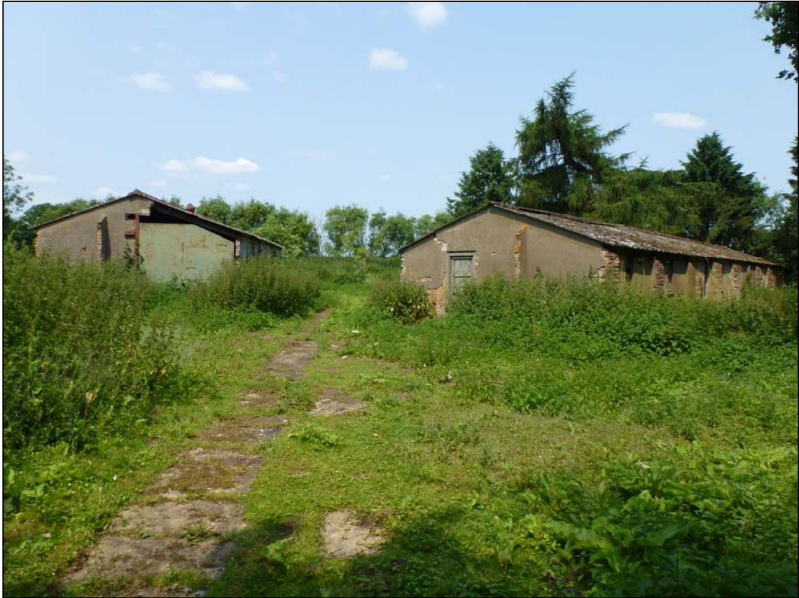
Plate 7. Building 1 (right) and Building 2 (left) -camera facing north west (ref. HTQ 09)
