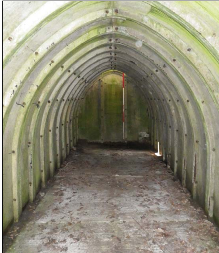
Plate 42. Shelter 3, internal view towards the rear wall (ref. HTR 60)
