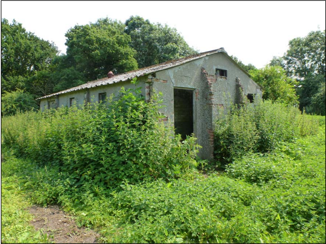
Plate 5. Building 2 -camera facing south (ref. HTQ 50)
