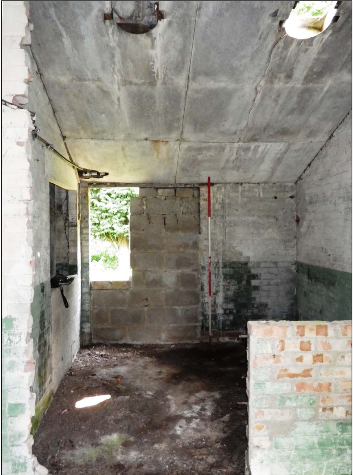
Plate 28. Building 1, view into Room 4 from Room 2 (ref. HTQ 76)
