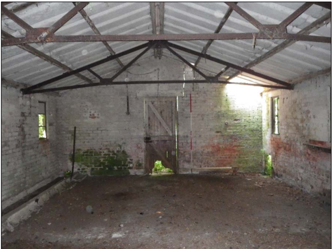
Plate 30. Building 1, Room 5, camera facing north (ref. HTQ 89)
