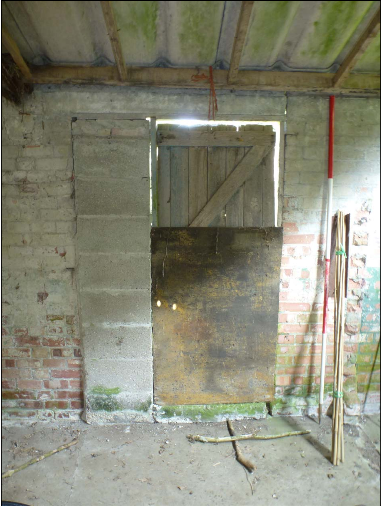
Plate 36. Building 2, Room 2c, Door 2 internal view (ref. HTR 25)
