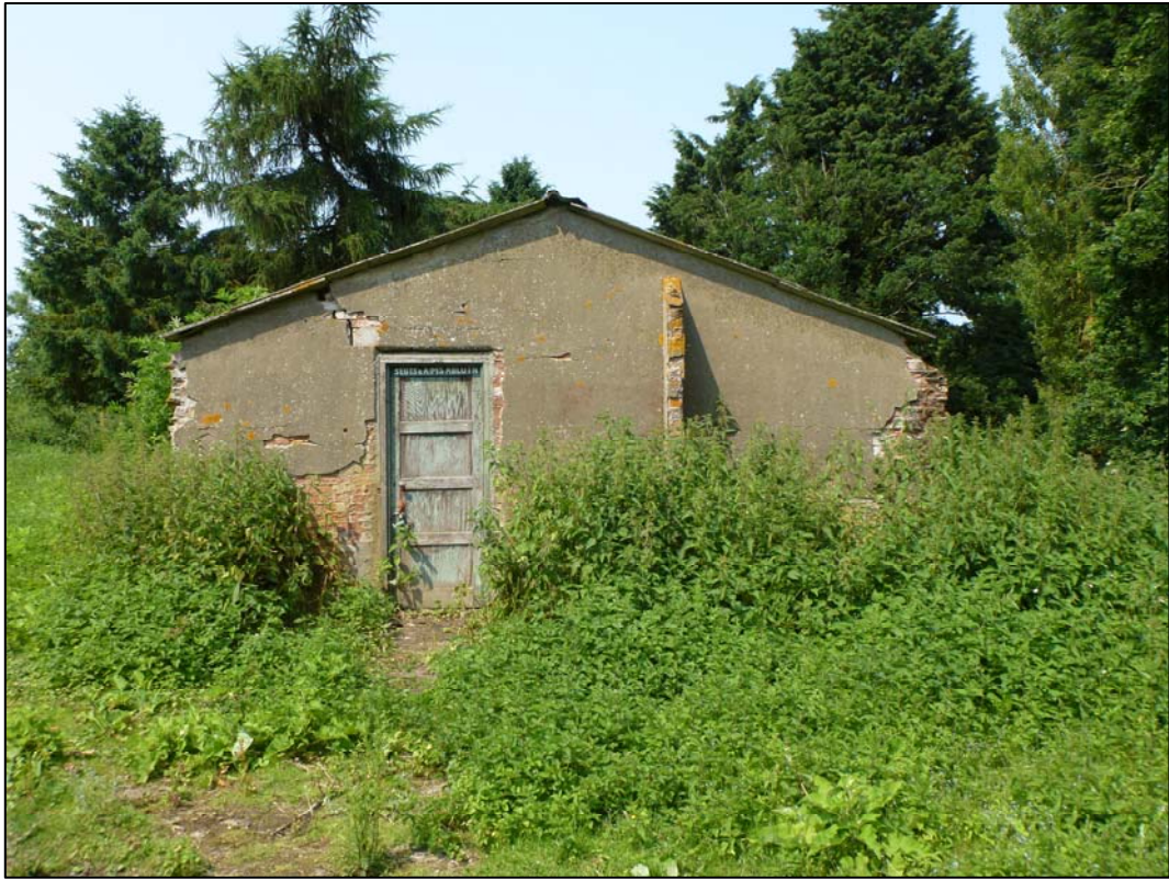
Plate 1. Building 1 -southern gable end wall (ref. HTQ 39)
