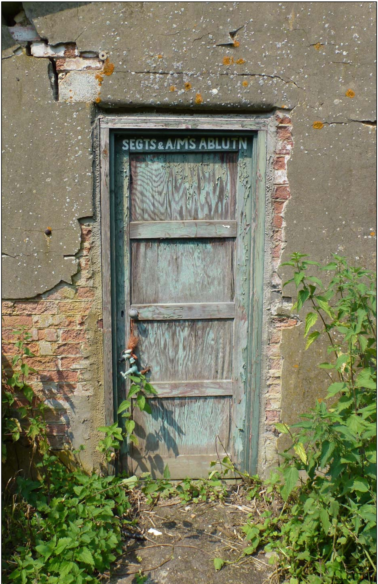
Plate 17. Building 1, Door 1 (ref. HTQ 45)
