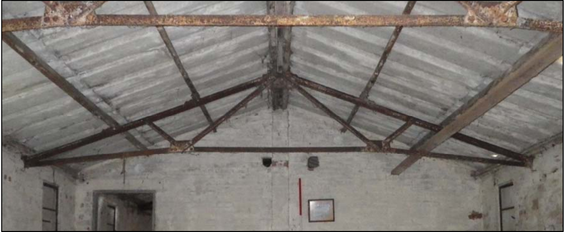
Plate 9. Typical roof truss, as seen in Building 1(ref. HTQ 65 [crop])
