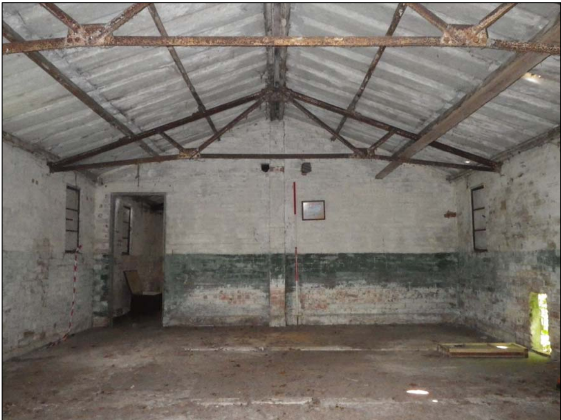
Plate 23. Building 1, Room 3, camera facing north (ref. HTQ 65)
