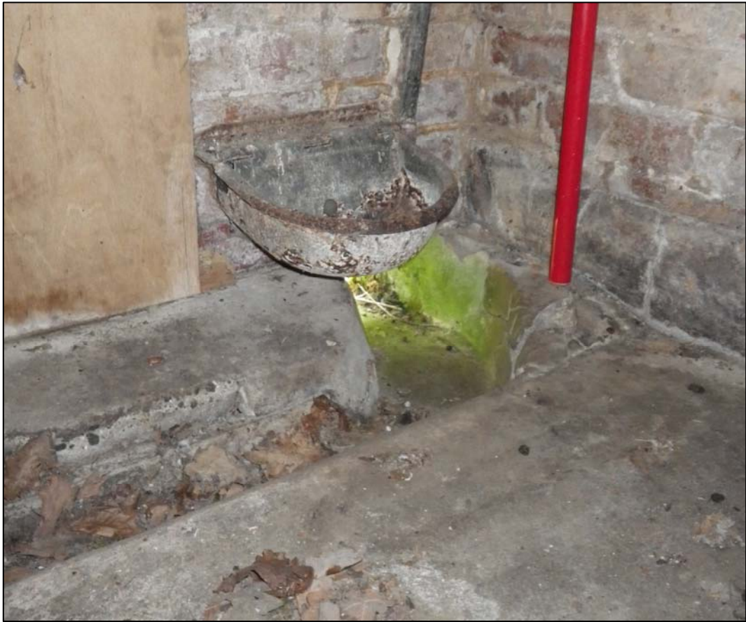
Plate 20. Building 1, Room 1, exit of eastern drain (ref. HTQ 80)
