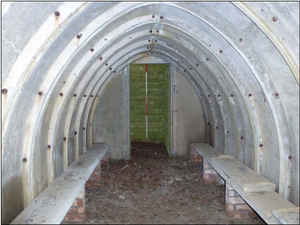
Plate 39. Shelter 1 internal view facing main entrance (ref. HTR 43)
