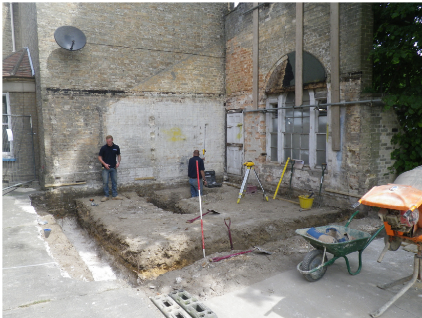
Plate 2. The development site with the foundation fully excavated. The soil profile within the trench nearest the camera shows a dark, clay-rich soil deposit over a thin charcoal spread relate to the century use/clearance of the site prior to the construction of Shrublands House in the 18th century .
