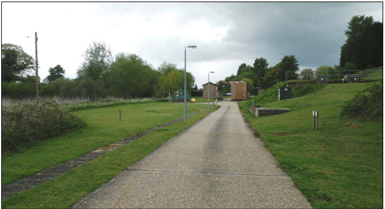
Plate 3. View north along main roadway showing the covered reservoir to the right and wild grassland away to the left
