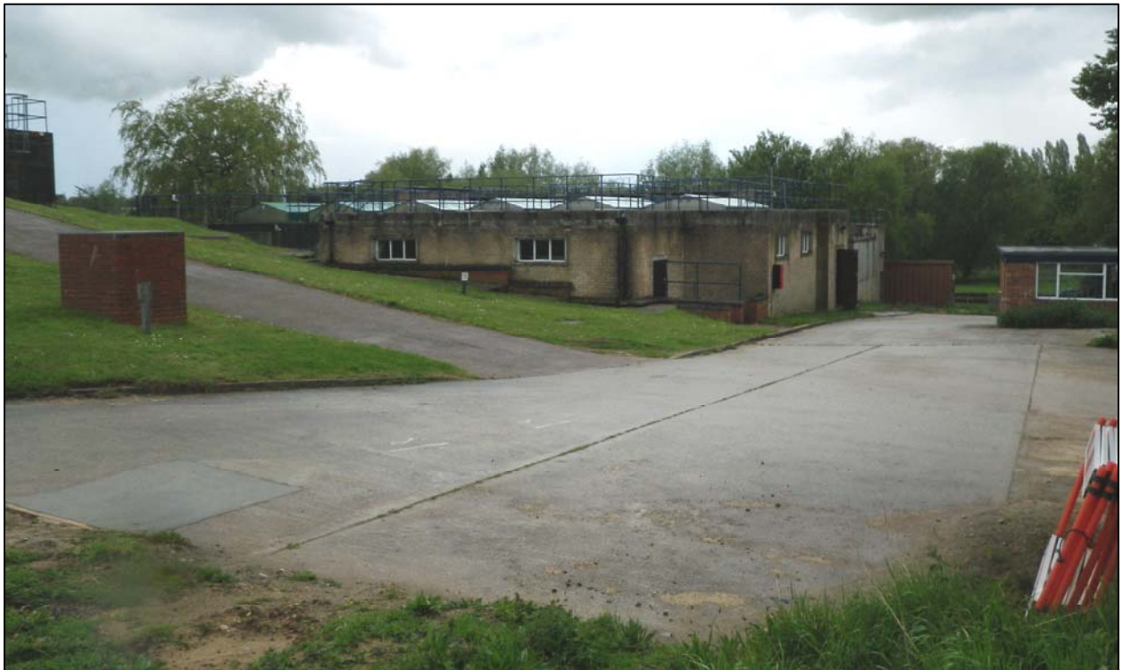
Plate 1. General view of the northern complex of buildings (camera facing south west)
