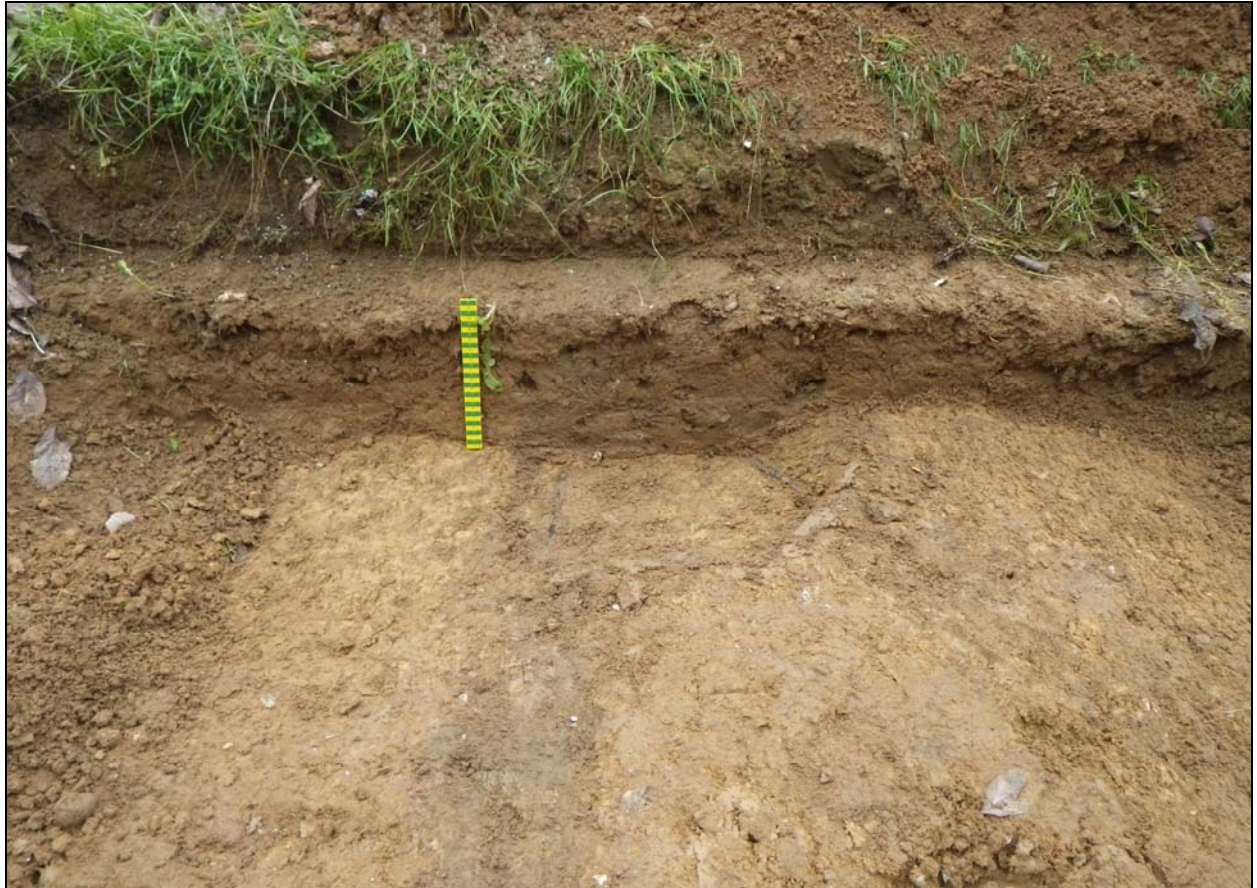
Plate 3. Trench 3 facing west and showing modern services and stepped section of trench (0.3m scale)
