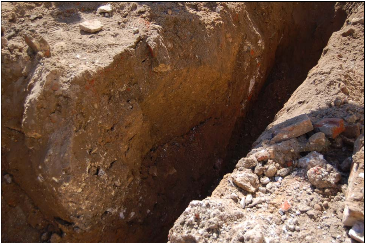
Plate 2. Section in footings showing lime-mortar(?)/CBM lined pit, facing southeast
