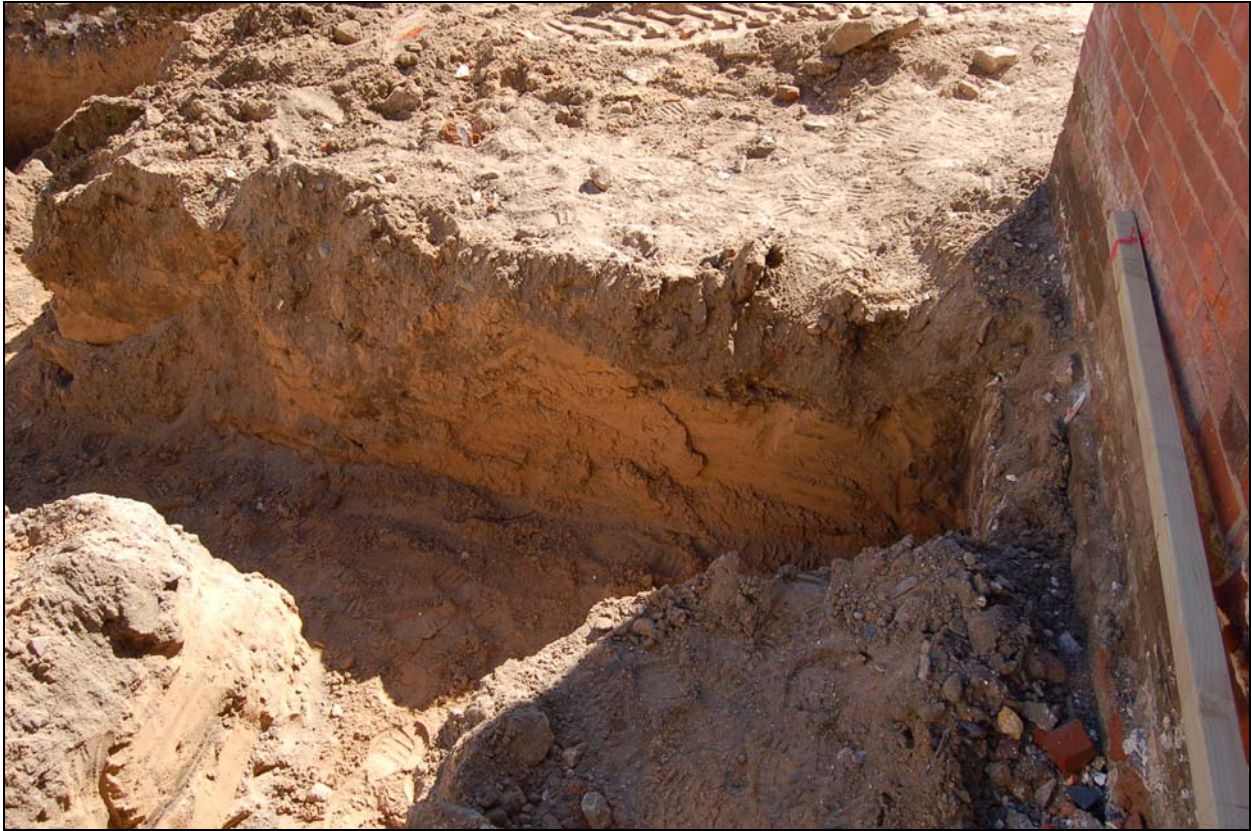
Plate 3. Section in footings showing undisturbed natural sands, facing east
