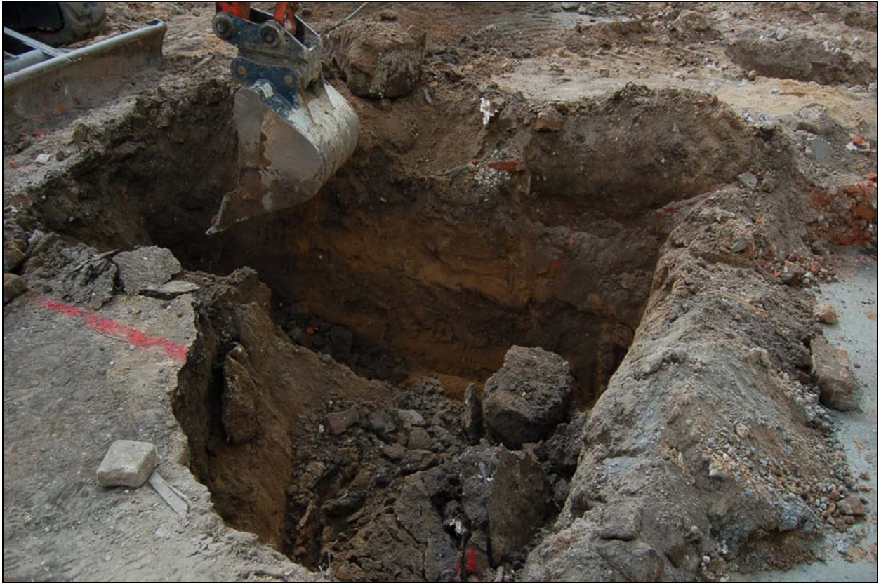
Plate 1. Section in footings showing layered stratigraphy as well as edge collapse, facing southeast
