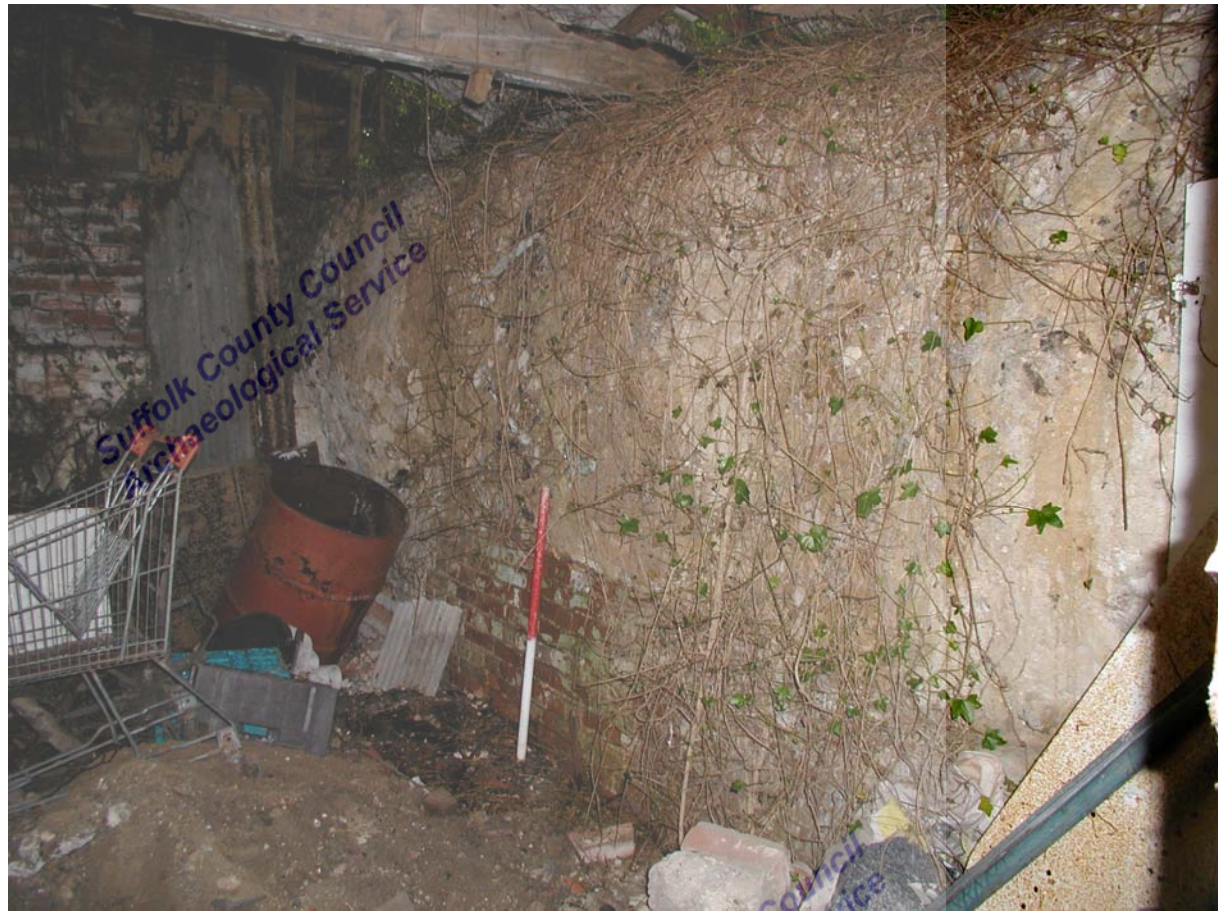
Wall Section 3, North Side, View A – A, Eastern End
