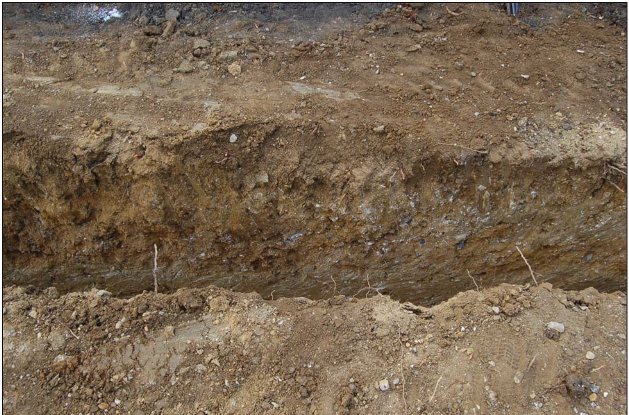
Plate 1. Footings on south side of house plot, facing south
