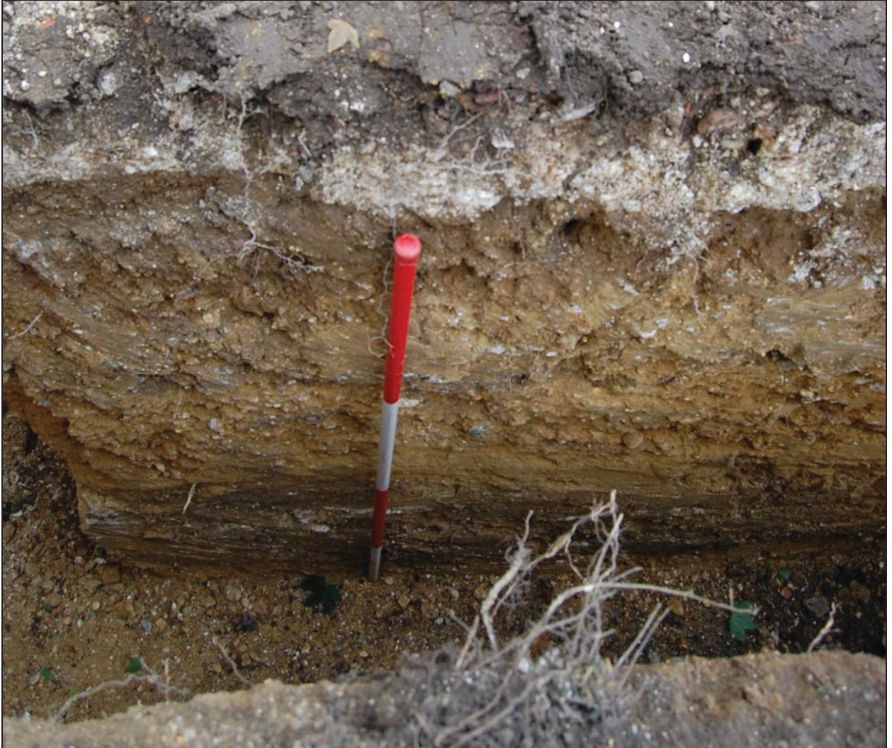
Plate 3. Footings of garage, facing south (2m scale)
